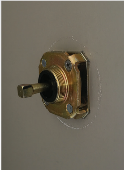
Figure 1. The 40H series lever return springs are located on the outside of the mortise lock case.
