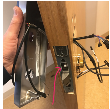
Figure 26. The author is feeding the wires through the hole, starting with the biggest.
