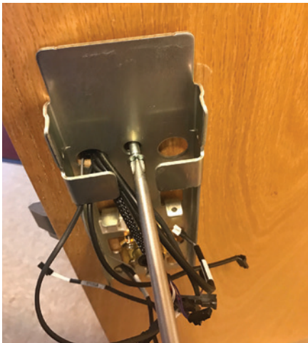
Figure 29. The wires have been passed through the door and backplate.
