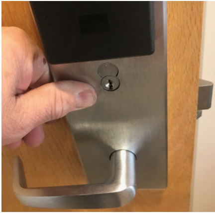
Figure 28. Take care that the cylinder isn't sticking out too much. If it does, there will be a gap between the door and the trim because the cylinder is pushing it out.
