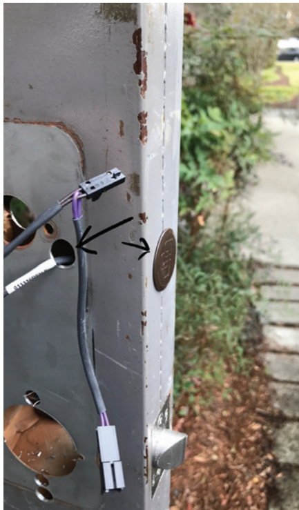
Figure 41. The author drilled a small hole on the inside only and ran the wire from the door sensor through it.
