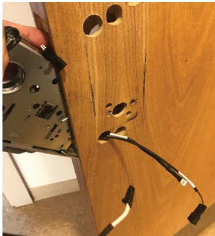
Figure 22. The author is about to pass the top wires through the “B” hole.
