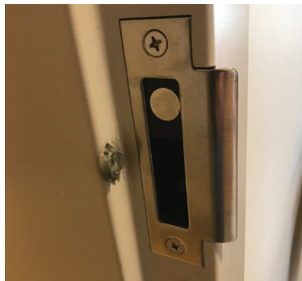
Figure 35. The author has installed the strike and box with the magnet at the top.
