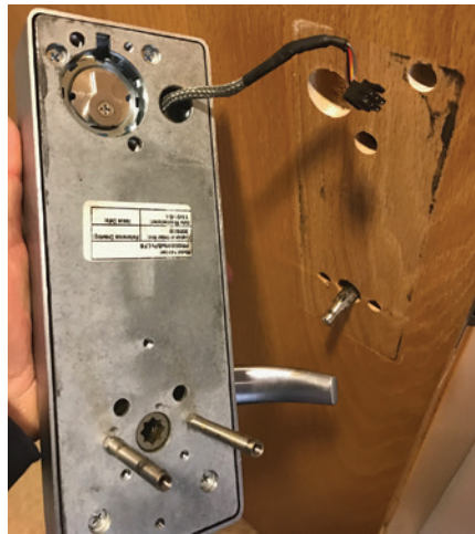
Figure 10. In this photo, the author is removing the outside trim.
