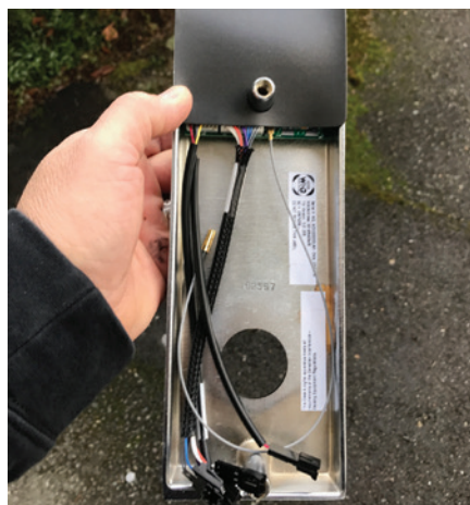
Figure 25. This photo shows an outside trim for a cylindrical lock, but it’s being used to show the wires that will feed through the “B” hole.
