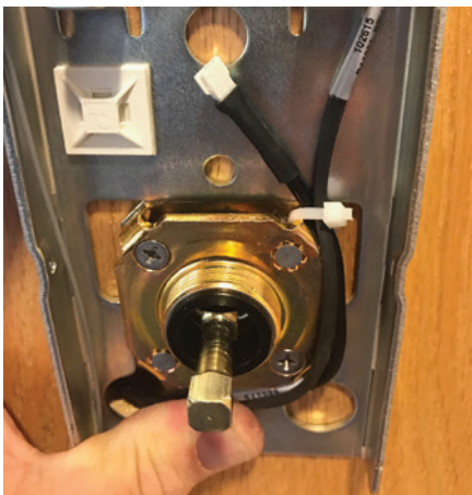
Figure 30. The author is wire-tying the bottom motor wire and RQE to the spring cage to keep it out of the way.
