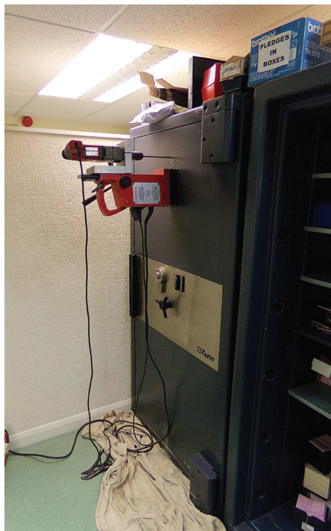
Figure 7. A hole was drilled in the same place as the bottom to see if there was difference in the distance the boltwork was traveling back, but there wasn't.
