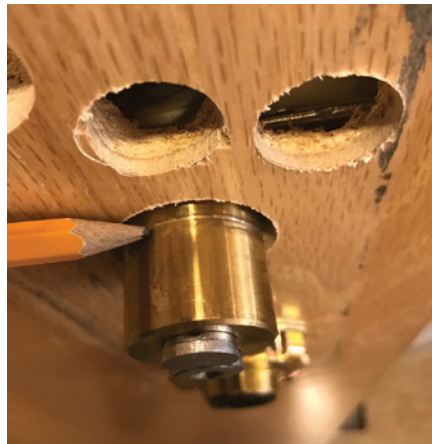
Figure 24. The spring cage is installed below the cylinder.
