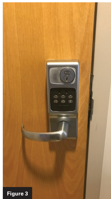
Figures 3-4. Figures 3 and 4 are the outside and inside trim of a Schlage combination mortise lock.
