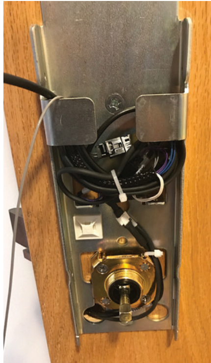
Figure 31. Once he connected the wires, the author wire-tied them in a bundle to keep them out of the way.
