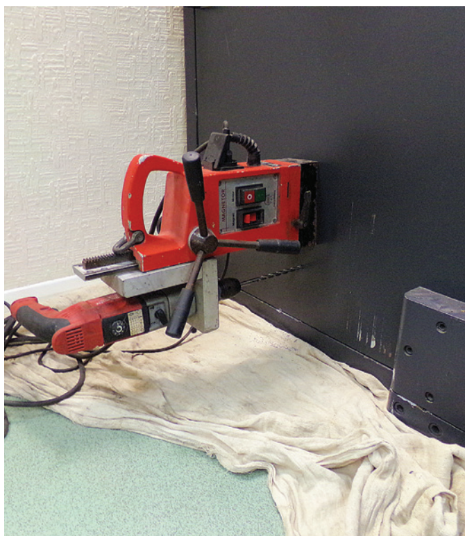
Figure 4. A hole was drilled in the bottom bolt area; drilling can be time-consuming in this area.
