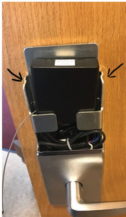
Figure 32. The bottom cover has been placed over the backplate and secured with two T-15 Torx security screws on the sides.
