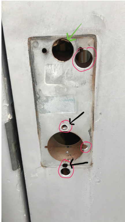
Figure 40. The prep is shown here. The pink circles are the new holes.
