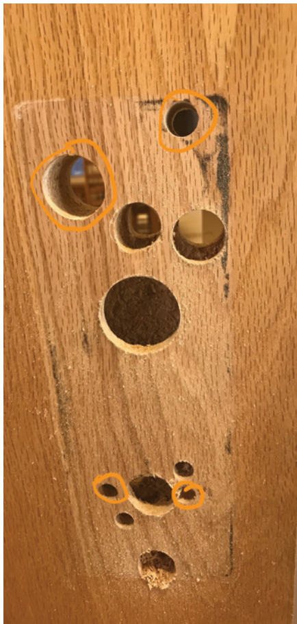
Figure 18. This photo shows the completed prep on the outside of the door.
