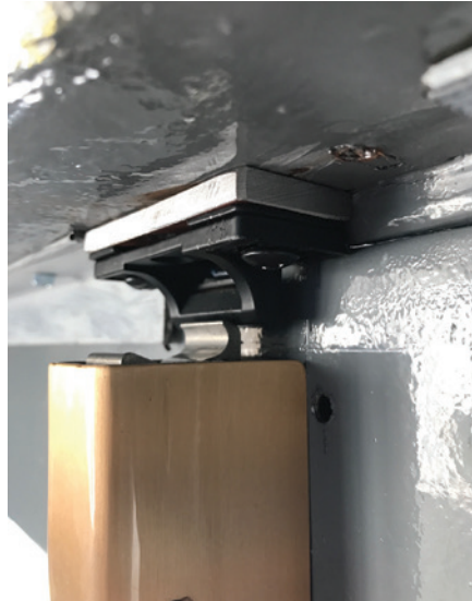
Figure 19. This photo shows the almost-finished strike and shim.
