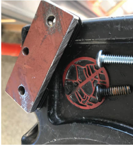
Figure 18. The contractor had some large pieces of angle iron that were close to the right thickness and cut them to size for the author to use as shims. All he had to do was drill through holes.
