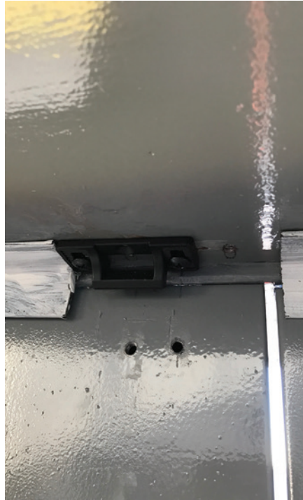
Figure 5. The contractor installed the angle stock to act as a temporary stop molding, allowing the author to correct the issues with the installation.
