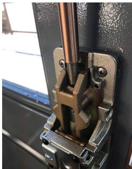
Figure 11. Here, the author is screwing the top rod back onto the head of the bar.
