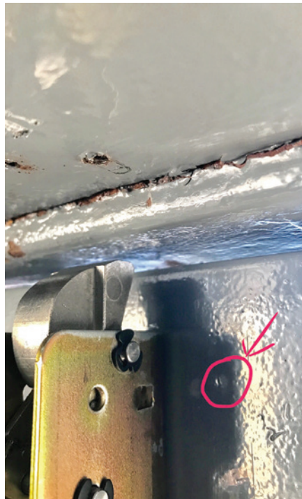
Figure 7. The latch is installed. Compare Figure 7 with Figure 4 to see the difference in height. The pink arrow points to an unused extra hole.
