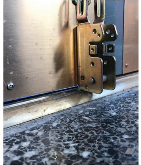
Figure 20. This image shows the bottom bolt improperly installed too low on the door.
