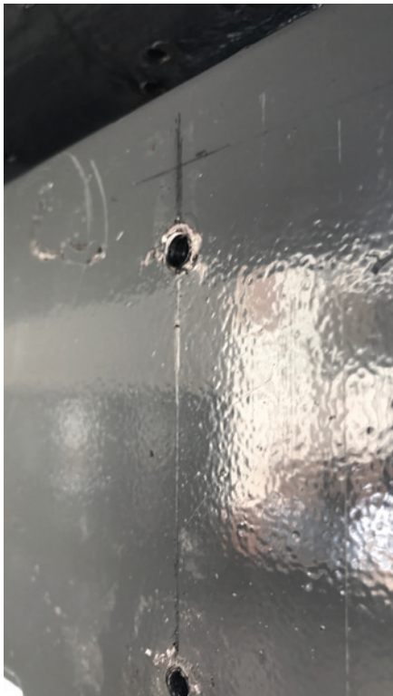
Figure 6. The penciled cross marks the centerline and the top of the top latch bracket.
