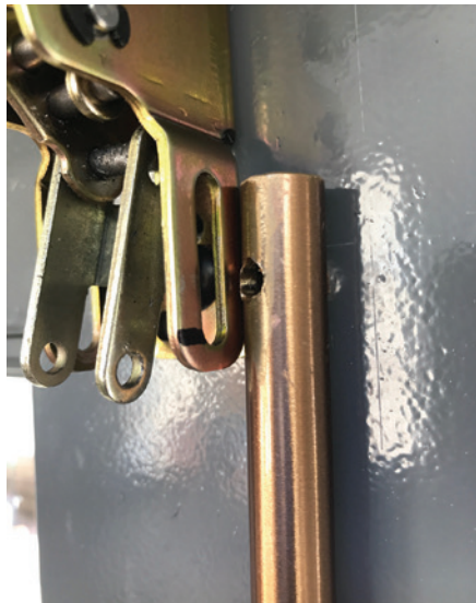
Figure 8. The top of the rod extends too far into the latch mechanism.
