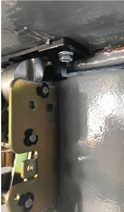
Figure 4. The bracket holding the top latch is placed too close to the top of the door to compensate for the lack of stop.
