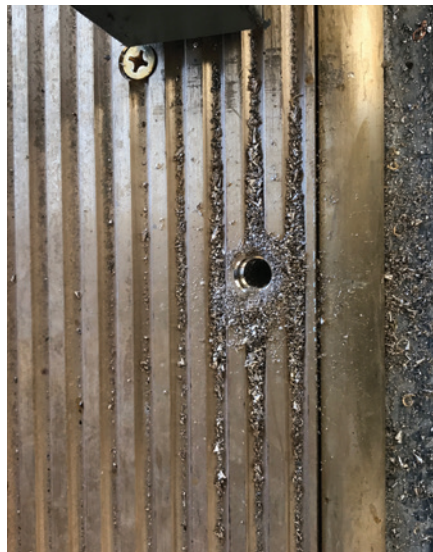
Figure 21. This photo depicts the drilled strike hole.
