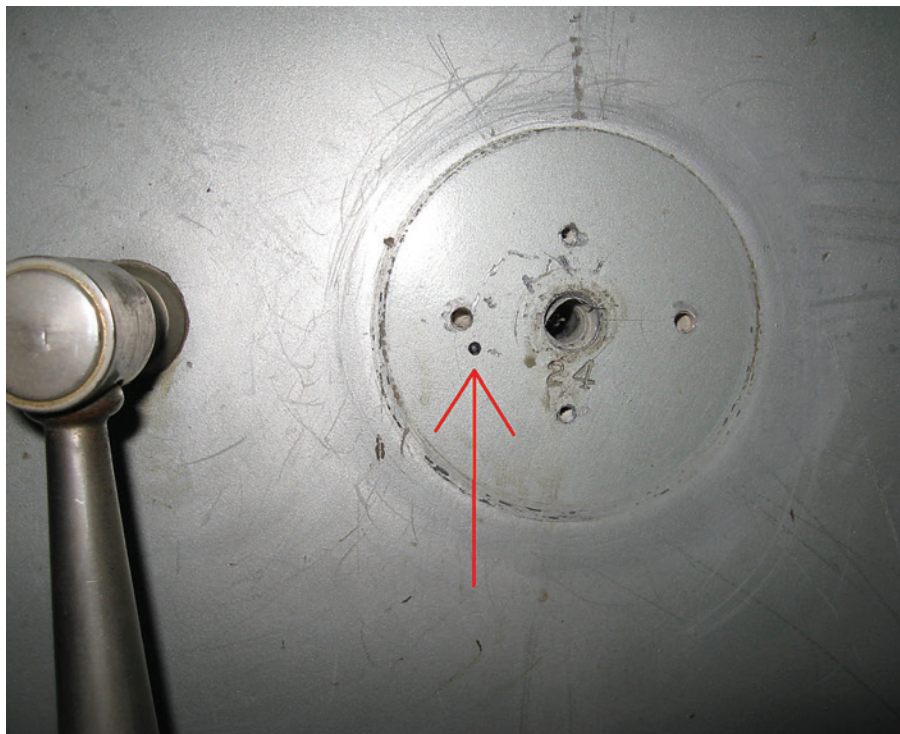
Figure 7. Using the template as a guide, the decision was made on where to put the hole in the door.
