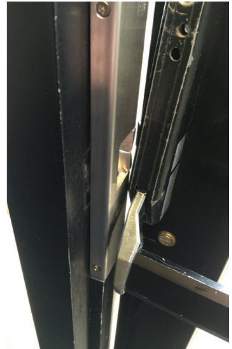
Figure 1. A panic device is hitting a recently installed electric strike and preventing the door from closing. The original technician should have determined that, at the very least, a sagging door due to worn pivots caused unacceptable clearances between both pieces of hardware, and this situation would eventually occur.
