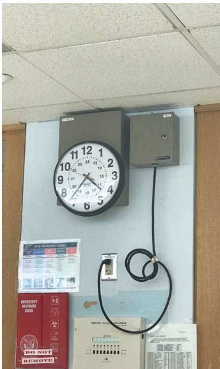
Figure 29. When the original system was installed years ago, an electrician was supposed to come back and hard-wire the power supply. You can see how that worked out.
