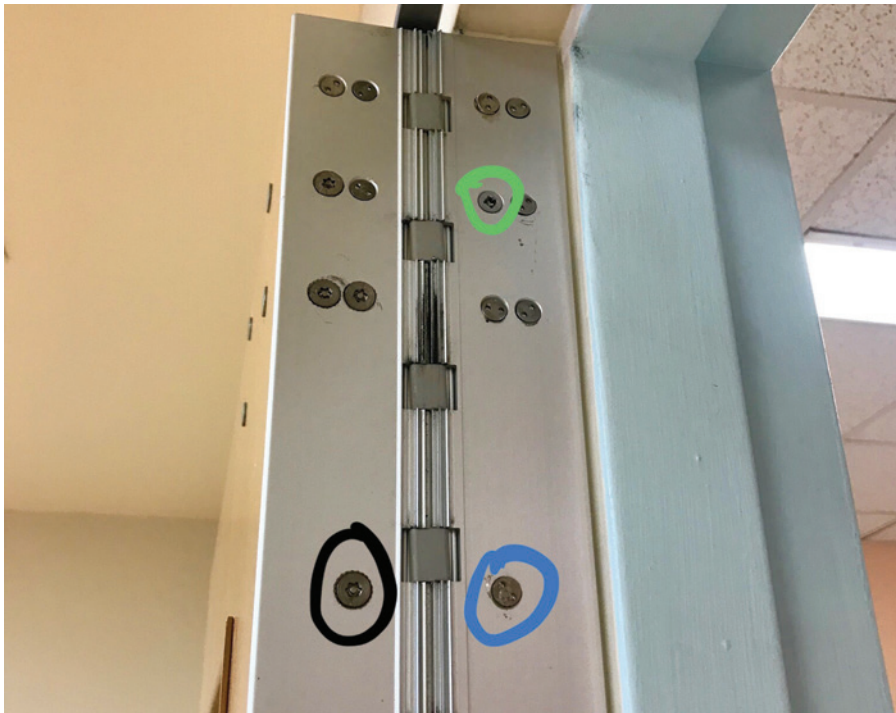
Figure 6. This image is a view of the existing full mortise continuous hinge. Take note of the mish-mash of different screws: black is a high-security torx, blue is a "snake eyes" spanner screw and green is a stripped #3 Phillips.
