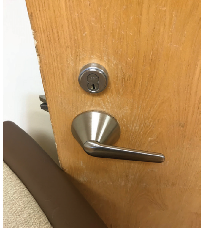
Figure 5. This photo shows the anti-ligature mortise lock made by Securitech.
