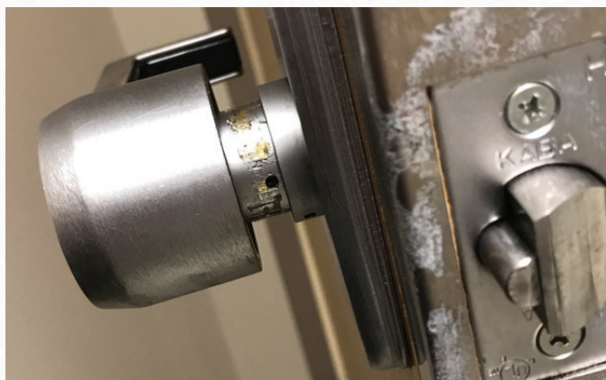
Figure 18. After rotating the ring with the pliers, it was apparent that the retainer access hole was back where it was supposed to be to access the retainer and remove the lever handle.
