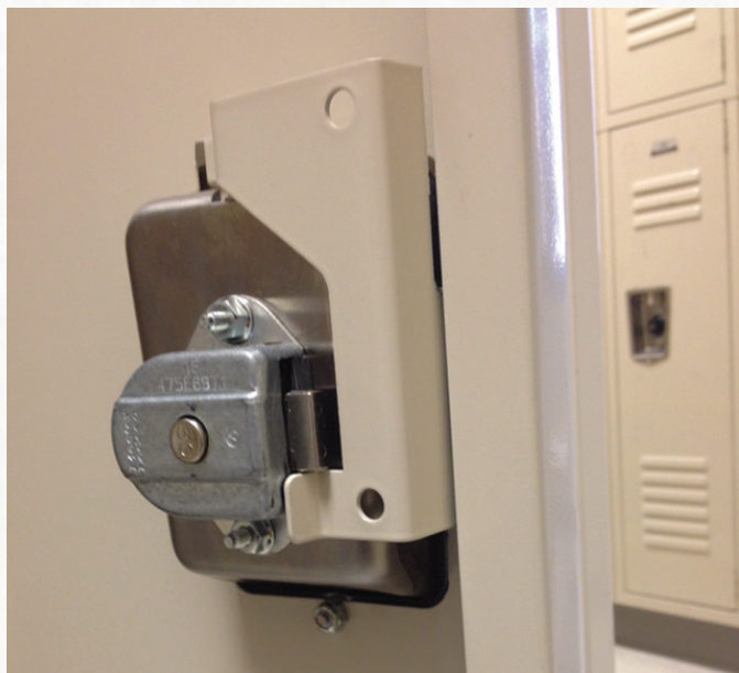
Figure 4. This photo gives an inside view of the locker door shows the mechanism that lifts when the lift handle on the outside is engaged. With the different locker styles, we used basically three types of Master combination locker locks. They are typically available in left and right hand versions of a particular style lock. This is a lift bolt style. When the correct combination is dialed, the outside lift handle is moved upward, which causes the mechanism to physically lift the bolt, allowing the locker door to open.
