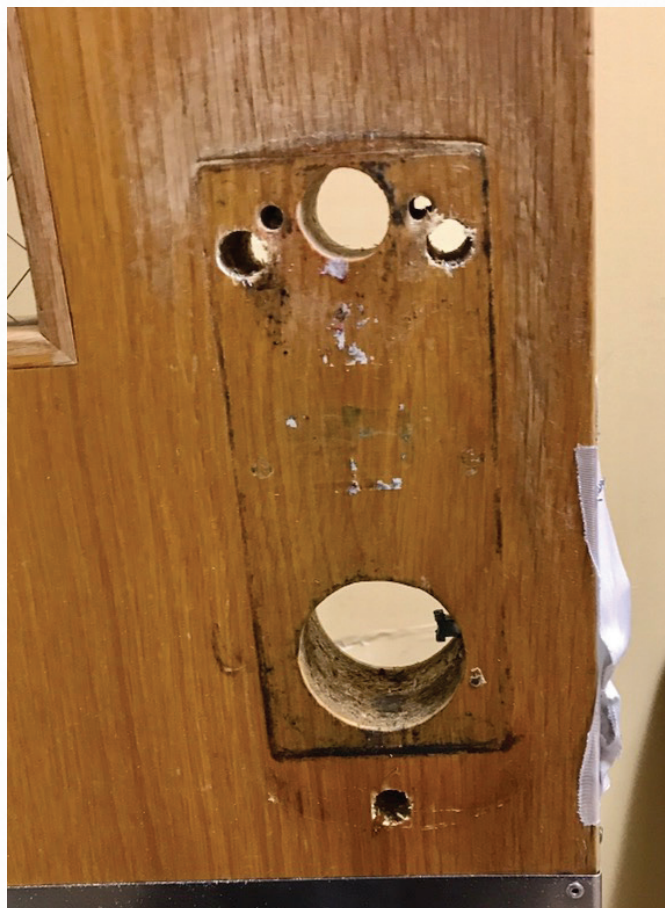
Figure 25. The lock is drilled off the door, and the previous mounting holes are exposed to view. A job can be made more difficult if someone unqualified tries to do the job first or if it doesn't get assigned to the right person in a reasonable amount of time before the situation degrades.
