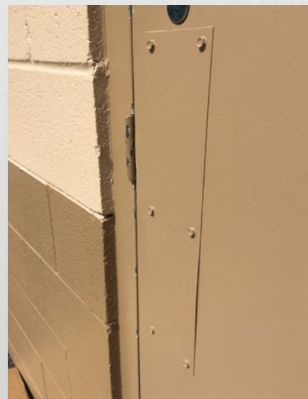
Figure 1. A push plate is covering a 161 prep on a door. The previous locksmith installed a panic device with no exit trim.
