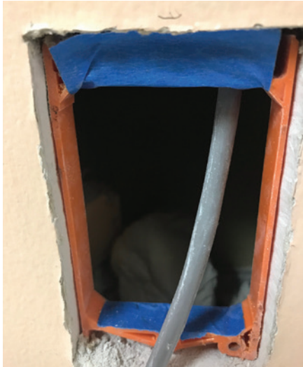
Figure 14. The author removed the plastic “wings” on the ring and reversed it. Tape is holding it in place while the adhesive dries.
