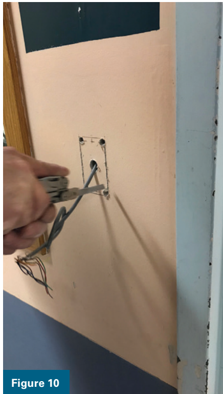
Figures 10-11. In Figure 10 , the author and his partner are cutting out the opening for the key switch, and Figure 11 shows the finished cutout.
