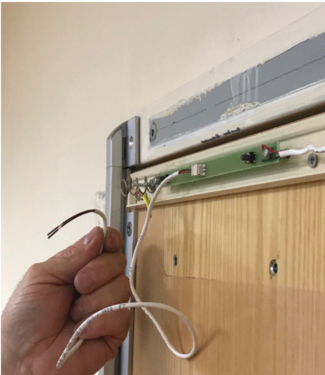
Figure 22. Under the spring with the yellow tape on the end of the wire is the cable that will connect to the hinge wire.
