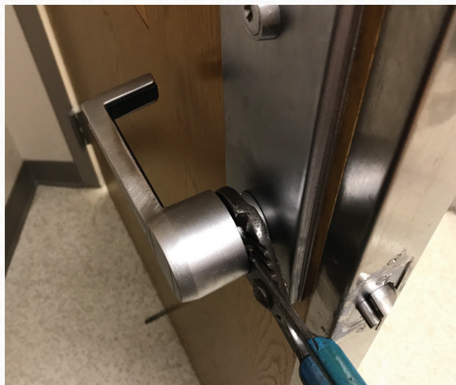
Figure 17. To compensate for what the earlier person did wrong, I had to take a pair of pliers to rotate the ring again so the retainer hole returned to its correct position about 3 o'clock.
