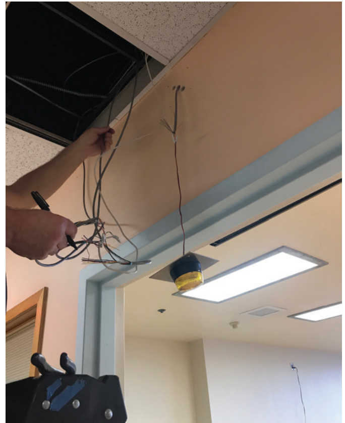
Figure 9. The author's partner is wiring the strobe to the wire the electrician ran.
