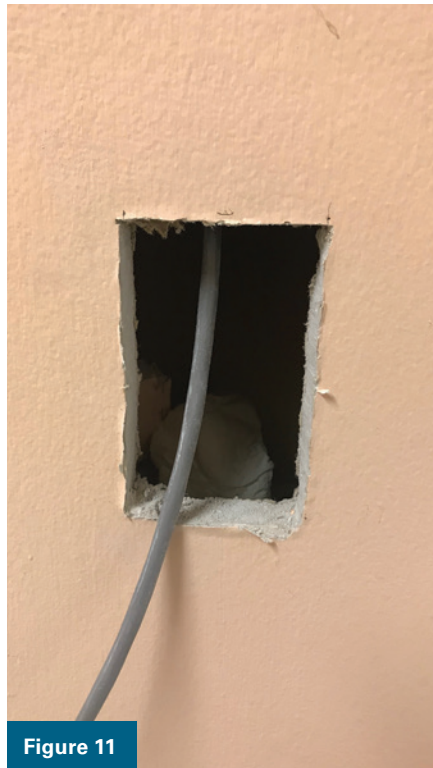
Figures 10-11. In Figure 10 , the author and his partner are cutting out the opening for the key switch, and Figure 11 shows the finished cutout.
