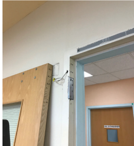
Figure 15. The author pulled the wire down through the hole after removing the door, marking the frame and drilling for the wire that connects the bar to the control box.
