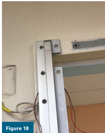
Figures 17-18. These photos show the position of the wires as they pass through the hinge and how the hinge will look on the frame once it’s installed.
