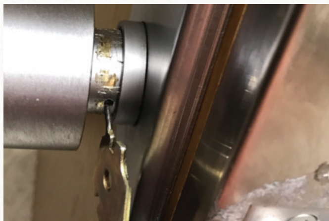
Figure 19. A poke tool is lined up with the access hole to attempt removal of the handle.
