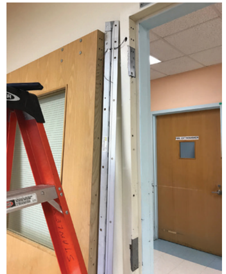
Figure 19. This image shows the wires connected and the splice inside the frame
