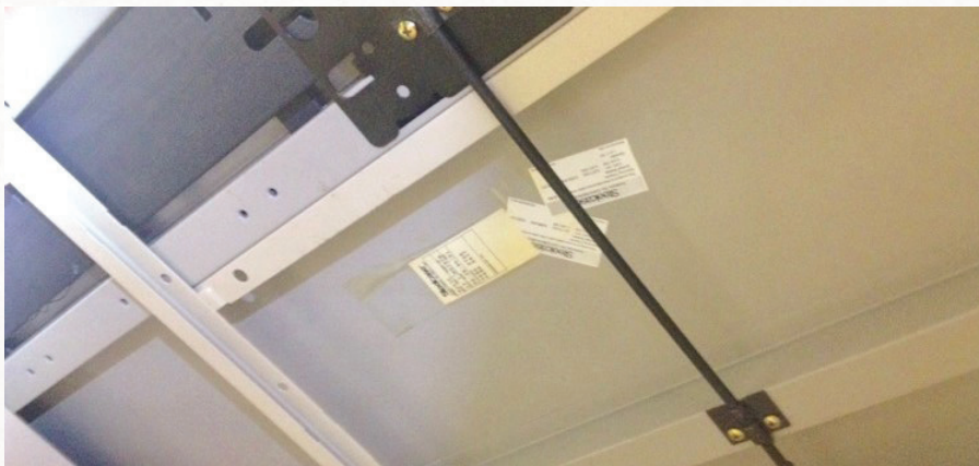
Figure 10. Here is another view of the parts that lock the center drawer. Office furniture repair has become a secondary skill to me. I never really repaired office furniture as a commercial locksmith. Heck, they wouldn't even want to pay me to fit a key, let alone actually repair the mechanism itself.
