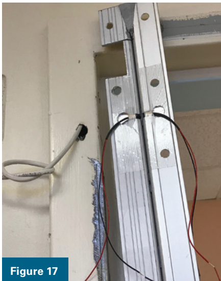
Figures 17-18. These photos show the position of the wires as they pass through the hinge and how the hinge will look on the frame once it’s installed.
