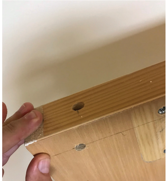
Figure 21. This photo shows the hole we drilled on the top of the door to join the other two holes to create a path from one to the other.
