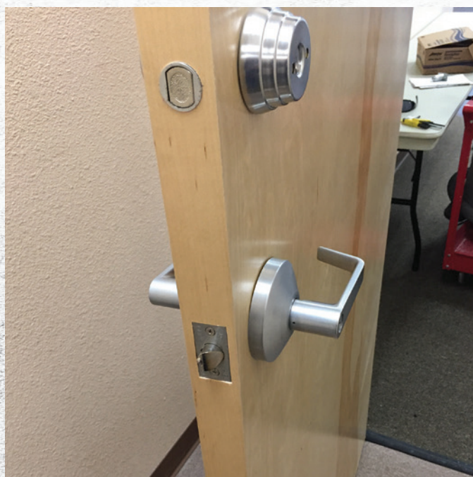
Figure 1. This photo shows the existing door with a standard lever lock. Notice the distance to deadbolt above the lock. There was not enough room for a taller push-button lock, and because this was between two office areas with separate exits, the customer wanted to keep the double-cylinder deadbolt. I could have moved the deadbolt up, but why do so when I could try out the Revolution?
