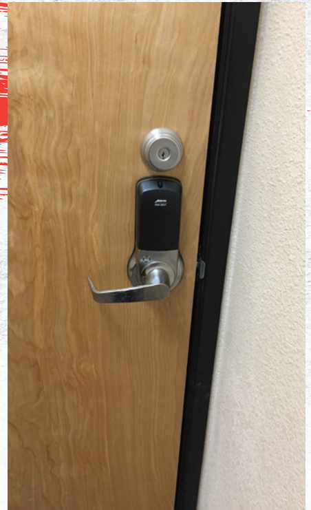
Figure 9. In the completed lock shown here, the housing or lock just fit under the deadbolt.
