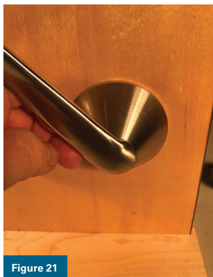
Figures 20 and 21. In Figure 20 , the author is holding the lever on with his thumb; notice the lever is tilted down. I would normally immediately move to Figure 21 , which causes the lever to rotate a little so the screw moves behind the step in the cutout.
