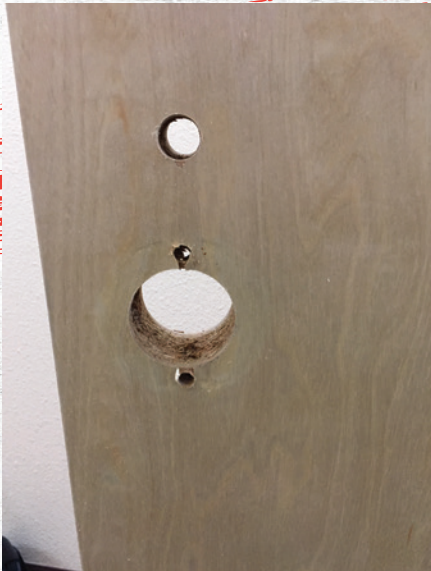
Figure 2. The only additional hole added was for the cable and upper thru-bolt. The original lock used the fairly common \frac{5}{16} " hole thru-bolt spacing of 2\frac{3}{4} " apart.
