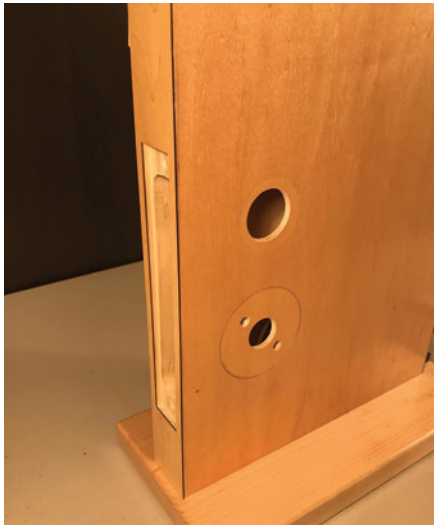
Figure 8. The prep for this lock is a typical mortise prep and is similar to, if not the same as, a Best 45H.
