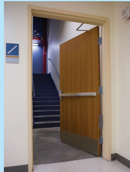
Figure 7. The stairwell re-entry requirements vary between the IBC and NFPA 101; the IBC requires all stair doors to allow re-entry, with the exception of the discharge door.
