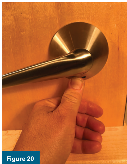
Figures 20 and 21. In Figure 20 , the author is holding the lever on with his thumb; notice the lever is tilted down. I would normally immediately move to Figure 21 , which causes the lever to rotate a little so the screw moves behind the step in the cutout.
