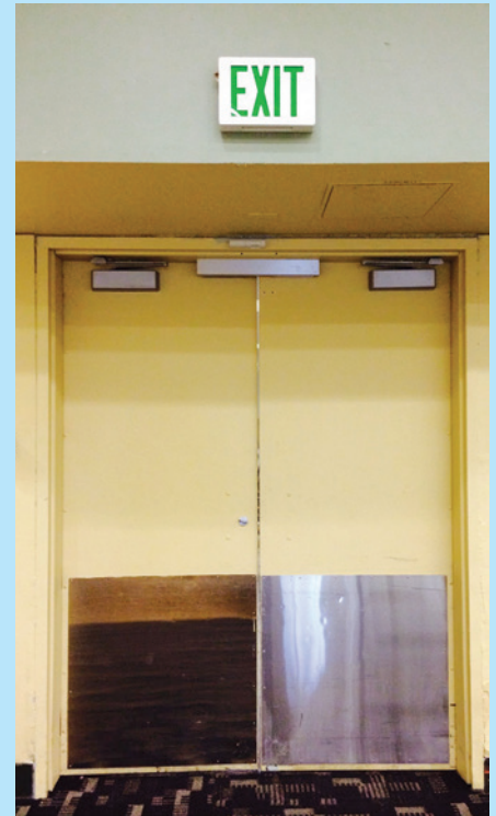
Figure 4. The section called “Access Controlled Egress Doors” was changed to “Sensor Release of Electrically Locked Egress Doors” in the 2015 IBC.
