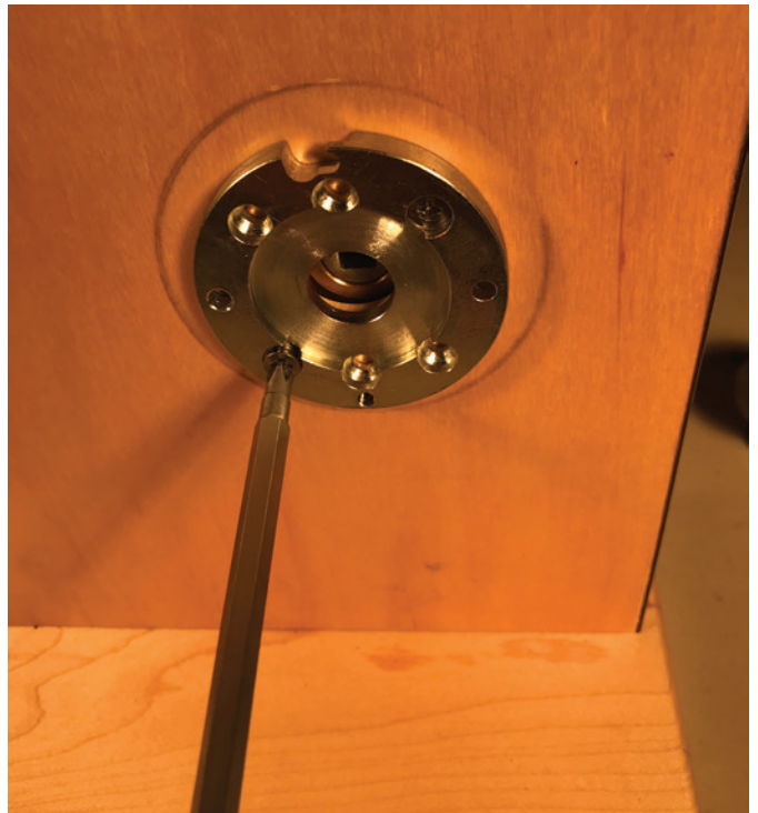
Figure 17. The author is screwing the backplate into the studs on the outside lever.
