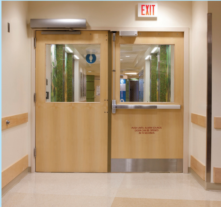
Figure 2. In the 2015 edition of the IBC, the activation time for delayed egress locks was changed from one second to three seconds, which is consistent with NFPA 101.
