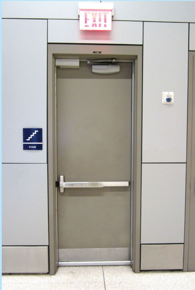
Figure 5. Mag-locks released by hardware mounted on the door are addressed in a separate code section from mag-locks released by a sensor.
