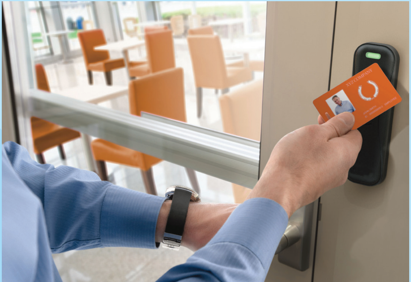
Figure 1. When a door equipped with an access control reader allows free egress using normal operation of the hardware, it is not typically considered one of the special locking arrangements.
