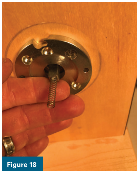
Figures 18 and 19. The author is inserting the spring-loaded spindle and then fitting the inside lever over the backplate.
