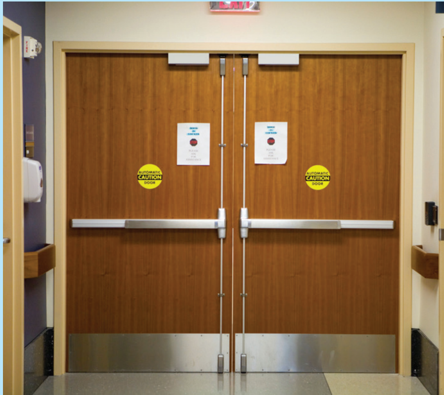
Figure 3. Controlled egress locks are allowed in some healthcare units, but staff must be prepared to facilitate egress if needed.
