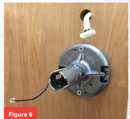
Figures 5 and 6. The solenoid cable needs to be routed through the spring cage assembly when mounting it to the lock.
