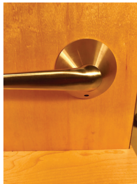
Figure 22. The inside lever is in its finished position with the lever horizontal.
