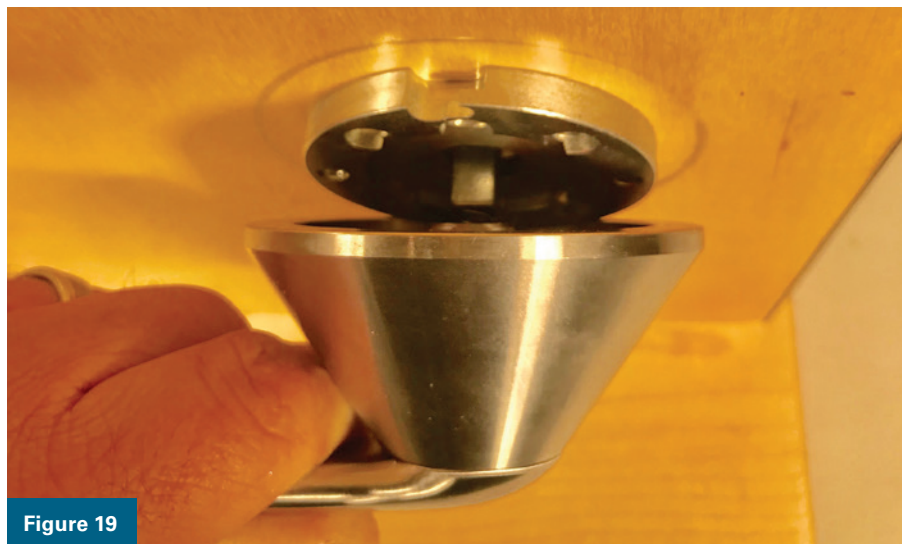
Figures 18 and 19. The author is inserting the spring-loaded spindle and then fitting the inside lever over the backplate.
