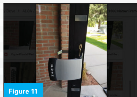
Figures 10-11. If the customer wants the lock to lock every time after the door closes, the Alarm Lock DL 1200 lock (Figure 10) is a good choice. The Adams Rite dead 4900 latch (Figure 11) will work well with this unit.
