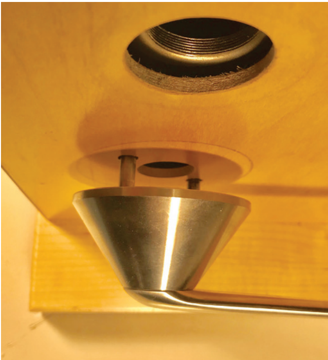
Figure 16. The author is fitting the outside lever studs through the door and lock. Notice that you don't see a spindle.
