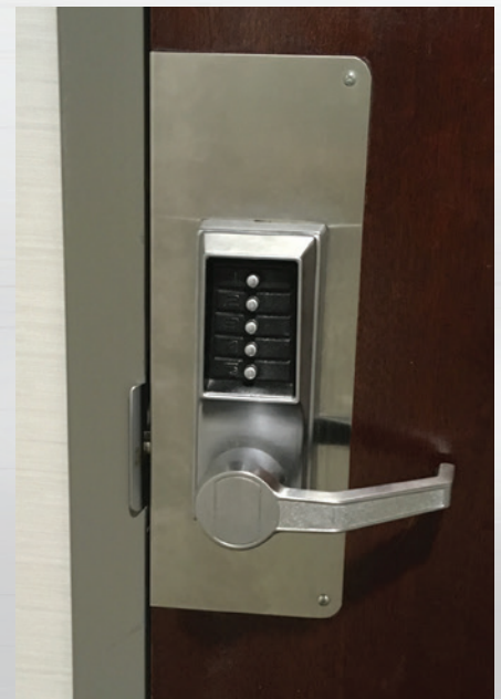
Figure 3. Don-Jo makes a wrap-around for the L1000 series to fit various existing preps.
