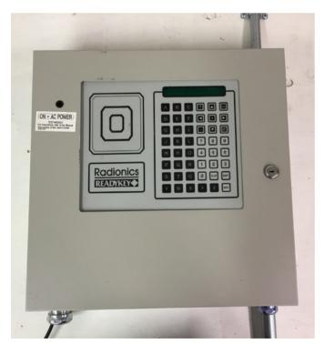
Figure 4. Radionics Readykey was purchased by Bosch a number of years ago. It's an older control panel that was produced by Stanley Pac, and they made two vintages in both two- and fourdoor models. The front keypad panel is used for initial programming, or it can be used to administer the system on the master or first controller in the system. Once the system is online with a computer or for all the additional panels on the system, the front panel is not needed.
