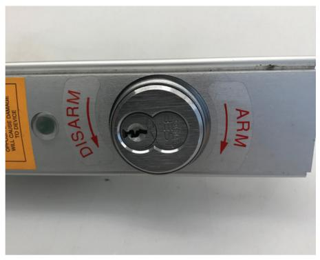
Figure 11. This photo shows the front of the cylinder and core.
