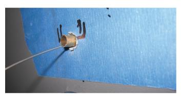
**Figure 9.** A piece of brass tubing a little longer than the thickness of the door was inserted into my <sup>5</sup>/<sub>16</sub>-inch hole.
