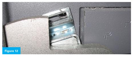
Figures 11 and 12. It took several tries to get the wire in front of the relocker, through the slot, and turned so that it was hooked.
