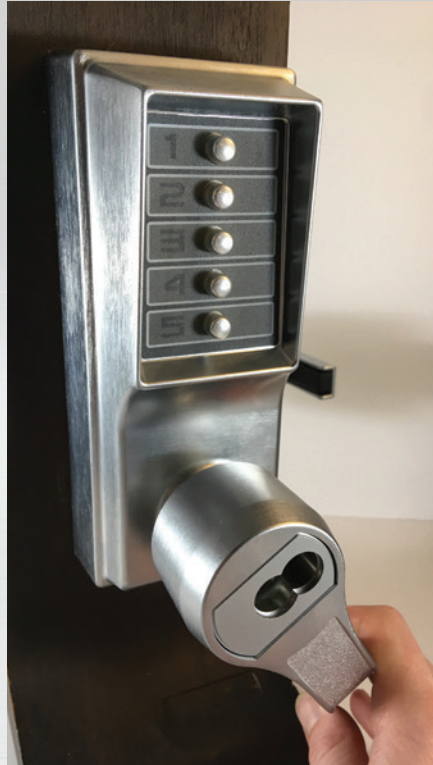
Figure 6. Turn the outside lever fully. The latch should not retract.
