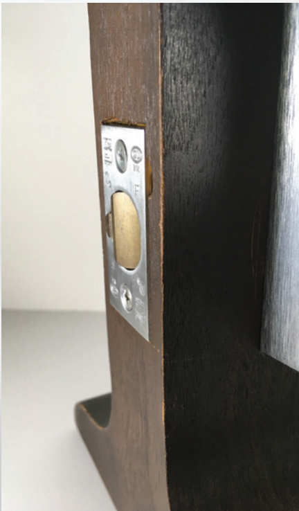
Figure 8. Turn the outside lever fully. The latch should retract. After ensuring the latch retracts, release the outside lever.
