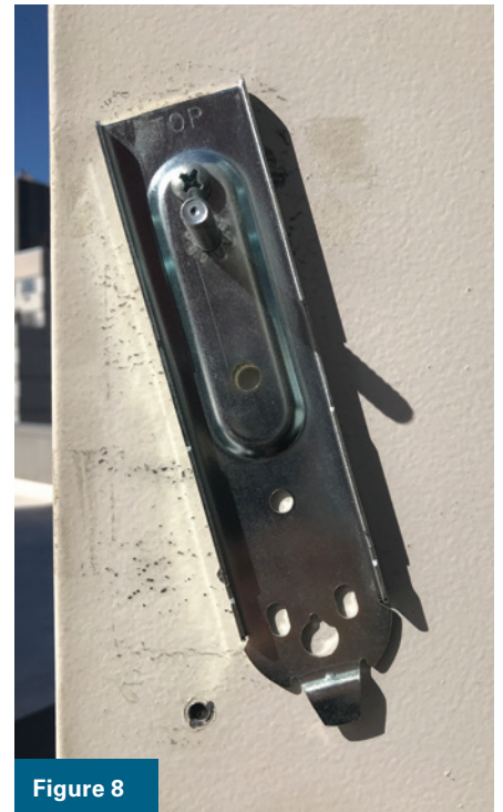
Figures 7 and 8. With the back plate set where it's supposed to be in Figure 7 , there's not another screw hole drilled into the door. Figure 8 shows how the plate can move and possibly trigger the alarm. The hole you do see doesn't line up with anything.
