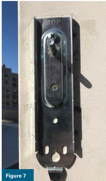
Figures 7 and 8. With the back plate set where it's supposed to be in Figure 7 , there's not another screw hole drilled into the door. Figure 8 shows how the plate can move and possibly trigger the alarm. The hole you do see doesn't line up with anything.
