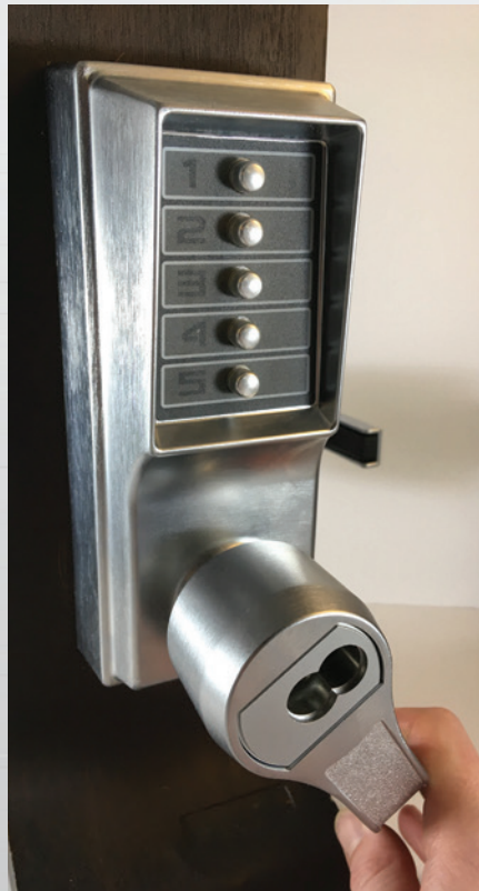
Figure 3. Turn the outside lever fully and release. The latch should not retract.
