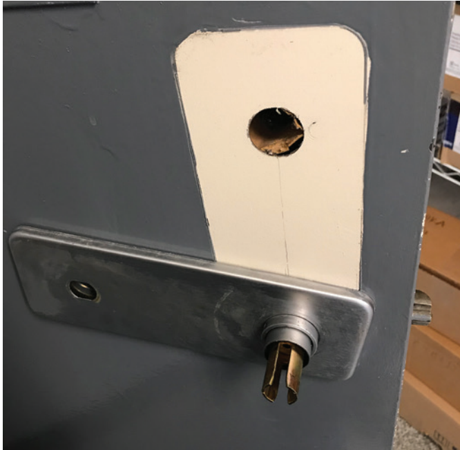
Figure 9. On this Simplex Unican lock, the outside trim of the lock looked crooked when the author encountered it. When he unscrewed the lock to reach the combination change sleeve, there was only one hole in the door aside from the 2½" hole for the chassis.
