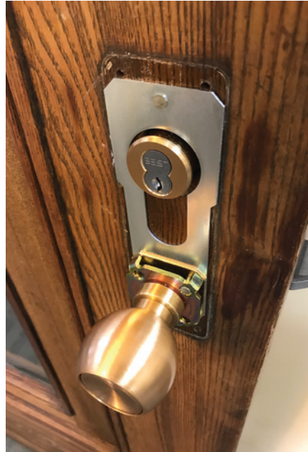
Figure 4. The author was forced to leave off the outside escutcheon to screw in the cylinder.
