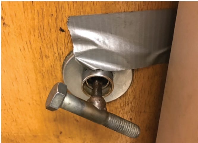
Figure 22. This image shows an innovative way someone replaced a broken lever using a welder.
