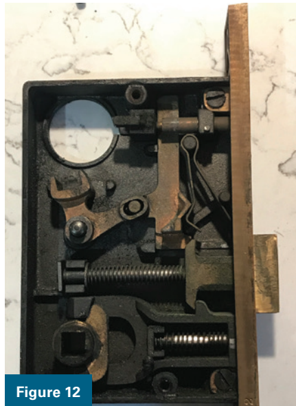
Figures 9-12. Figures 9-11 give the front, back and side views of the lock, and Figure 12 is the view of the internal parts.
