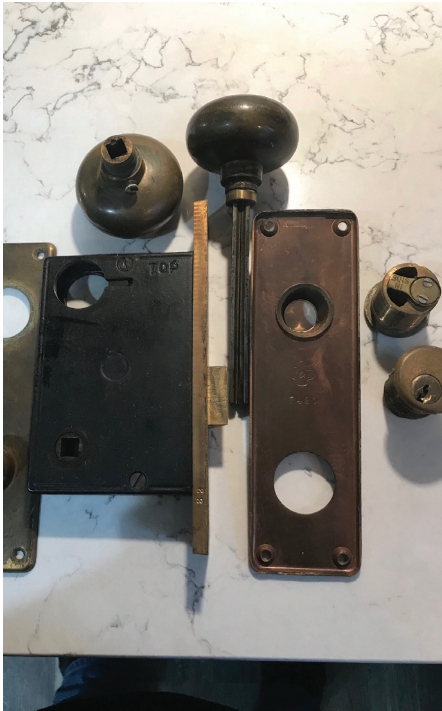
Figure 6. The old lock was a Yale and Towne with two cylinders.
