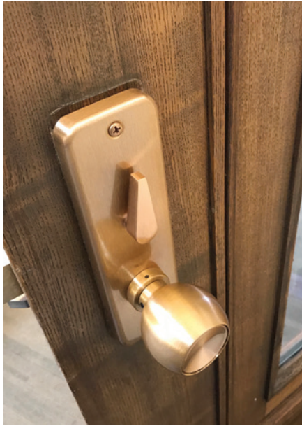
Figure 3. The thickness of both the inside escutcheon and the door made it impossible to screw the standard cylinder into the lock.
