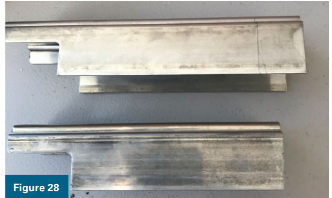
Figures 27–28. These images show the rear cover of the panic bar in two views, with the existing cover on the bottom and the blank replacement cover on top.
