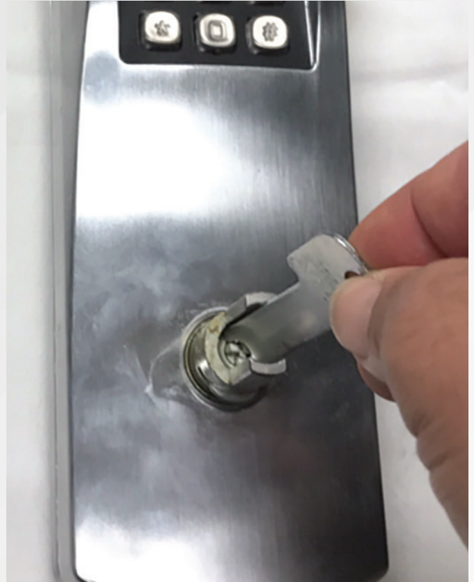
Figure 7. I am rotating the part clockwise to allow the retainer to be pushed upward to accept the lever handle.
