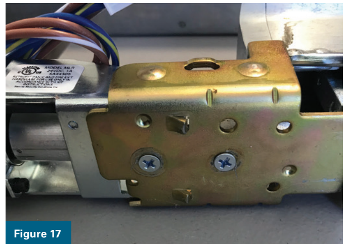
Figures 16 and 17. In Figure 16 , the two red arrows are the screw holes that attach the MLR to the bar, and Figure 17 shows the screws installed.
