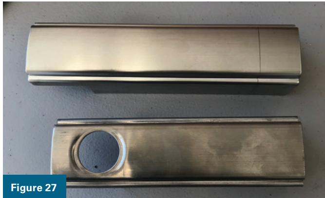
Figures 27–28. These images show the rear cover of the panic bar in two views, with the existing cover on the bottom and the blank replacement cover on top.
