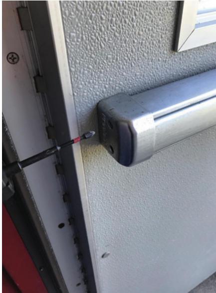
Figure 4. The author is removing the end cap screws.
