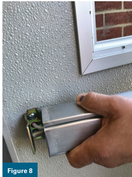
Figures 8 and 9. The author is pulling the end of the bar off the end bracket and the wire.
