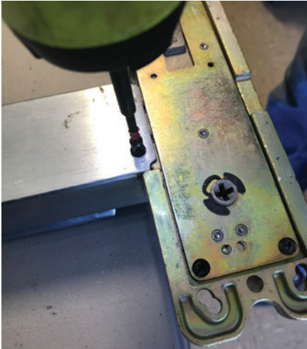
Figure 10. The author is removing the two screws that hold the bar cover to the head of the bar.
