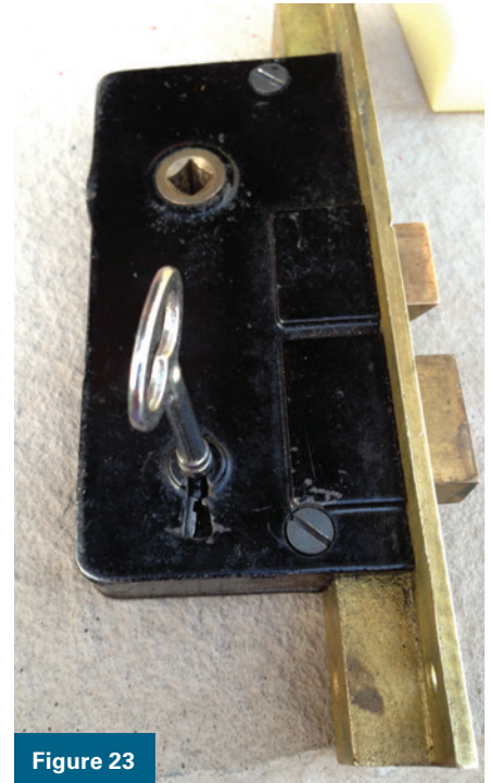
Figures 20-23. These images show the front and back of the working key and the bolt thrown by the key and also retracted.
