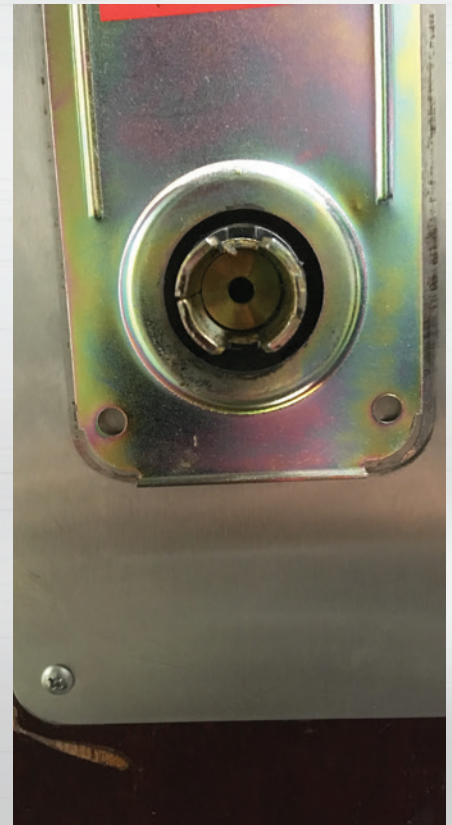
Figure 5. Before fully tightening down the screws, make sure the reinforcing plate is parallel with the edge of the door and centered around the inside drive sleeve.
