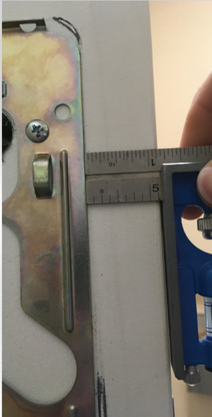
Figure 6. You can use a combination square to ensure the reinforcing plate is parallel with the edge of the door.
