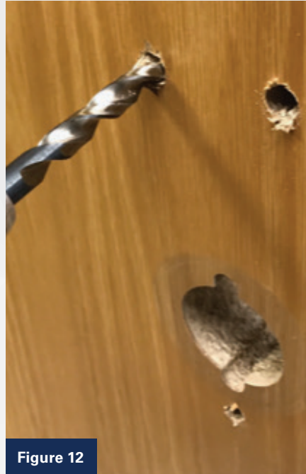
Figures 12 and 13. Three additional mounting holes were required. The author drilled the top hole to the right (Figure 12) and was starting on the top hole to the left. Then he drilled the bottom hole (Figure 13).
