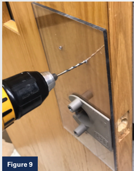
Figures 9 and 10. With the template in position, the author drilled the two top pilot holes (Figure 9) using a \frac{1}{8} " diameter drill bit and the bottom pilot hole (Figure 10).
