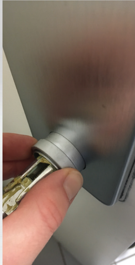
Figure 7. After placing the trim plate over the reinforcing plate, hand tighten the thread ring onto the inside drive sleeve.
