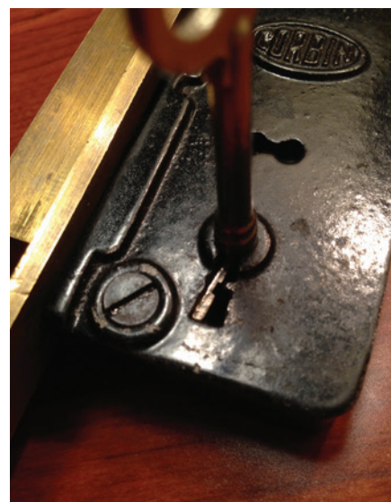
Figure 8. The blank was fitting in, but barely turning.
