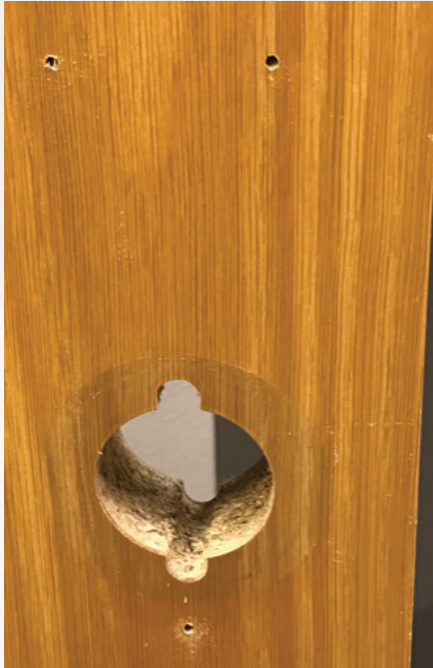
Figure 11. After removing the template, three \frac{1}{8} " diameter holes are visible on the door.
