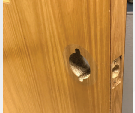
Figure 7. The previously installed Best grade 1 cylindrical lever handle lockset has been removed.
