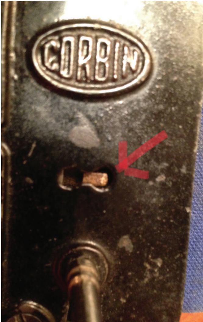
Figure 18. The arrow is pointing to the fence, which is on the right side of the eight.
