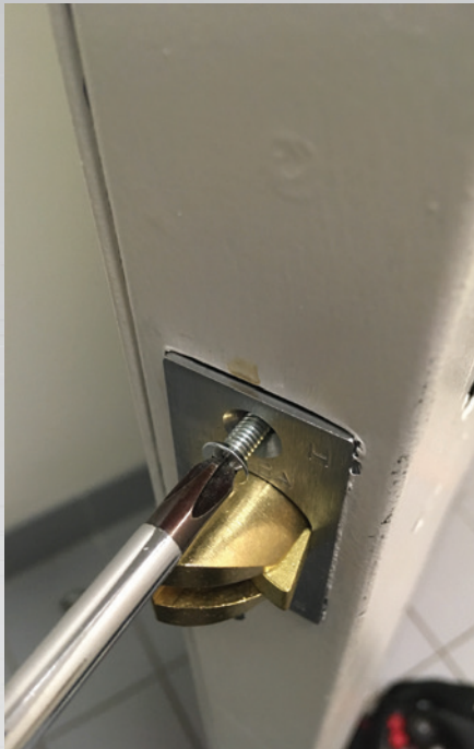
Figure 2. Step two is to install the latch.
