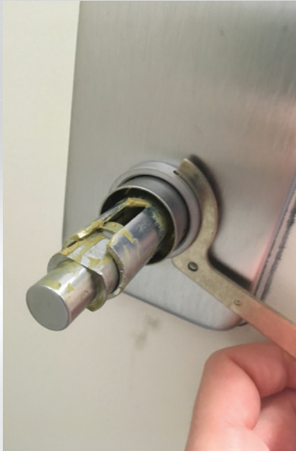
Figure 9. Use the spanner wrench to fully tighten the thread ring.
