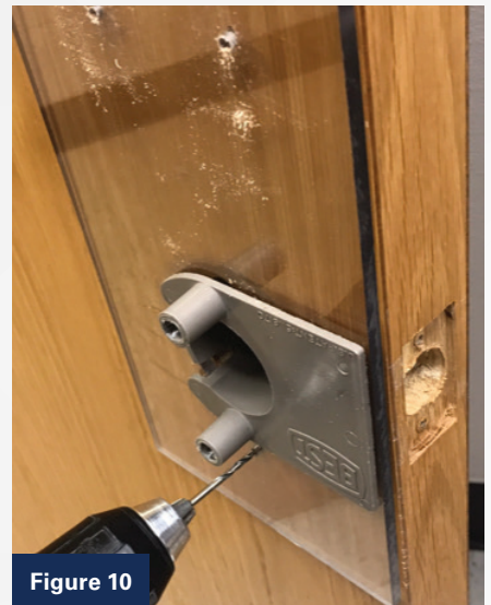
Figures 9 and 10. With the template in position, the author drilled the two top pilot holes (Figure 9) using a \frac{1}{8} " diameter drill bit and the bottom pilot hole (Figure 10).
