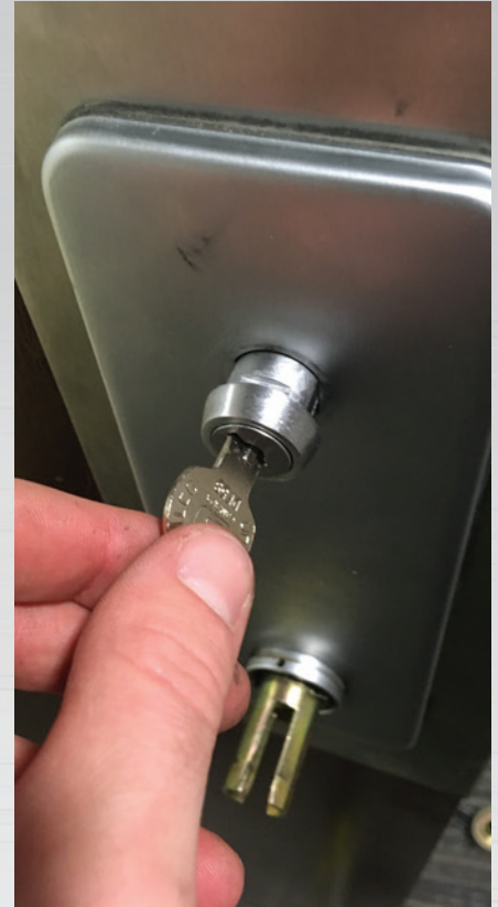
Figure 8. Before using the spanner wrench to fully tighten down the thread ring, begin threading the combination change plug assembly and tighten it until snug.
