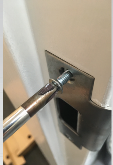
Figure 11. Step seven is to install the strike.
