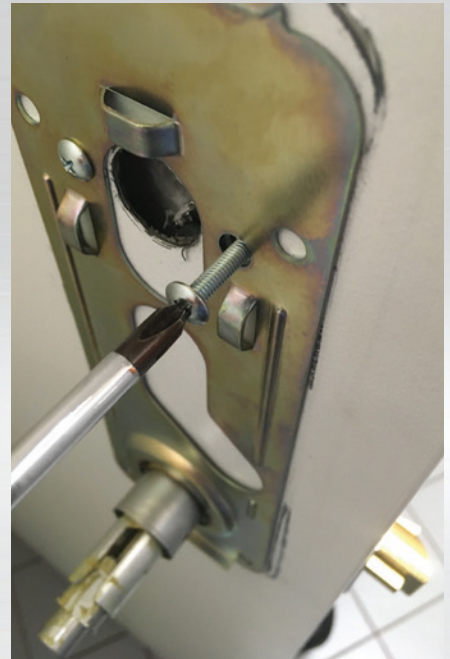
Figure 4. Step four is to install the reinforcing plate.
