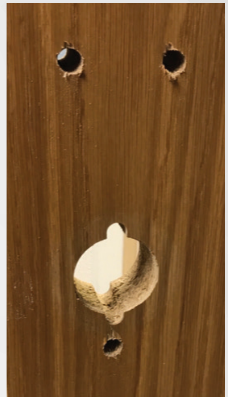
Figure 14. You can see the three additional holes on the opposite side, with the holes completely through door so that you can install the lock.
