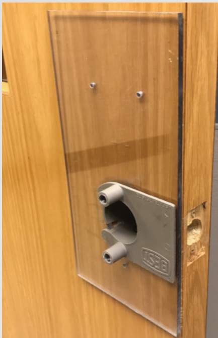
Figure 8. The combination of Plexiglas template and plastic jig is held in place by the cross bore hole.
