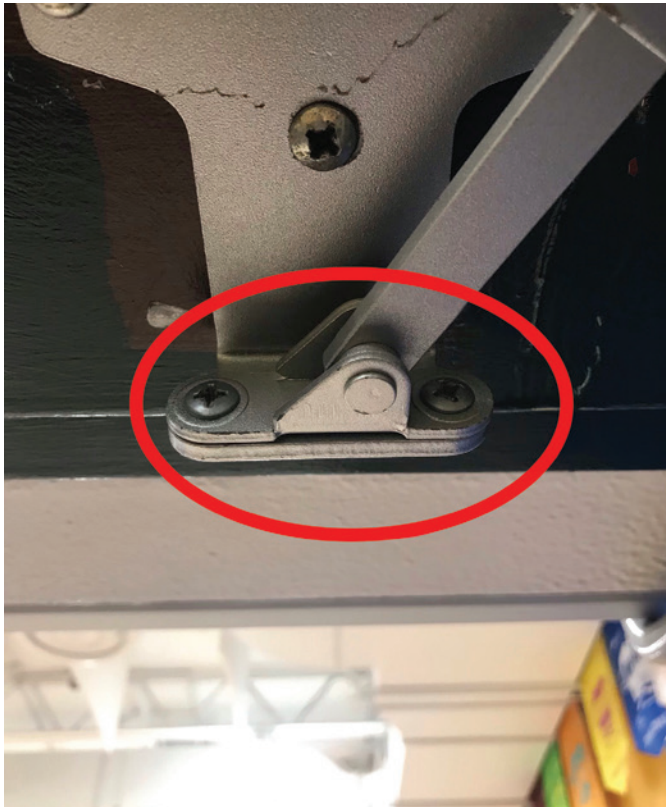
Figure 9. Depicted is a fixed shoe that you simply turn over to shift the arm.
