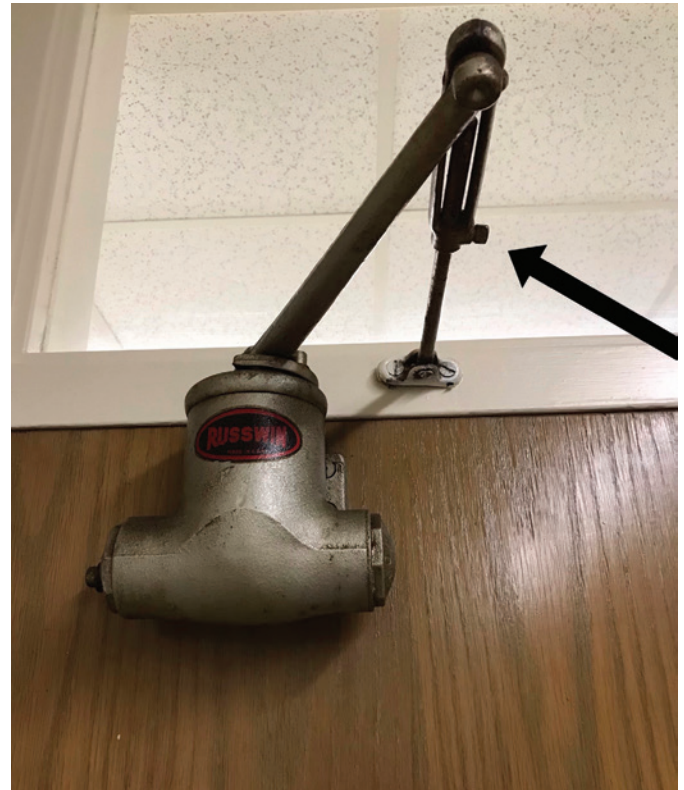
Figure 10. The arrow is pointing to the nut that attaches the main arm to the arm on the shoe.
