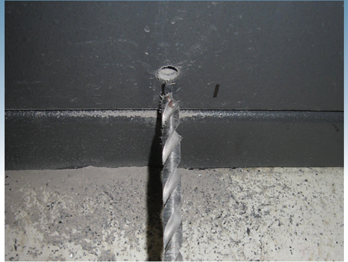
Figure 4. The drill hit dead center on the front of the bolt at just a little over 3" in.
