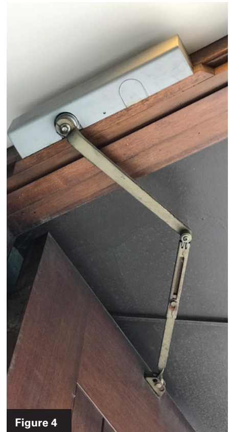
Figures 1-4. The three types of installation for surface-mounted closers are regular arm ( Figure 1 ); parallel arm (PA) ( Figure 2 ); and over-door mounted closed ( Figure 3 ) and open ( Figure 4 ).
