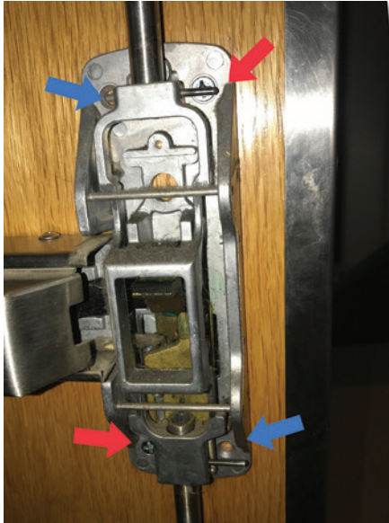
Figure 3. The red arrows point to two of the four mounting screws that were installed, and the blue arrows point to where the second two screws should have been installed.
