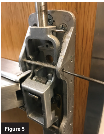
Figures 5-7. These photos show the author using a thin awl to tap the pin out, the pin partly out and where he left it, still attached but out of the way.
