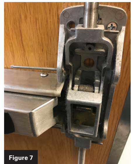
Figures 5-7. These photos show the author using a thin awl to tap the pin out, the pin partly out and where he left it, still attached but out of the way.
