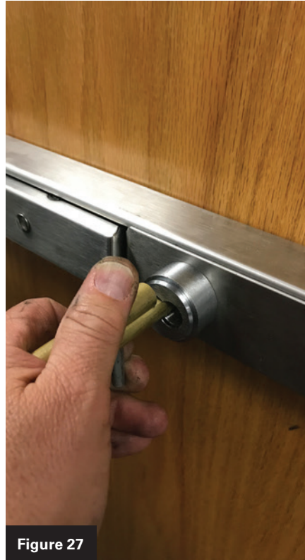
Figures 27 and 28. These images show the operation of the dogging device.
