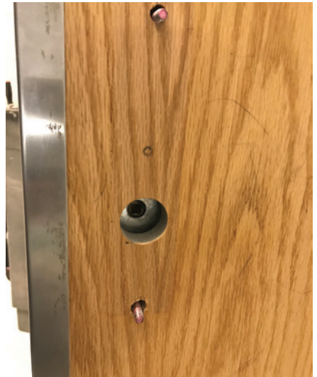
Figure 10. You can see the hub for a spindle on the head of the bar viewed from the outside of the door.
