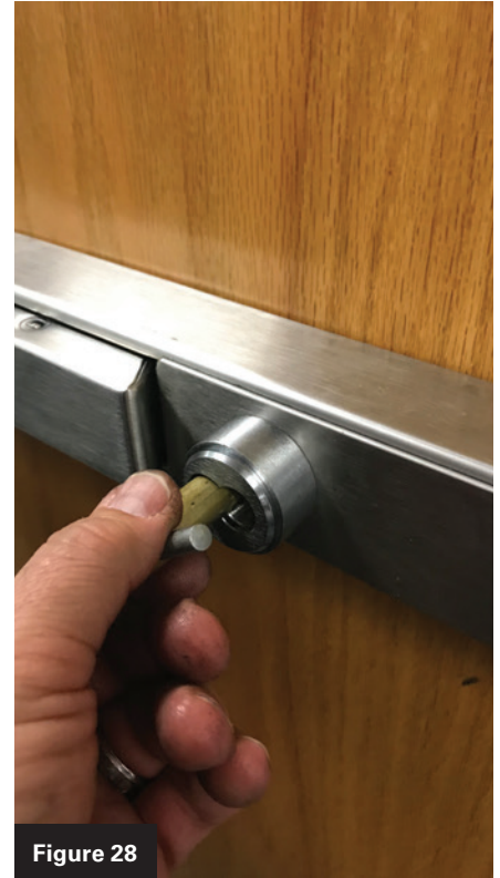
Figures 27 and 28. These images show the operation of the dogging device.
