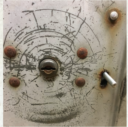
Figure 20. The latch bar lift handle is made from a modified 1/4-20 shoulder bolt.
