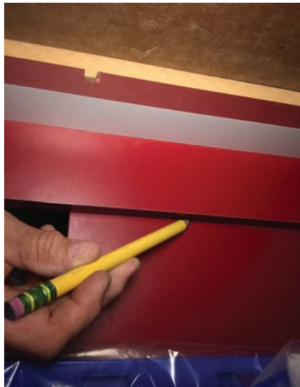
Figure 4. This is a shot from the inside as the author used a pencil to mark the bottom of the frame.
