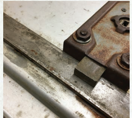
Figure 11. This photo shows where the lock meets the latch bar.
