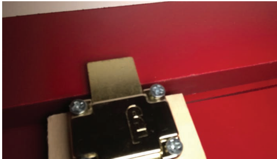
Figure 16. This photo shows the inside view of the bolt locked behind the frame to secure the door.
