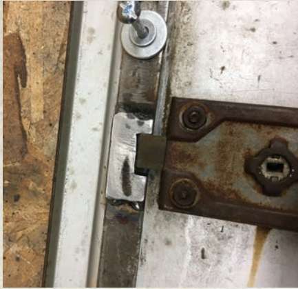
Figure 18. The gate has been cut into the small section of flat bar and welded in place.
