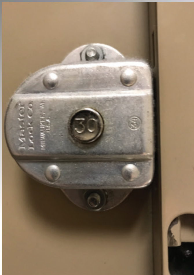
Figure 8. This image provides an inside view of the door of a lift-bolt-style lock.
