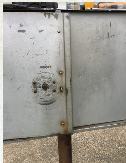
Figure 26. The completed repair is shown, including hinge repairs and adjustment on the secondary door.
