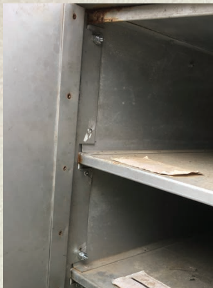
Figure 24. On the inside, rivets were used to further secure the hinge.
