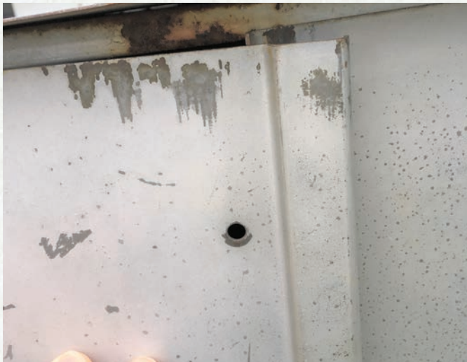
Figure 3. The latch bar is missing, and the doors do not align properly.
