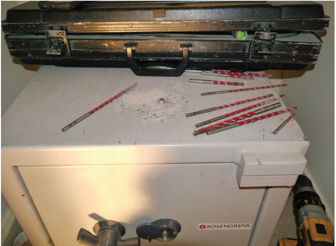
Figure 3. Plenty of drill bits were used for this job — about 10 at $7 each.
