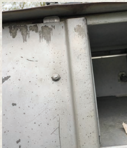
Figure 25. The main door was further adjusted to align properly with the opening. Shims were used on the lower hinge to facilitate reinforcing the adjustment.
