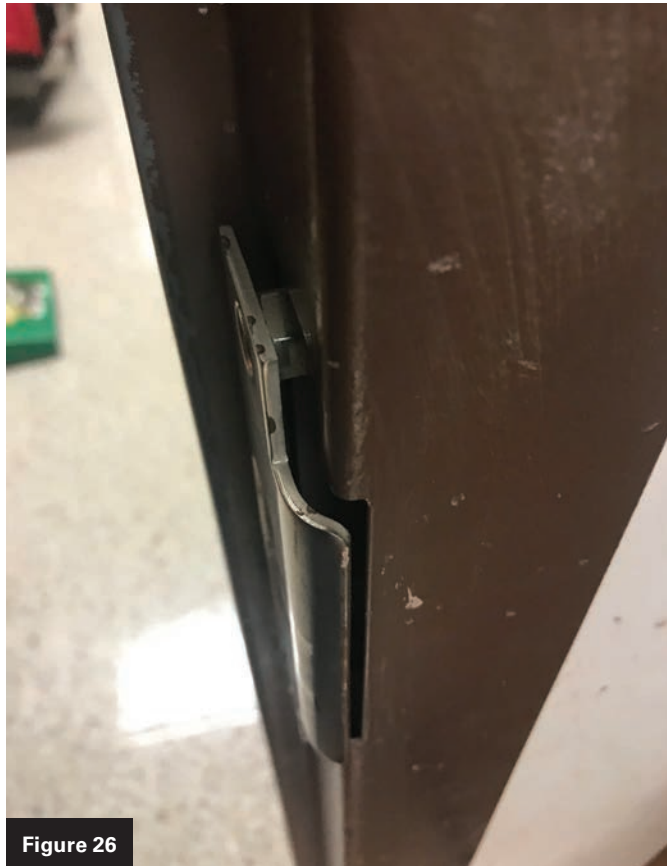
Figure 26 and 27. These photos provide two views of how the maintenance department dealt with too big of a gap on the lock edge.
