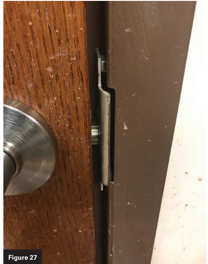
Figure 26 and 27. These photos provide two views of how the maintenance department dealt with too big of a gap on the lock edge.
