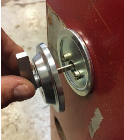
Figure 16. On a standard door, the tailpiece needs to be cut for the inside handle to fit over it.
