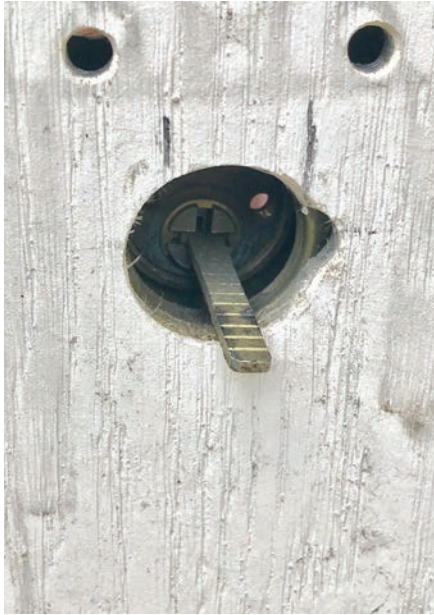
Figure 21. The backplate is removed.
