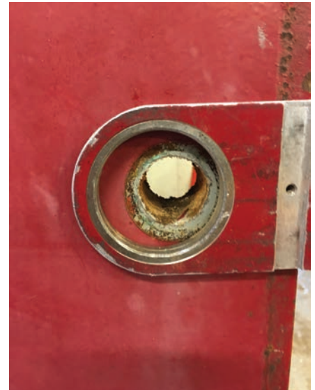
Figure 6. The wood inside the hole and the metal skin around it tells us this is a Kalamein door.
