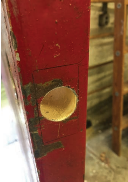
Figure 10. The bolt is marked out.
