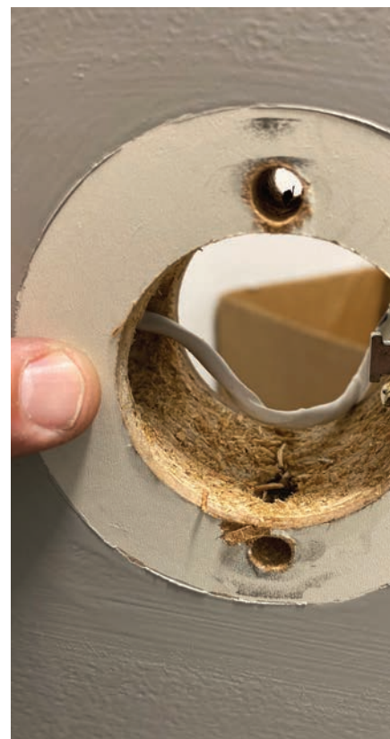
Figure 12. The author is pointing where a notch should have been made so the black wires could pass through without pinching.
