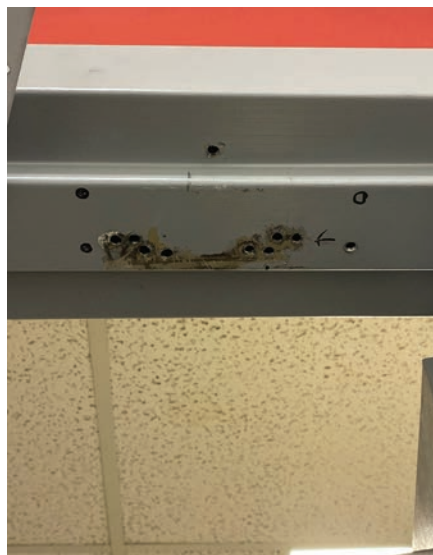
Figure 2. The stop on the frame has a double set of identical holes.
