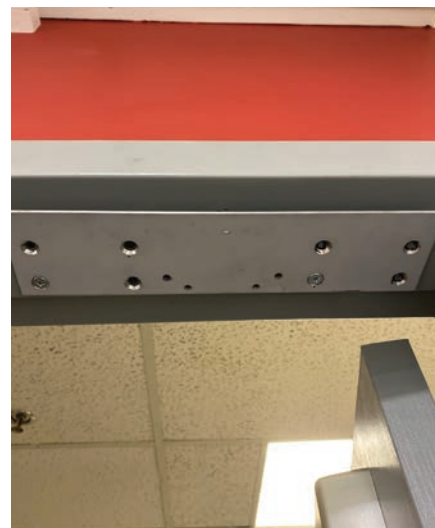
Figure 3. The plate is held on by two screws so the author can spot the rest of the holes.
