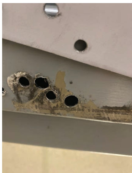
Figure 4. This image shows that the author enlarged the holes that will be under the tapped holes on the plate.
