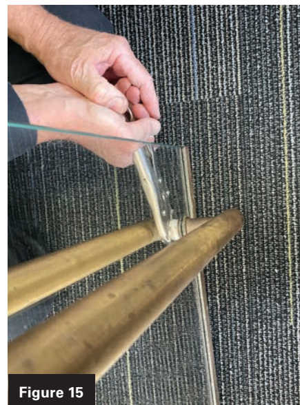
Figures 14 and 15. These images show the author and his associate taping the nut and using locking pliers to loosen it.
