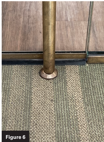
Figures 5 and 6. The floor strike is shown in Figure 5 , and Figure 6 shows the inside handle over it.
