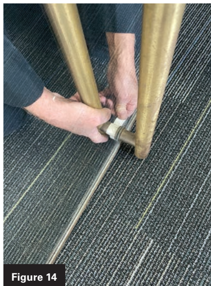
Figures 14 and 15. These images show the author and his associate taping the nut and using locking pliers to loosen it.
