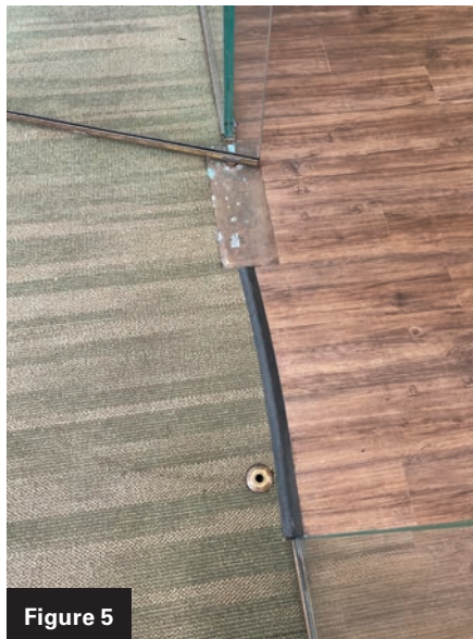
Figures 5 and 6. The floor strike is shown in Figure 5 , and Figure 6 shows the inside handle over it.
