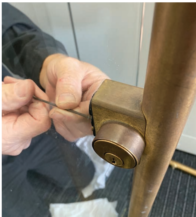
Figure 19. The author is using an Allen wrench to loosen the screw from the inside of the door with the outside housing still stuck to the door.
