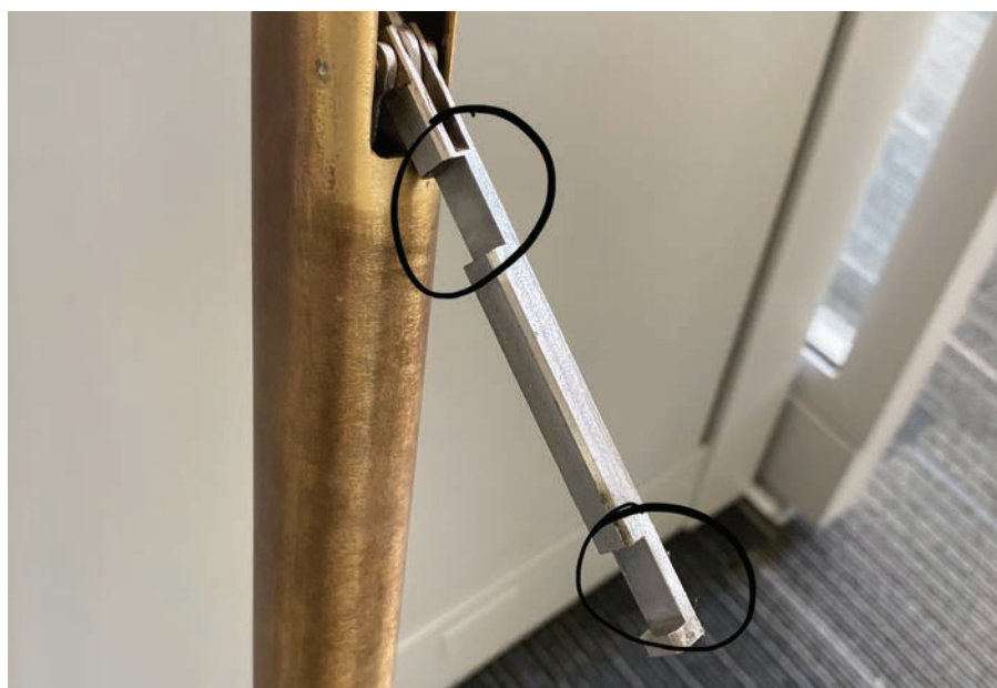
Figure 16. The silver part with the black circles is the actuator.
