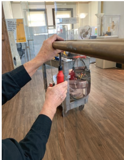
Figure 13. The author is loosening the set screw holding the horizontal tube of the bar.
