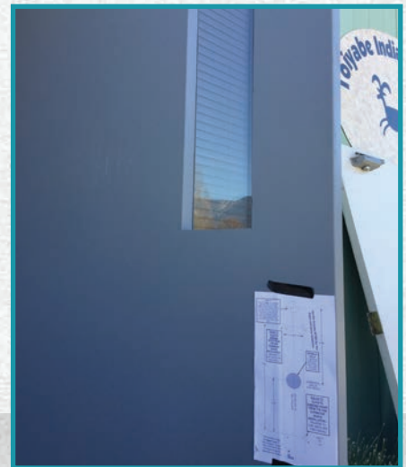
Figure 13. The author likes to put the paper template in place as a guide to ensure he's not drilling extra holes and to help with alignment or orientation. He then uses a center punch to mark the hole locations.
