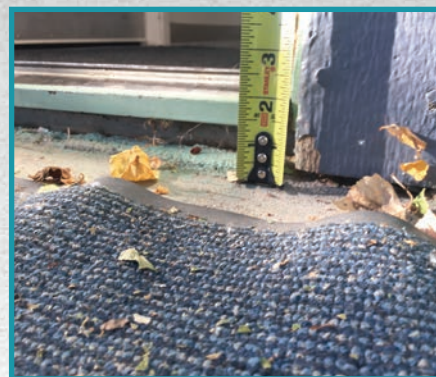
Figure 4. The existing threshold was over 2½" at one edge to the top.
