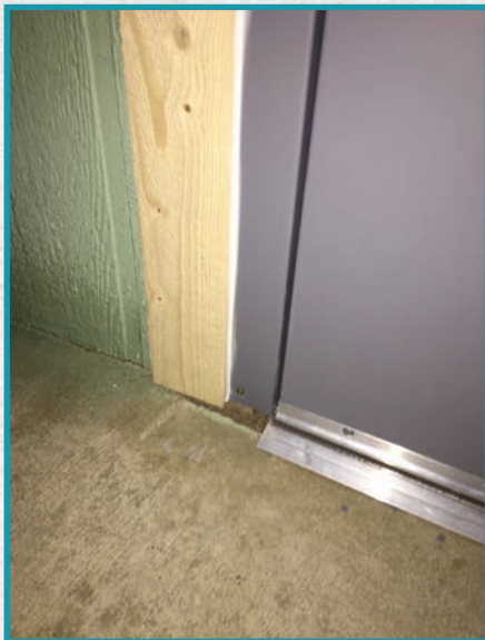
Figure 8. The new threshold is the correct height to meet ADA requirements. Dropping it down avoided the need for a ramp.
