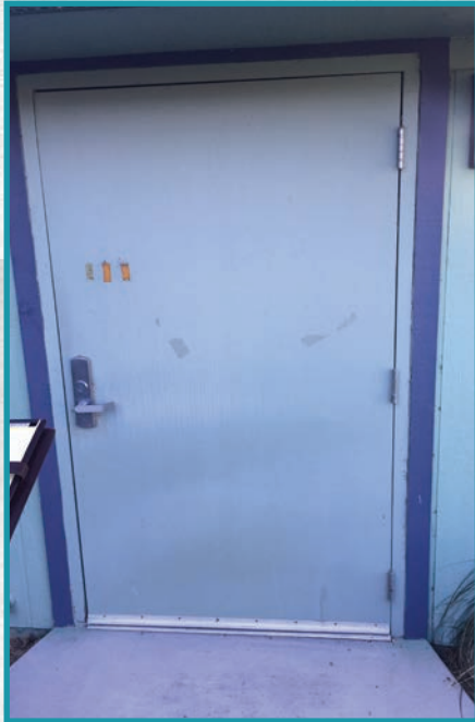
Figure 17. The existing second door is for an ambulance crew exit. It is hinged right hand reverse. The customer wanted the outside hardware removed and door swing changed to LHR for better flow to the emergency parking.
