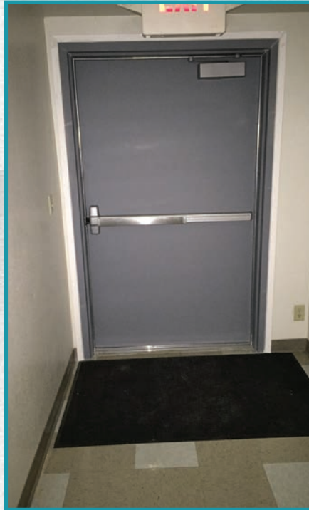
Figure 18. The inside of the newly installed door is shown. The installers reused the original panic without the outside trim.
