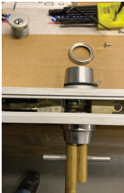
Figure 6. This image provides a view from the top of the rail at the two new Best cylinders.
