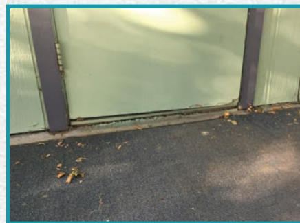
Figure 3. The concrete was not poured level. The author generally loves a challenge, but it seemed best to pass this off to a concrete company to fix.
