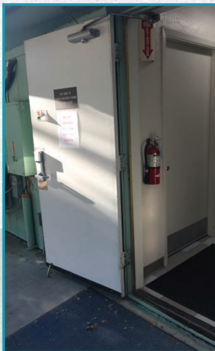
Figure 2. The standard hinges were worn out and needed to be replaced. With all the needed work, it made sense to replace the entire assembly. The other doors looked a little better, but the customer decided that to make all of them look better, it was best to replace them all.
