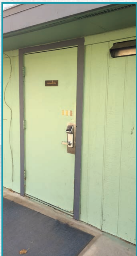
Figure 1. The back door presented the biggest challenge; the threshold was too tall to meet ADA requirements.
