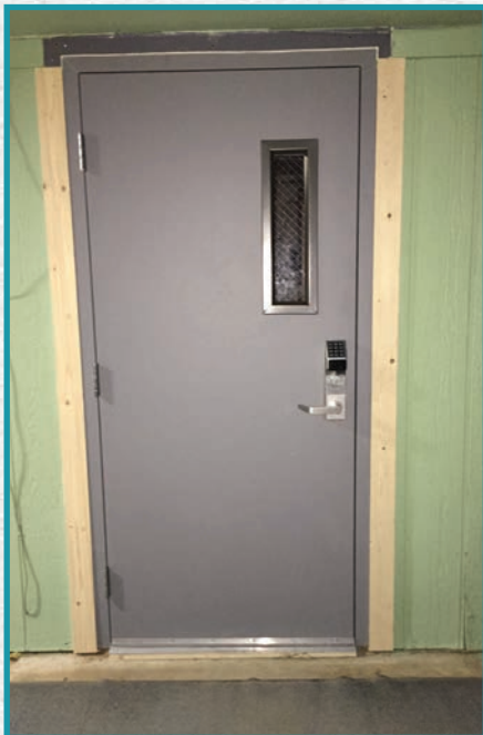
Figure 20. The outside of the back door is shown with the Alarm Lock Networkx outside trim installed. The carpenters trimmed out the door with new wood and caulked off the gaps, leaving painting to the customer's crew.
