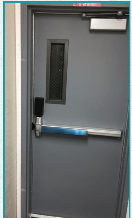
Figure 22. The finished install of the back door is shown, including the battery pack cover.
