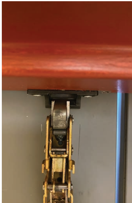
Figure 14. The latch is installed too low on the door. The strike is also not centered on the latch, though it will still work.
