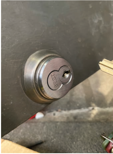
Figure 8. A Best cylinder is installed on the bottom of an aluminum door.
