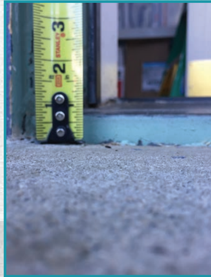
Figure 6. Most residential thresholds are too tall. This one was more than an inch too tall to meet the ADA requirements for commercial buildings.
