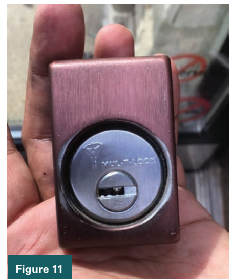
Figures 10 and 11. The new mortise cylinder is shown in the 8650 escutcheon pad.
