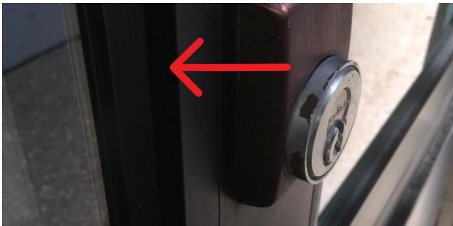
Figure 1. There is not a set screw that holds the mortise cylinder in from the face of the lock, unlike most mortise cylinders.
