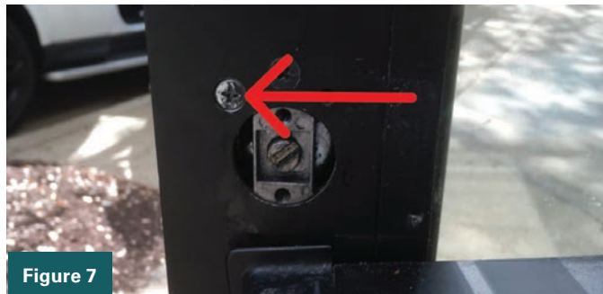
Figure 5. Remove the two screws holding the device to the door.
