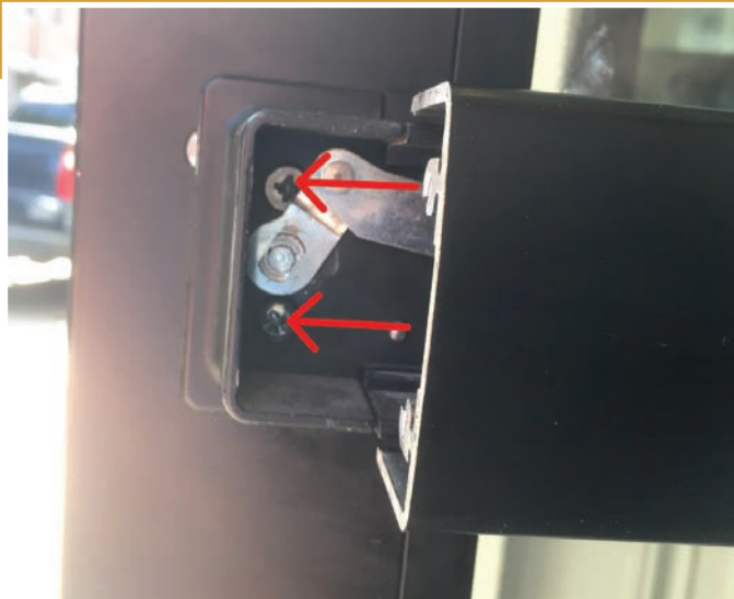
Figure 5. Remove the two screws holding the device to the door.
