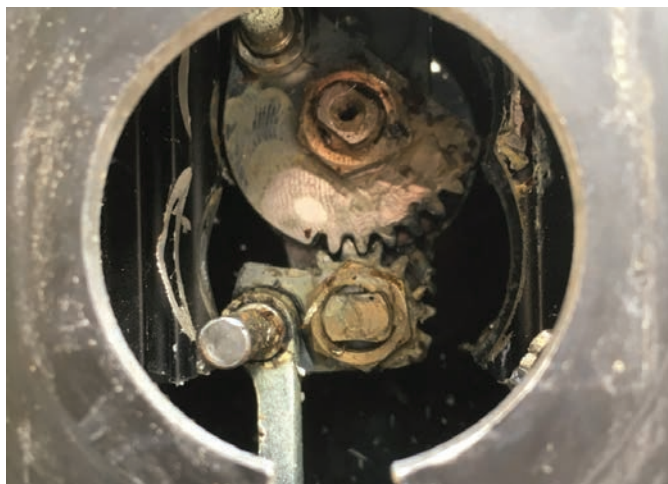
Figure 9. This image shows the outside view once the 8650 escutcheon pad is removed.
