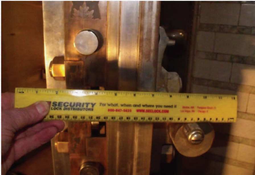
Figure 16. Here, we see the thickness of the outer door.
