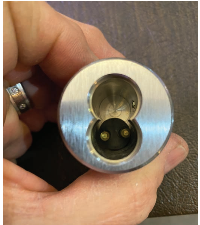
Figure 24. The spacer is an example of installing everything in the box out of ignorance.
