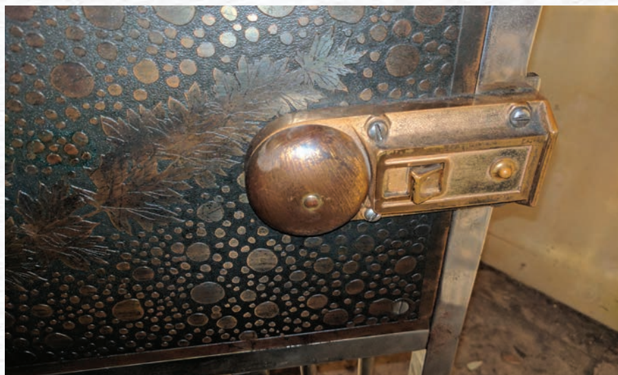
Figure 25. The Rim Latch lock with bell alerts you if someone is entering.
