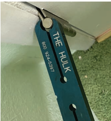
Figure 4. Residential hinges need to be adjusted one knuckle at a time. The "hulk" tool provides this adjustment without opening the door. Tighten the tool on a knuckle and use the tool a little like a wrench to move the knuckle. Then move to another knuckle and move it the same amount.
