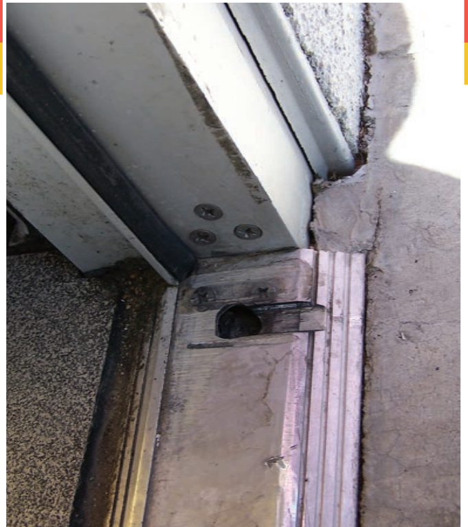
Figure 7. Here is the result of the worn-out hinge: The bottom bolt of the exit device has scraped a groove in the threshold.
