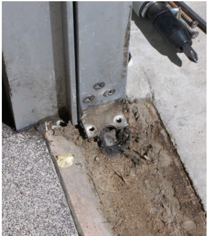
Figure 9. Removing the old thresholds reveals the mounting bracket for attaching the threshold to the jamb.
