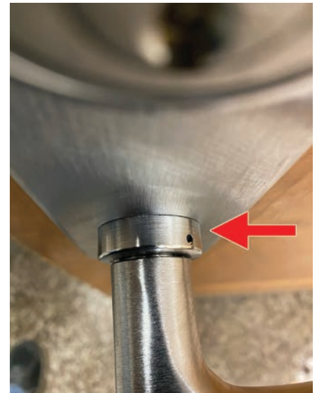
Figure 3. The installer nearly had only hand tightened on the "rose ring" (red arrow).
