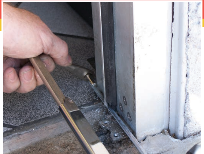
Figure 11. The doorstop had to be cut away to allow room for the new threshold.
