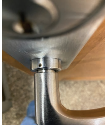
Figure 5. Notice the large gap between the ring and the lever.
