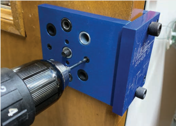
Figure 7. If applicable, drill for the anchor plate lugs.
