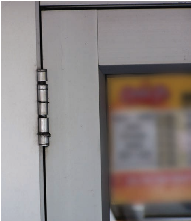
Figure 6. This hinge is worn out. No amount of adjustment is going to help this one, and it needs to be replaced.
