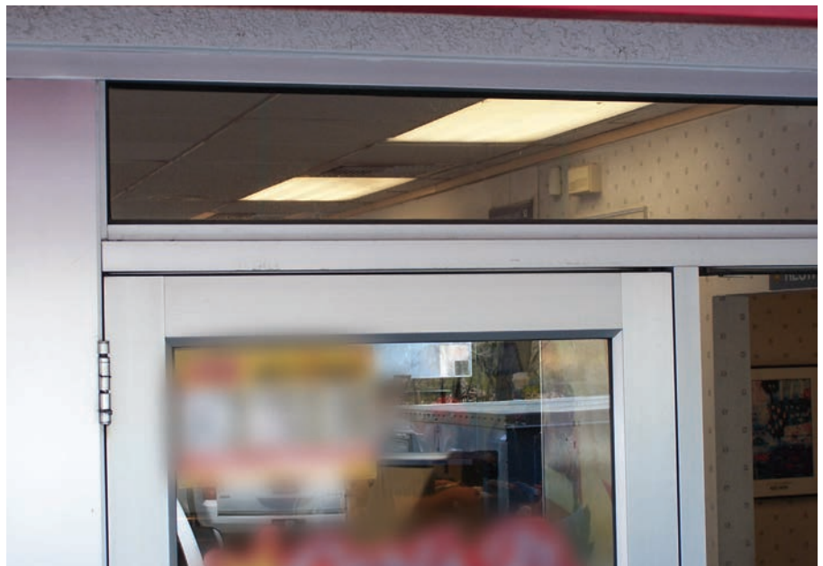
Figure 5. This door has dropped. You can see the gap between the top of the door and the header.
