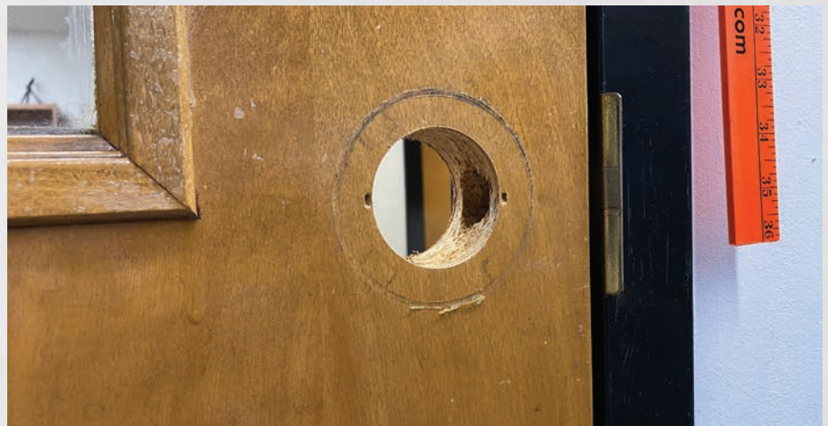
Figure 3. Start by removing the existing hardware, if applicable, including the latch.
