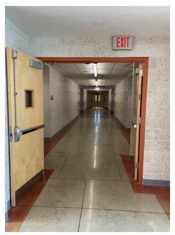
**Figure 1.** Two corridor doors swing in opposite directions within the same opening.
