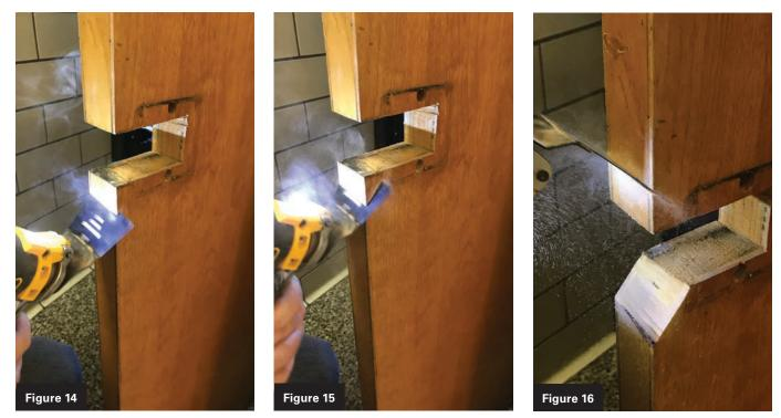
Figures 14-16. Each cut took about a minute to finish with an oscillating saw.
