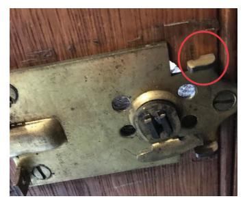
Figure 8. The red circle indicates one of the two hooks built into the backplate.
