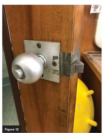
Figures 12 and 13. An old unit lock and its prep are shown.
