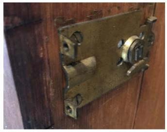
**Figure 9**. This view shows the two threaded holes that the flathead screws above and below the latch screw into to complete the installation.
