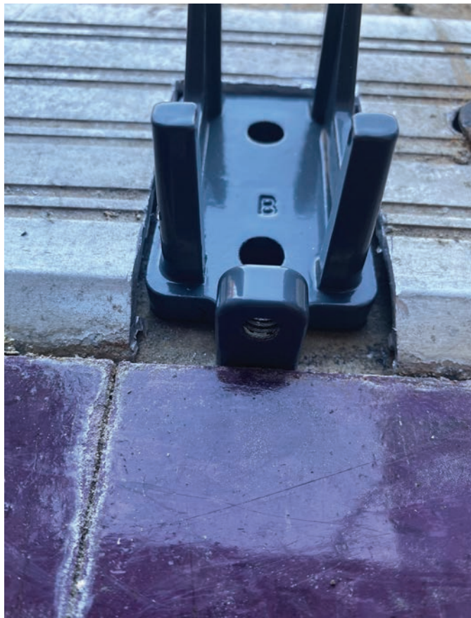
Figure 8. The bracket is shown in relation to the finished floor and saddle.
