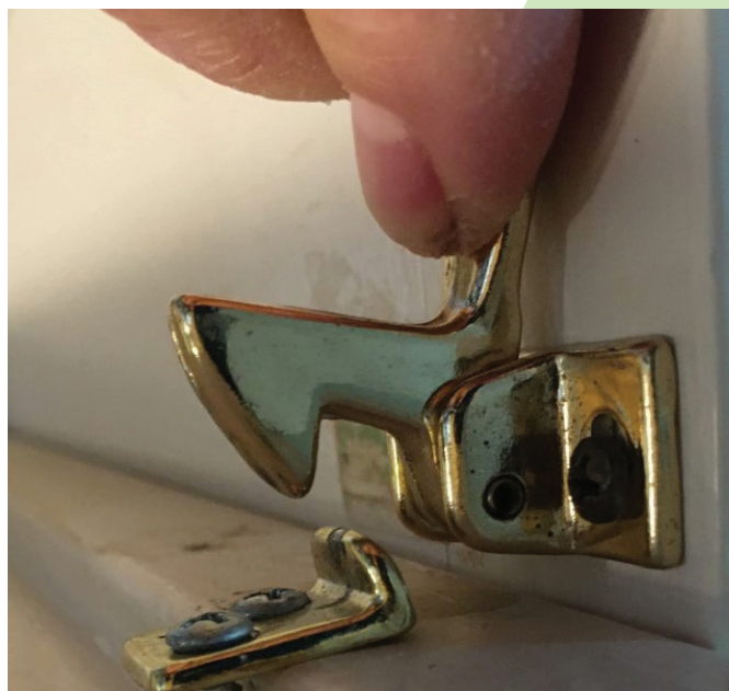
Figure 2. A typical elbow catch is engaged into the L-shaped strike plate in the latched position, keeping the door from opening.
