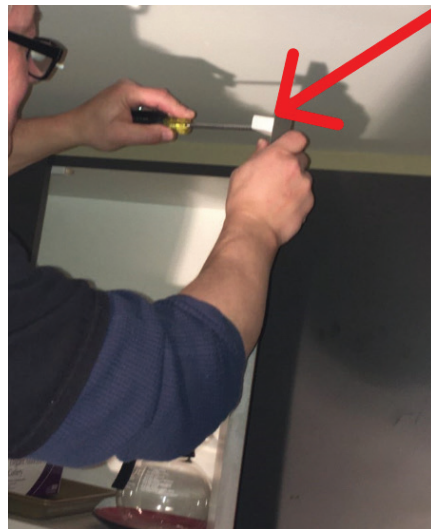
Figure 14. When the door is closed, the activator pushes the bolt through to the catch side.
