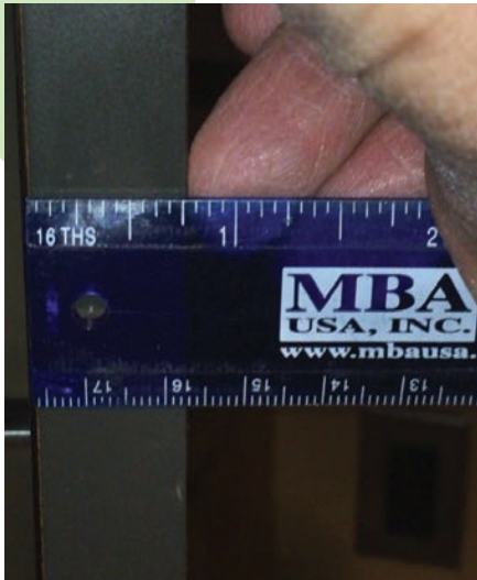
Figure 10. Before starting the install of the DDLK, measure the thickness of the cabinet.
