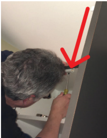
Figure 13. Mount the latch on the exact center of the mark that you made.
