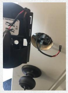
Figure 15. There is a small rectangular hole in the plate through which the wires will be extended.
