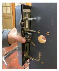
**Figure 4.** The author is holding the trim against the door and lining up the posts/ studs with the existing holes in the door.
