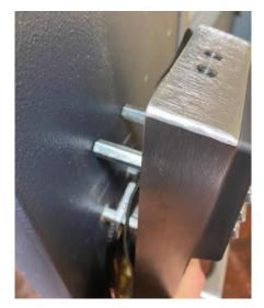
**Figure 8.** The author is holding the trim against the door and partially in the existing holes.
