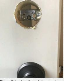
Figure 10. Looking through the cross-bore hole, you can see the holes on each side where the mounting screws will pass through and the slot in the middle that the tailpiece will go through.
