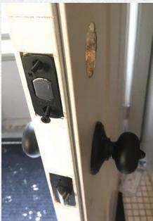
Figure 8. The latch bolt is in place, and the screws are started.
