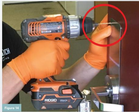
Figures 13 and 14. Before installation, the author used his center punch to center each screw (Figure 13) and then used a pilot bit to pre-drill the screw holes (Figure 14).
