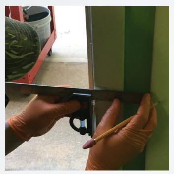
**Figure 18.** The author measured the 12C electric strike and transferred the measurements to the doorframe using a carpenter's square.
