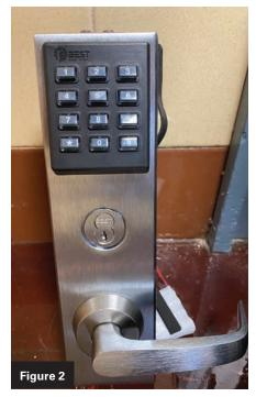
**Figures 1 and 2.** The author did a retrofit job removing the existing key operation-only trim (*Figure 1*) on a PHI panic device and replacing it with a BEST EZ keypad trim (*Figure 2*).
