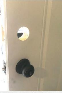
Figure 2. An inside view of the door shows the 2%" cross bore hole for the deadbolt lock.
