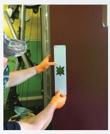
**Figure 8**. The remodeler's plate covered all of the holes in the door.
