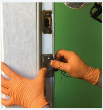
Figure 19. The author held the electric strike up to the doorframe with his markings to visually check the measurements again.
