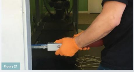
Figures 20 and 21. To make the cutout for the electric strike, the author used both wood chisels (Figure 20) and his electric file to clean things up (Figure 21).
