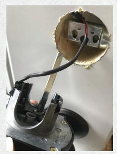
**Figure 11**. Insert the wires into the hole just above the latch bolt.
