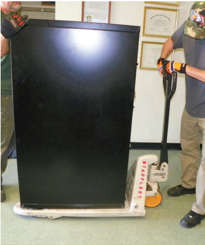
Figure 4. We are slowly releasing the pallet jack hydraulics to allow the cabinet to set on the block. When the pallet jack hydraulics are fully released, the block of wood will suspend the cabinet about \frac{3}{8} " in the air above the pallet jack forks. It is at this point your assistant has the easy job of balancing the cabinet in place. The pallet jack will remain where it is, once again for safety reasons. If the load becomes off balance for any reason, the pallet jack will catch it before it becomes an issue.
