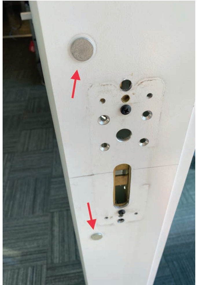
Figure 9. The author screwed the screws into the sexbolts (red arrows).
