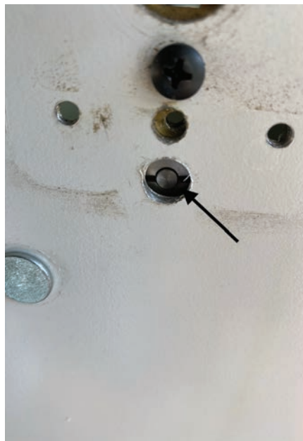
Figure 13. The arrow is pointing to the bottom rod screw.
