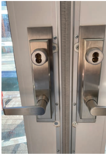
Figure 10. The completed trims are installed.
