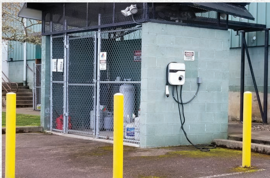
Figure 6. Areas with dangerous machines or chemicals or those with high voltage should have single keyed locks to prevent unneeded access.
