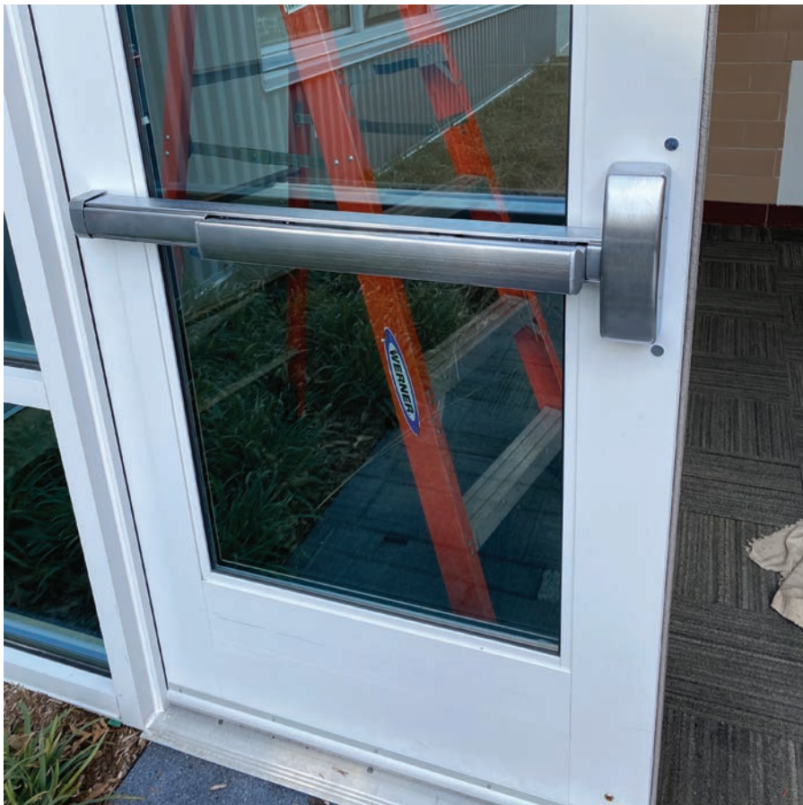
Figure 1. A PHI MLR concealed vertical rod panic device is shown.
