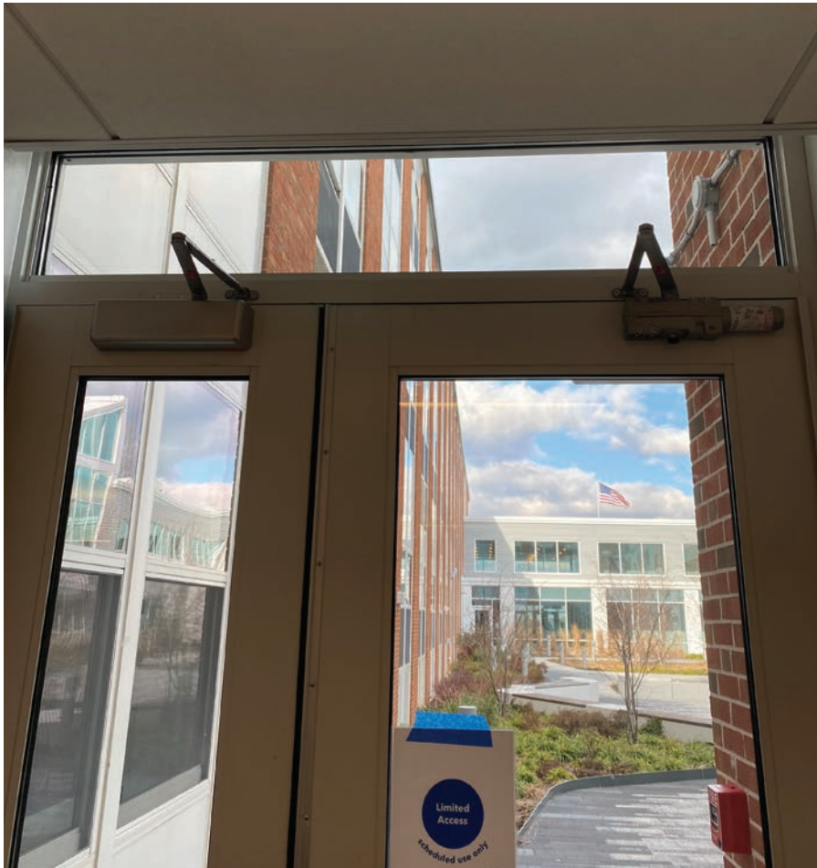
Figure 3. The closer on the left is not preloaded. On the right door, the arm is close to where it should be.
