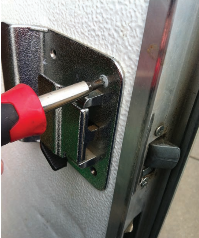
Figure 5. The author is removing the lock from the door.
