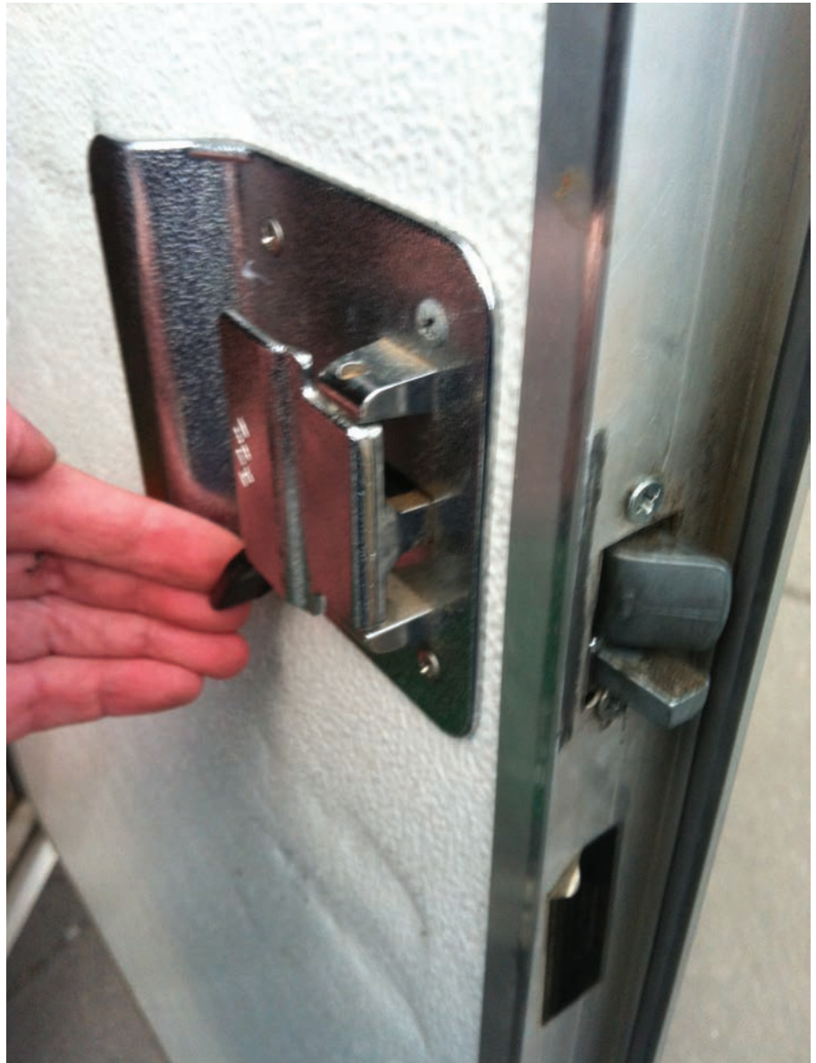
Figure 3. The bolt is extended and won't retract.
