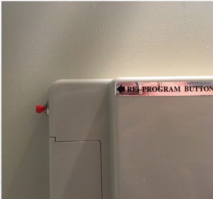
Figure 7. To change the combo, depress the red button and immediately enter the new desired code.
