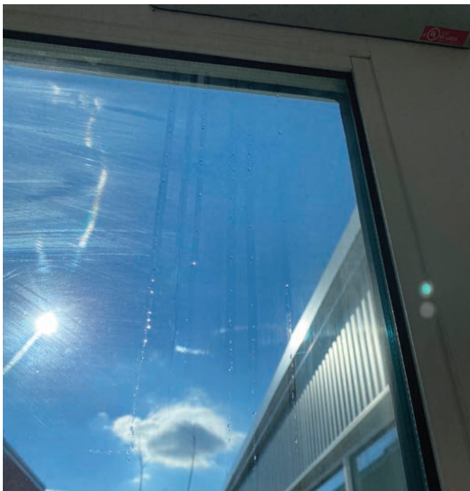
Figure 1. You can see the tracks of hydraulic fluid leaking out of a door closer and running down the door.
