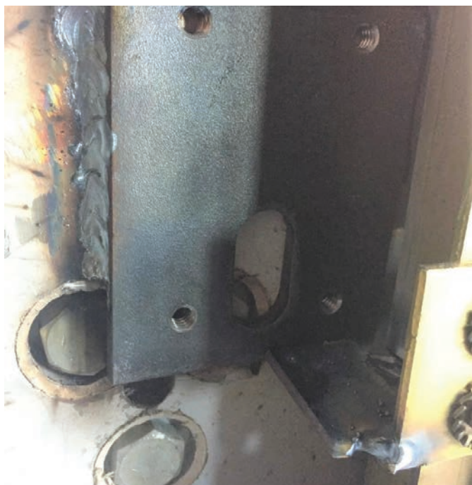
Figure 9. The standard-footprint plate is welded in place.
