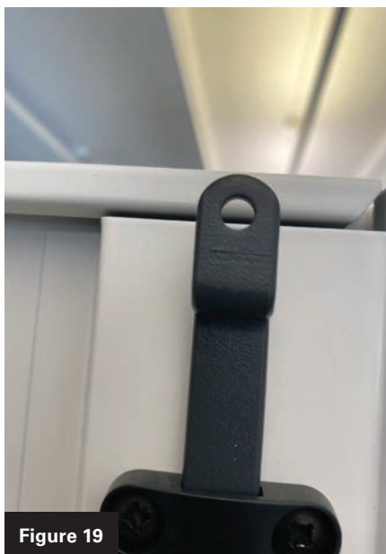
Figures 19 and 20. The top rod is in the locked and unlocked position.
