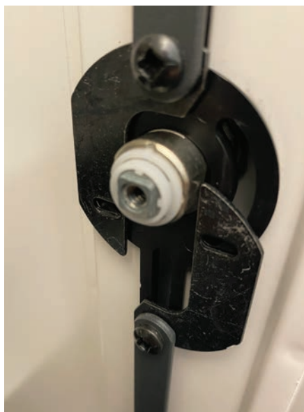
Figure 18. The top and bottom rods are in place along with the plastic bushing.
