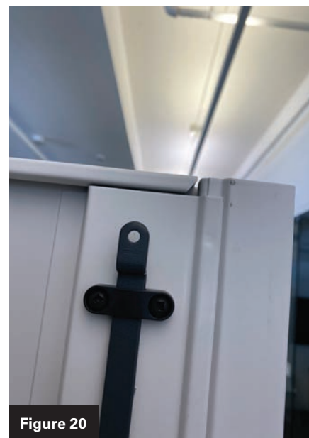
Figures 19 and 20. The top rod is in the locked and unlocked position.
