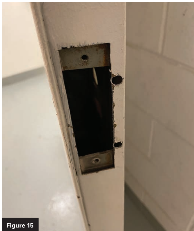
Figures 15 and 16. The author drilled two holes and bent the obstruction out of the way.
