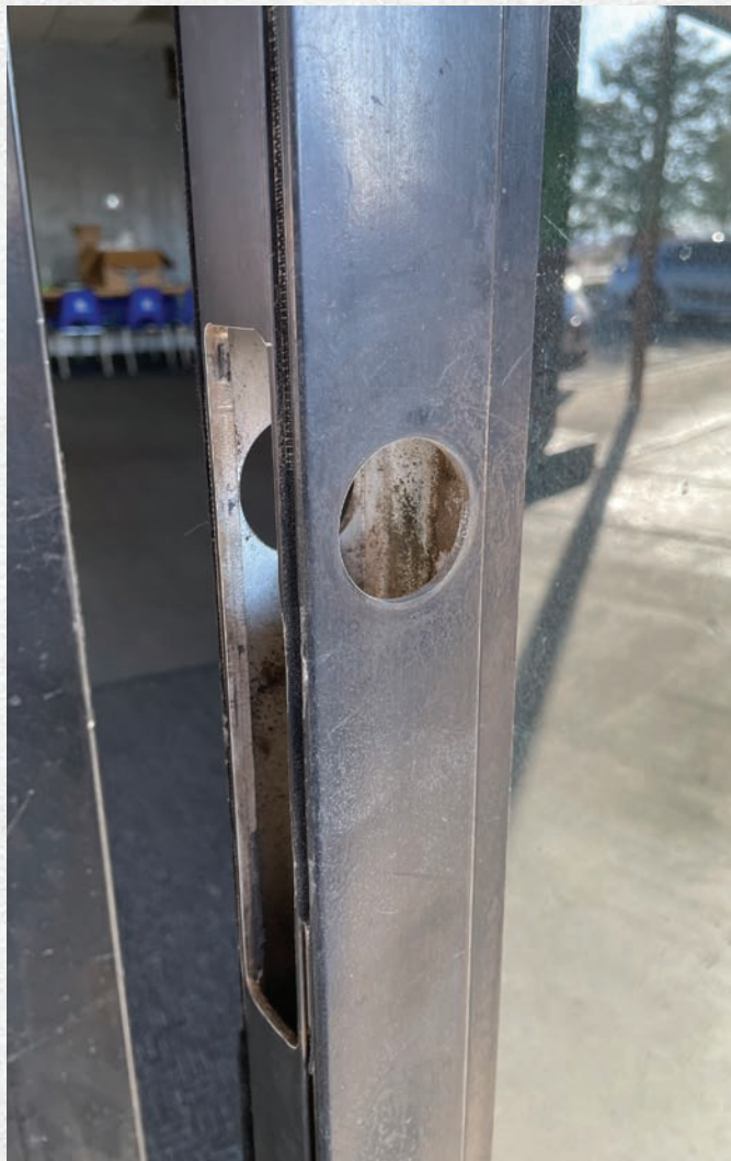
Figure 3. One nice part of swapping the swing bolt for a latch is they use the same cutout in the door.
