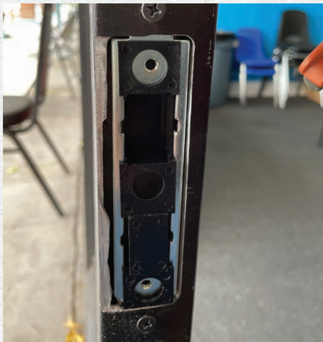
Figure 19. A plastic filler is supplied with the Adams Rite 4901 to fill the bottom hole of the strike. This also allows the strike to be used for either hand.
