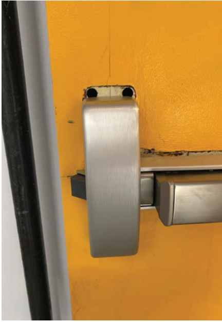
Figure 3. These two large through holes are remnants of the old mortise panic bar.
