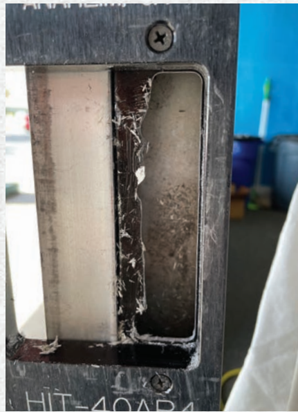
Figure 17. Rout the opening slowly. The difficult part is seeing the front face of the door and not cutting through it. Once most of the material is removed, carefully reset the depth of the router bit to just cut away the thickness of the strike as you exit to the front. If the author were to do this again, he would add a spacer to the face of the door to create a gap between the door and his angled aluminum.
