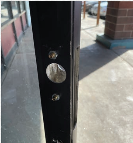
Figure 10. After installing the lock and outside trim, the author realized what he was missing: the mounting bolts for the inside paddle. The instructions for the Alarm Lock don't include the inside paddle, or you could use the mortise panic version. The author had to take it back out and line up for these.
