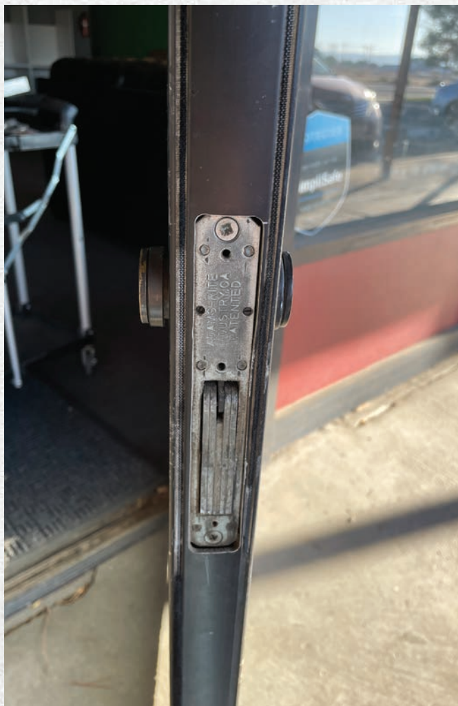
Figure 2. The swing bolt deadbolt was missing the face plate when the author started giving easy access to the set screws.
