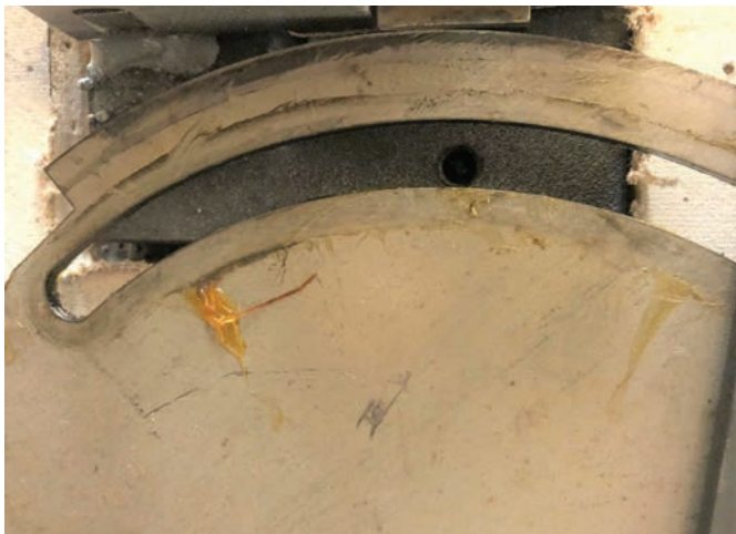
Figure 5. This is the track used to restrict throw and retraction of the bolts. You can see the hole that the offending bolt fell out of.
