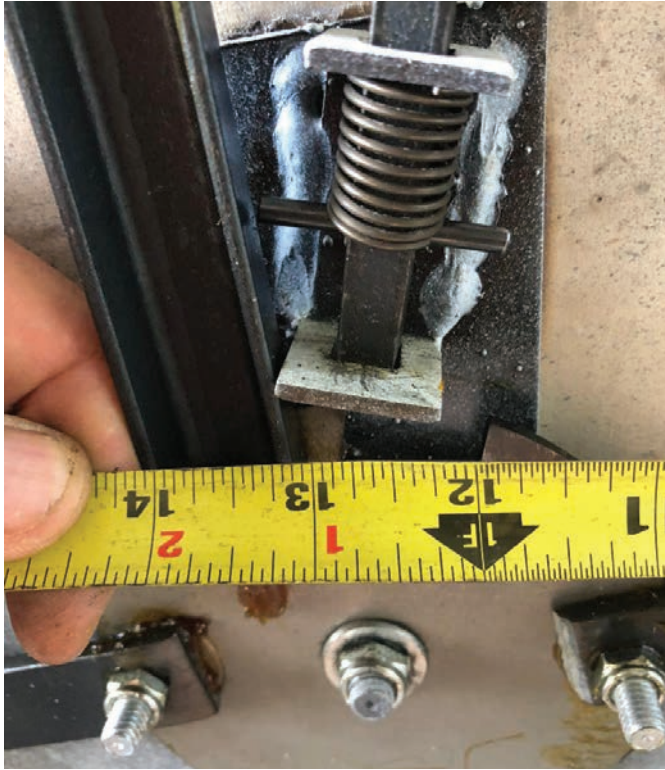
Figure 9. In this photo, you can see the distance from the opening side of the door to the second external relocking device.
