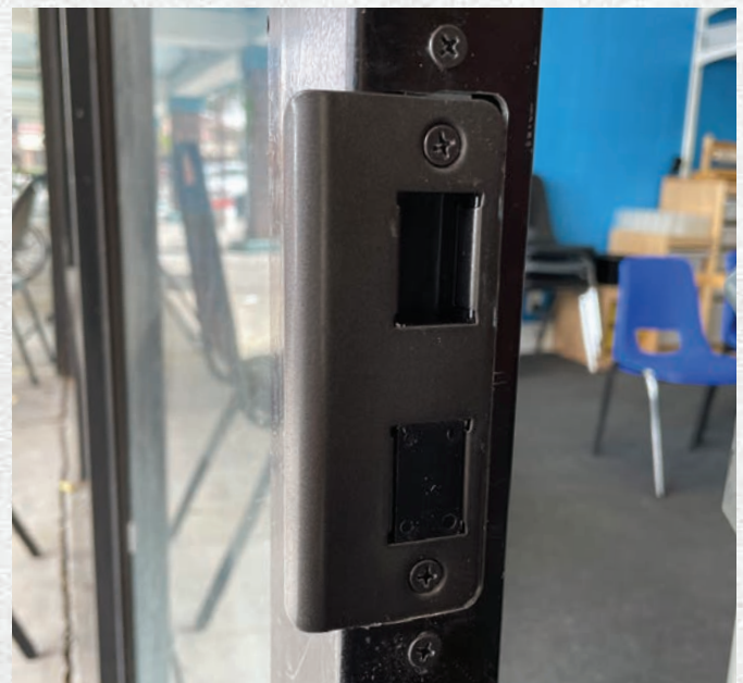
Figure 20. You can now install the strike in the opening. The author noticed the opening looks a little large in this picture at the top. His guess is that he must have tilted the router slightly as he routed this area. It is slight, as he didn't notice it after he installed the lock. Something he says he could have done to hide this better is to have used a black marker to color the bare aluminum.
