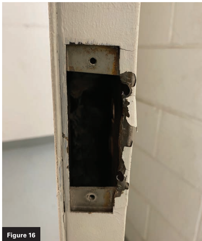
Figure 14. The prep for the old lock is shown.
