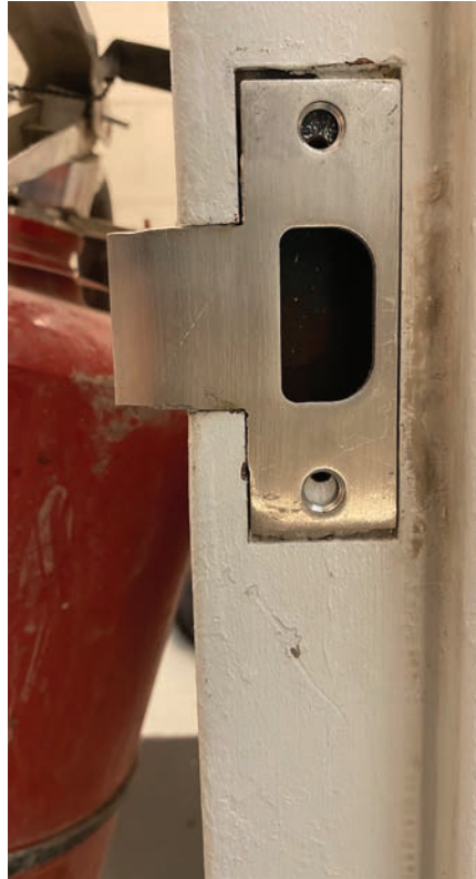
Figure 8. The modified strike is in the prep.
