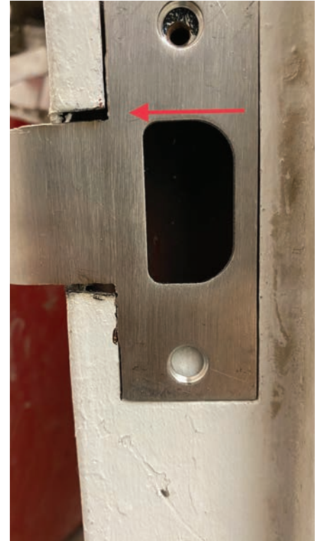
Figure 9. Now there is a clear spot to drill a new bottom hole..
