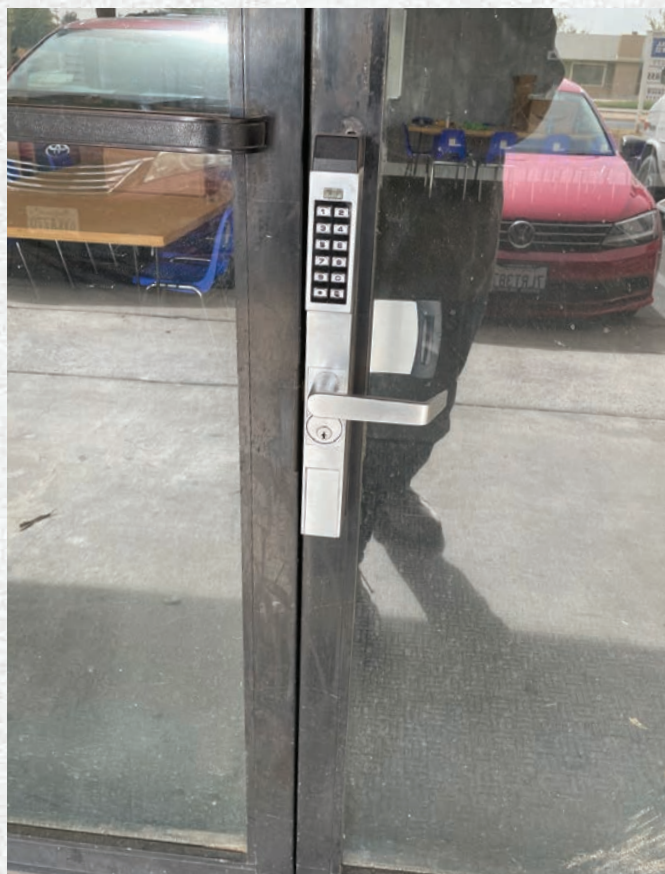
Figure 22. This is the final product after the author adjusted the arms on the Jackson concealed overhead door closer to create the additional gap so the door would close and latch properly. The upper push/pull bar mounting hole was filled with a little caulking.
