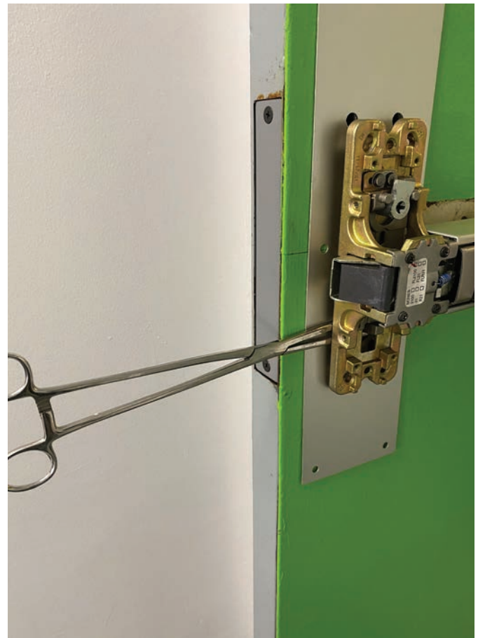
Figure 6. The large hemostat is clamped on the finger lift of the trim, holding the trim against the outside of the door.
