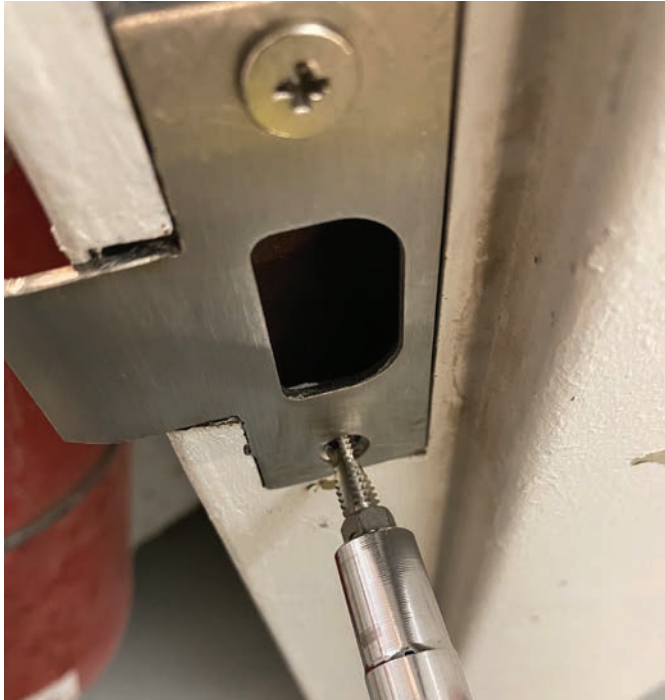
Figure 10. The author is using a Klein Tools Multi Tap Bit screwdriver to tap the bottom hole for 12-24.
