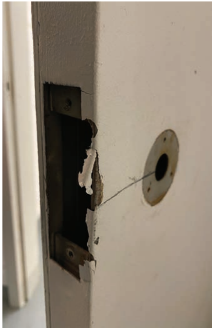
Figure 17. Here, you can see the horizontal centerline and the small spindle hole from the old mortise lock.
