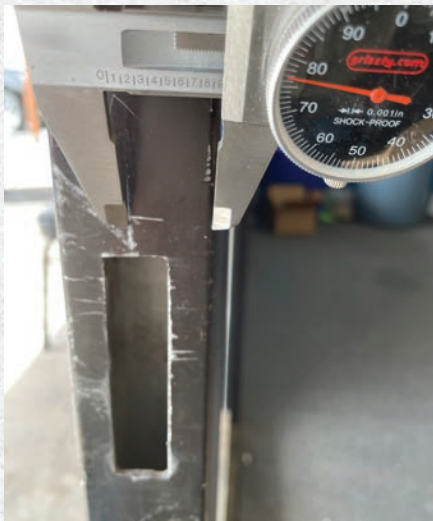
Figure 13. The strike requires placing the holes dead center on the inactive door. The author likes using calipers. They provide a very accurate measurement, and you can use the sharpened end to scratch or create the mark.
