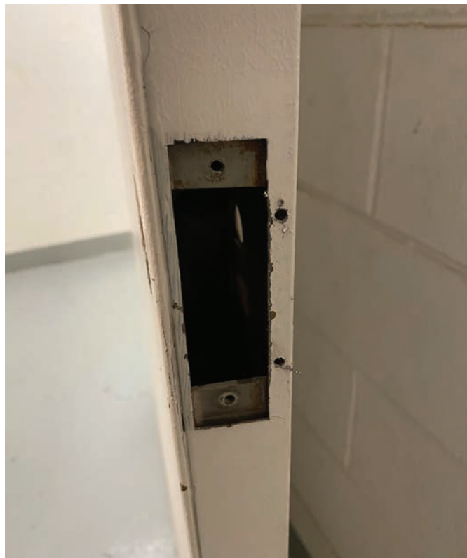
Figure 14. The prep for the old lock is shown.
