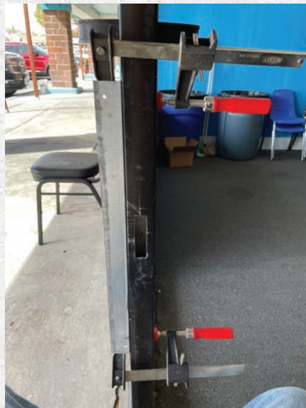
Figure 14. The door is too narrow to support the router or a template. You can use a piece of angle aluminum to provide a wider surface.
