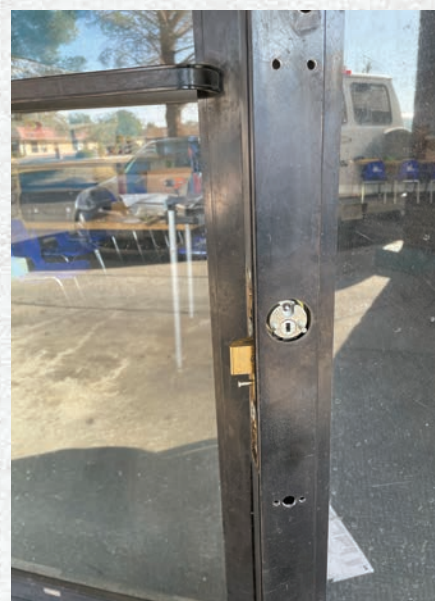
Figure 7. Once the holes are drilled, you can install the lock with the cam assembly in the cylinder hole.
