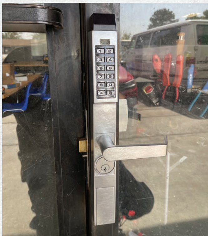
Figure 9. The outside assembly is installed; this model is push-button only. Alarm Lock offers it with a proximity card reader. The cylinder below is for key override in case the batteries go dead. The mortise cylinder cam must be ordered from Alarm Lock, as it's not a standard or common cam. The author recommends you order it with an interchangeable core cylinder or order that cylinder separately if Alarm Lock offers the appropriate cam.
