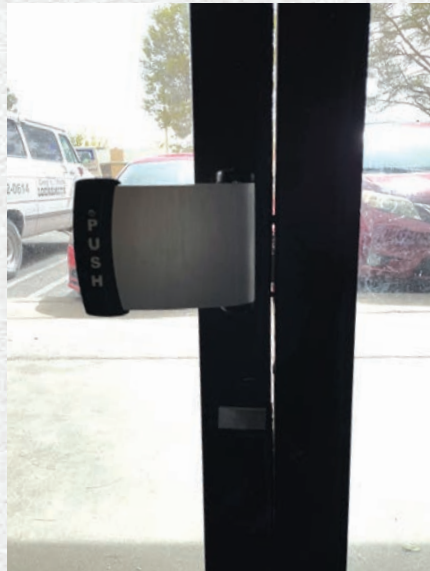
Figure 11. The author installed the mounting bolts and then the lock, and he installed the paddle assembly on the inside.
