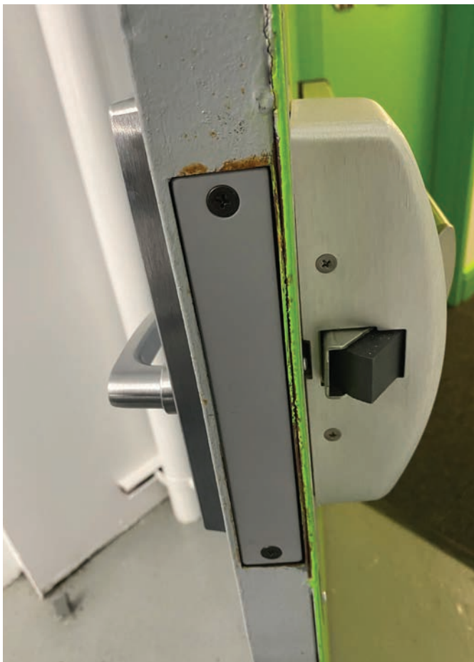
Figure 1. The author used this filler in the mortise cutout.
