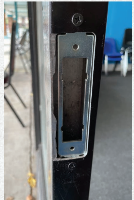
Figure 18. After removing the template, the author drilled the template mounting screw holes to the correct size for the mounting bracket screws and then countersunk the holes for the heads. You can see where the face material is left and where he adjusted to cut the face for the strike.
