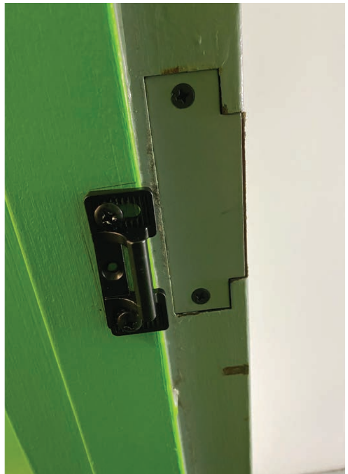
Figure 2. This is the filler for the old strike.
