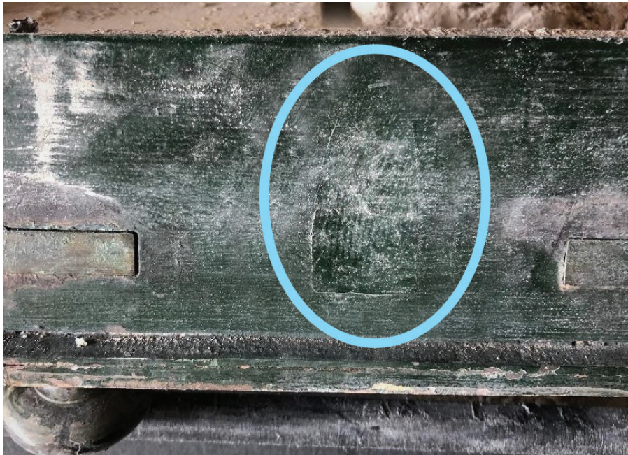
Figure 13. The solid rivets are hidden.
