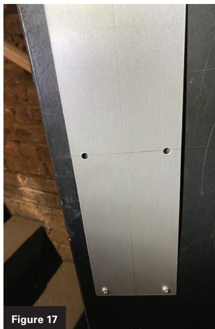
Figures 16-18. These images show the old prep on the inside of the door, the push plate installed and the holes drilled for the head of the bar.
