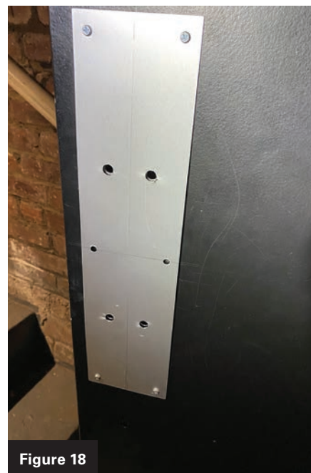
Figures 16-18. These images show the old prep on the inside of the door, the push plate installed and the holes drilled for the head of the bar.
