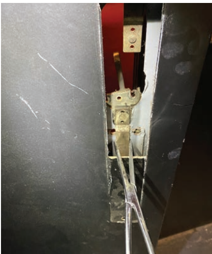
Figure 9. The author's forceps are holding up the bottom rod from the outside. Notice the the size of old prep, which the new bar isn't going to cover. A caveat: Avoid bumping the forceps and jarring them loose.
