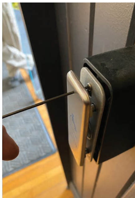
Figure 24. This Allen wrench is inserted through an access hole to loosen one of the two screws that hold on the button.
