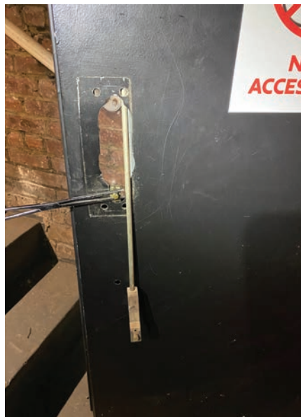
Figure 10. The author has changed position of the forceps so he can pull down the top rod and latch.
