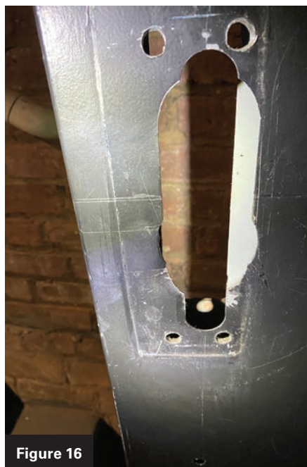
Figures 16-18. These images show the old prep on the inside of the door, the push plate installed and the holes drilled for the head of the bar.
