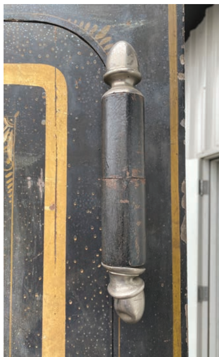
Figure 3. The top hinge and acorns are shown.
