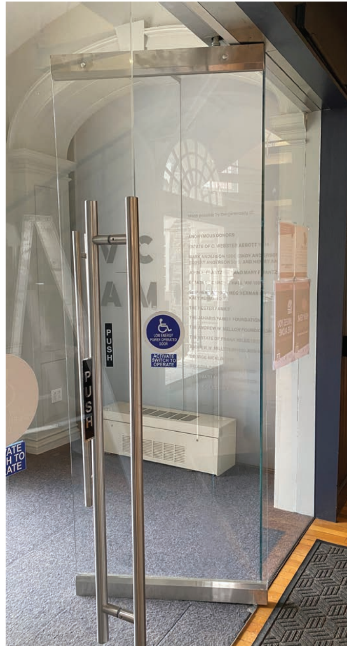
Figure 20. This glass door wouldn't close properly.
