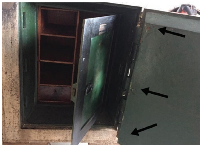
Figure 4. The interior and the back cover screw locations are shown.
