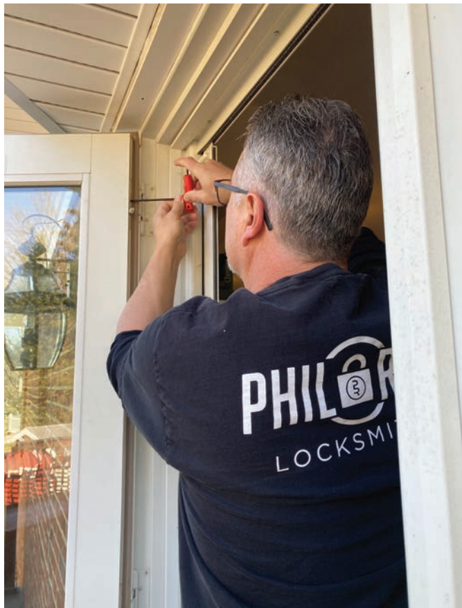
Figure 15. Turn the Allen wrench counterclockwise to decrease the space between the door and the side jamb on the top hinge.
