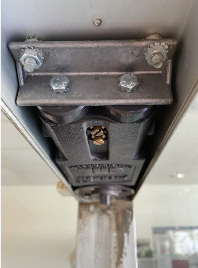
Figure 20. Here are the two bolts that need to be removed to drop the closer. Most of the time, the closer needs a little coaxing by using a screwdriver as a small pry bar to remove it from the opening.
