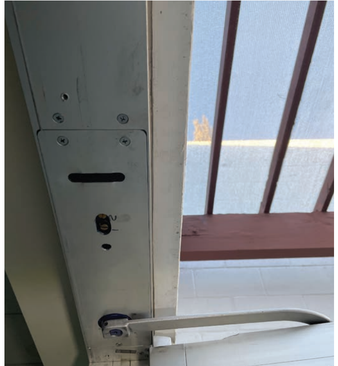
Figure 25. The offset arm version is the same closer body, but it does mount in a slightly different location in the header. This one has screws to hold the cover in place.
