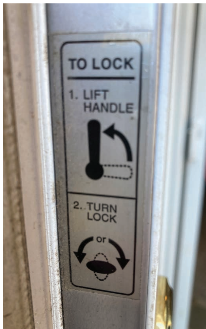
Figure 2. To lock the door, the interior door handle or exterior door handle on the active door must be lifted.
