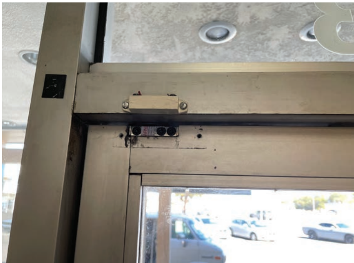
Figure 4. Here are the three arm-clamping block screws to be removed. The older screws use a different-size hex key than the current Jackson closers. Once the screws are removed, the door can be pushed out. Use great care to catch the door. I often go outside and pull on the door if it doesn't come free, and then I keep a hand on the latch edge and typically use a rubber mallet to tap on the frame of the door at the arm. Once the door is free, tilt it away from the frame and lift it off the bottom pivot. The door can now be laid down on its latch edge in a safe location to replace the arm and, if needed, the bottom pivot. You can also open the door and tilt it into the opening to remove the door. Hold-open closers are easy to hold in this position. When dealing with non-hold-open closers, shut or tighten the closing speed valve to hold it in position. Be careful not to overtighten the valve and damage the valve seat. Occasionally, you may need a pry bar to lift the door off the bottom pivot, so be prepared with one. I typically have my cart with all the tools I may need, including a prybar within reach anytime I remove a door.
