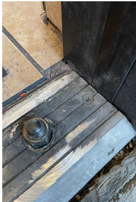
Figure 13. This one was loose and wearing a hole through the threshold. You'll see in the next photo why I was called to work on the door.
