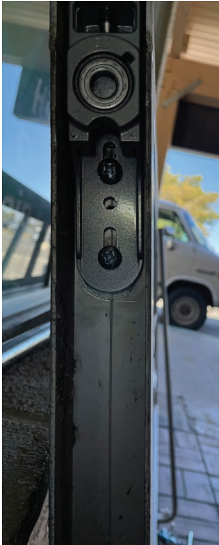
Figure 11. Before moving to the closer body, it's best to replace the bottom pivot, as it takes most of the door's weight. Be sure to mark the location with a scribe before replacing it. Sometimes, you'll find a different pivot or that the existing one is fine and doesn't need to be replaced.
