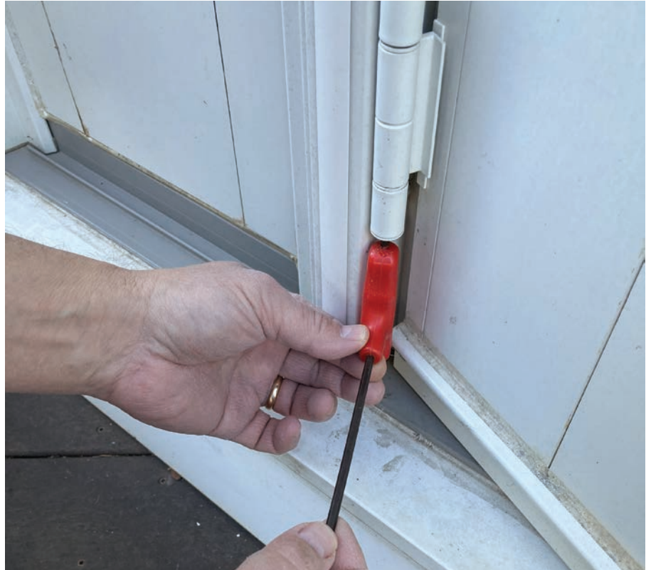
Figure 18. The author inserted the \frac{5}{32} " Allen wrench into the bottom of the bottom hinge to begin the vertical adjustment.
