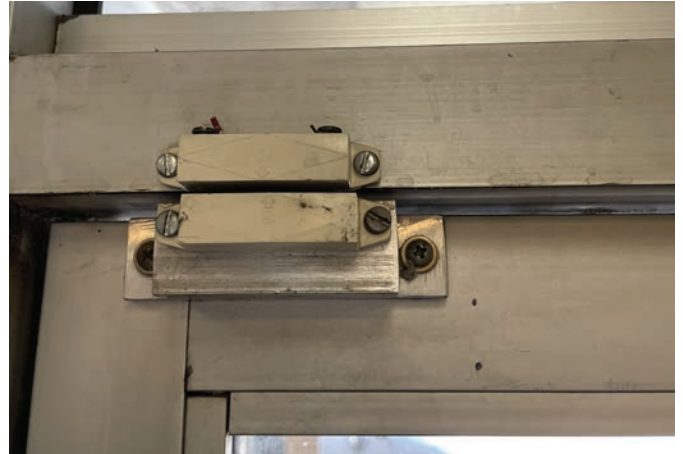
Figure 2. This door has an alarm contact magnet mounted over the top of the arm screws. It needed to be removed to access the screws.
