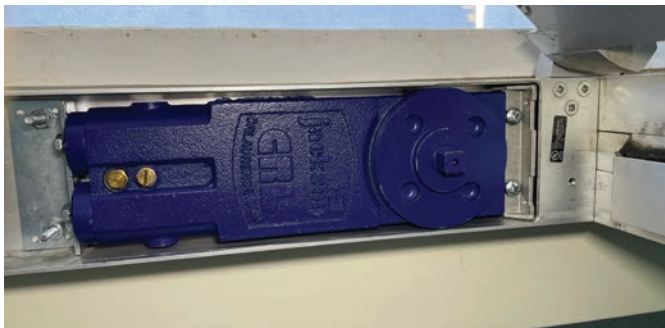
Figure 26. I replaced the closer body with an adjustable-size body. The adjustable bodies are painted blue. One thing I dislike about the adjustable bodies is the cover plate must be removed to adjust the spring tension.
