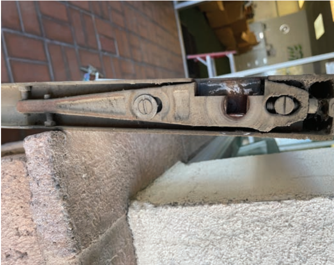
Figure 5. Once the door is out of the opening, it can be laid down on the latch edge to make it easier to work on as you replace the arm and possibly the bottom pivot. Remove the holding screw that locks the arm to the door, loosen at least one of the two hex head bolts called centering screws and then remove the top centering adjustment screw at the end of the arm. This screw adjusts the door horizontally in the opening.
