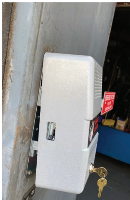
Figure 26. The author has fitted the flange into the slot at the top of the mounting plate.
