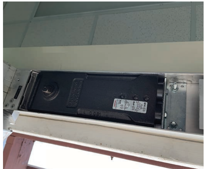
Figure 23. This is an International door closer in a different header. Installing the closer is the reverse of taking it out. I typically loosely install the two screws with lock washers.
