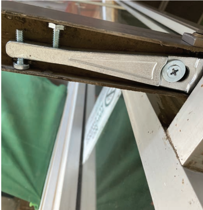
Figure 24. The arm adjusts the door center position with these two bolts. The arm has a screw on the end that we saw in Figure 5 to adjust the horizontal position in the opening. Once these are all adjusted, tighten the Phillips-head screw to hold everything in position.
