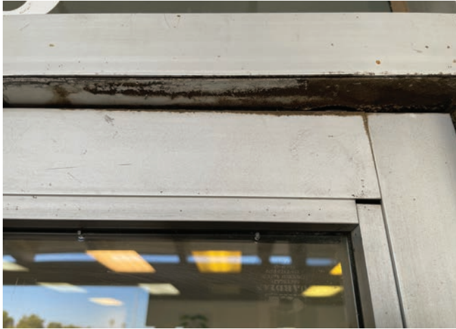
Figure 1. Oily dirt on the bottom side of the cover plate is an open opportunity for a sale on this center-hung door closer.
