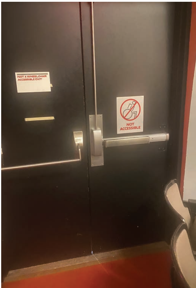
Figure 1. The panic bar without the bottom rod is semi-finished.
