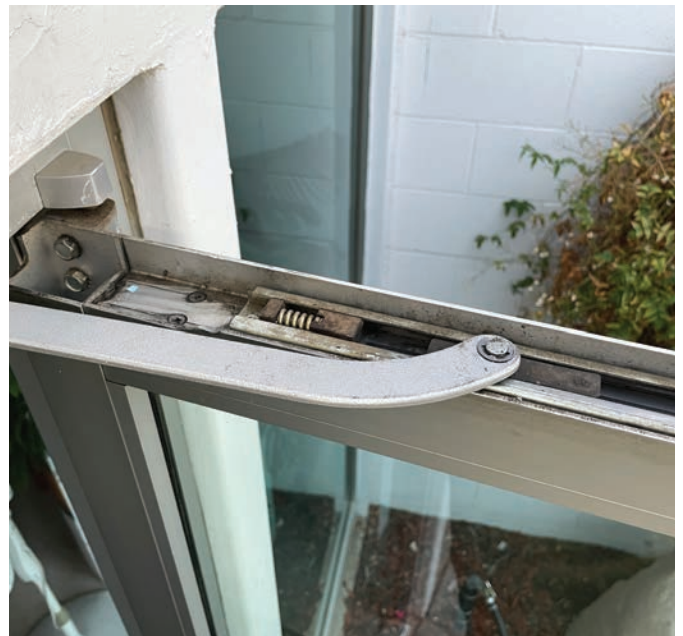
Figure 27. The offset arm connects to a track that has a sliding bolt. When changing the closer, you need to remove the C-clip to disconnect the arm. The older ones used to have a smaller axle or shaft through the plastic slide block. These would often break, and the arm would slip off. The next step is to loosen the socket head cap screw that clamps the arm onto the spindle. The rest of the replacement is the same as the center-hung version. 🛠️
