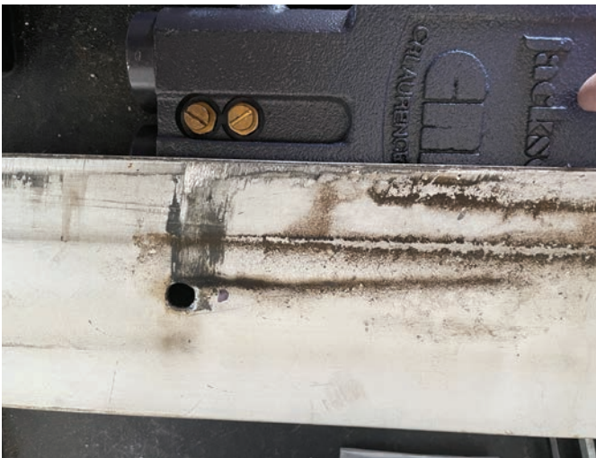
Figure 22. The older closers had a single adjustment valve screw for both the sweep and latch speeds. The closer speed changes with full turns, and the latch speed is adjusted by turning it partially. If you are replacing an older closer, you'll need to add a second and maybe a third hole.
