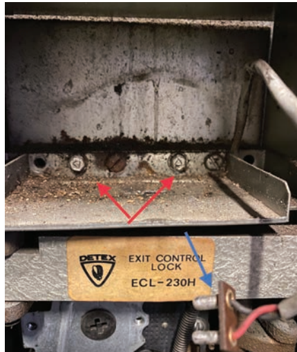
Figure 4. The red arrows point to the hex-head self-drilling screws that attached the top of the DETEX body to the door. The blue arrow points to what was plugged into the battery.
