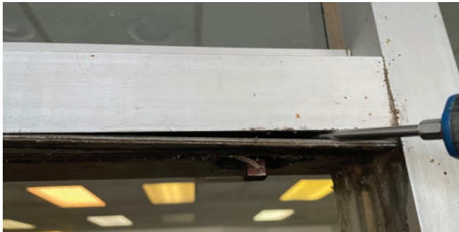
Figure 17. Once the arms and pivots are replaced, it's time to install the new closer. This starts with removing the snap-in cover. Sometimes the cover will extend the full length of the opening, but most often I find them with a split cover. Use a small screwdriver to spread the header away from the snap in the cover and gently pry it down along its length.
