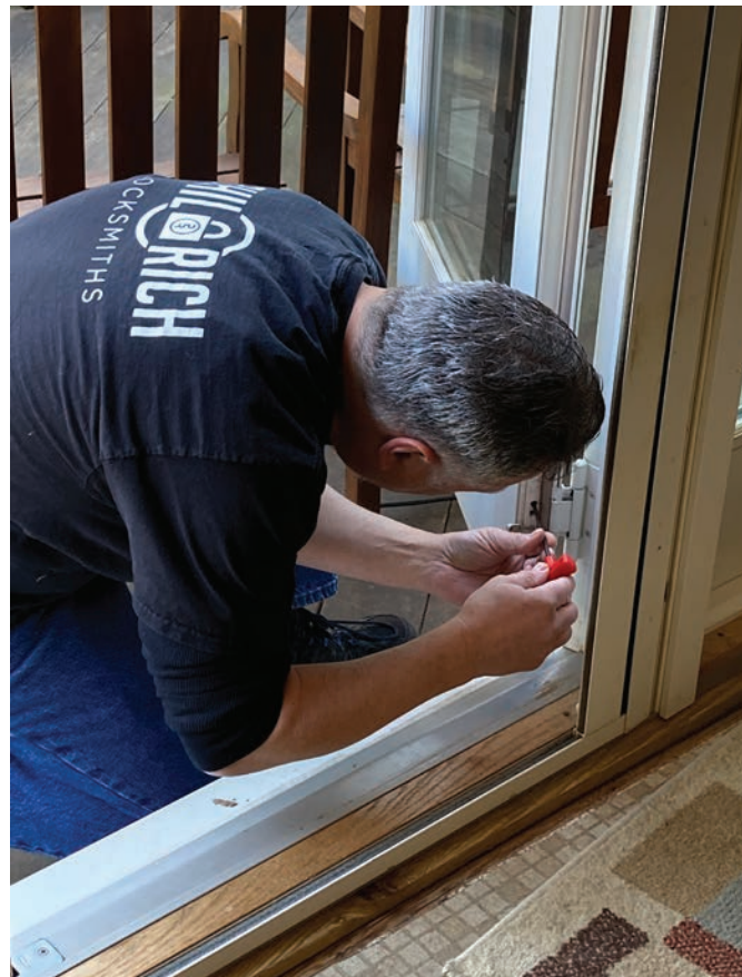
Figure 16. The author is making the horizontal adjustment on the bottom hinge.
