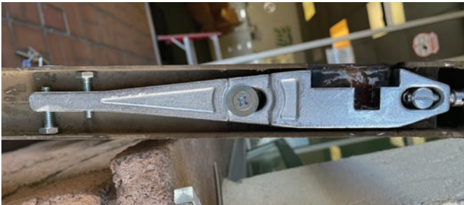
Figure 7. I highly recommend installing a new arm with the closer. It only takes a few minutes, and the arm normally comes with the closer. Before removing the old arm, use a scratch awl to mark the location of the arm. Although you'll adjust it after reinstalling the door, this provides a great starting location.
