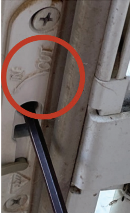
Figure 17. If the gap is too tight, turn the Allen wrench clockwise to increase the space between the door and the side jamb. You can see the words “IN” (counterclockwise) and “OUT” (clockwise) with a directional arrow here.
