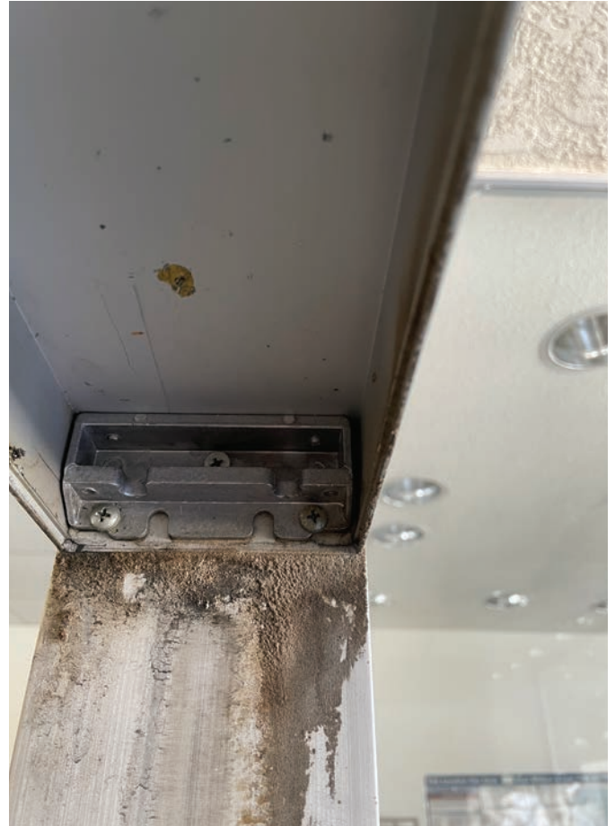
Figure 21. Be sure to check these three screws that hold the bracket to the frame rail while the closer body is out of the header.
