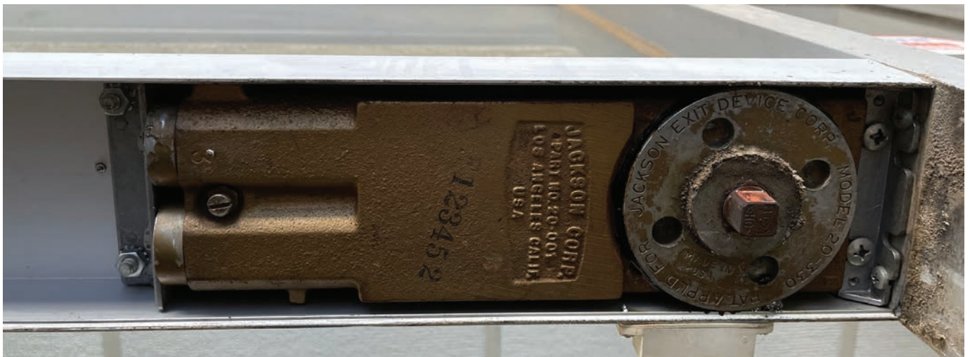
Figure 19. There are two screws that need to be loosened or removed prior to taking out the bolts on the other end.
