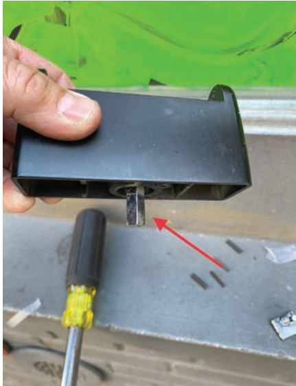
Figure 8. The red arrow points to the spindle, which projects into a cam in the lock.
