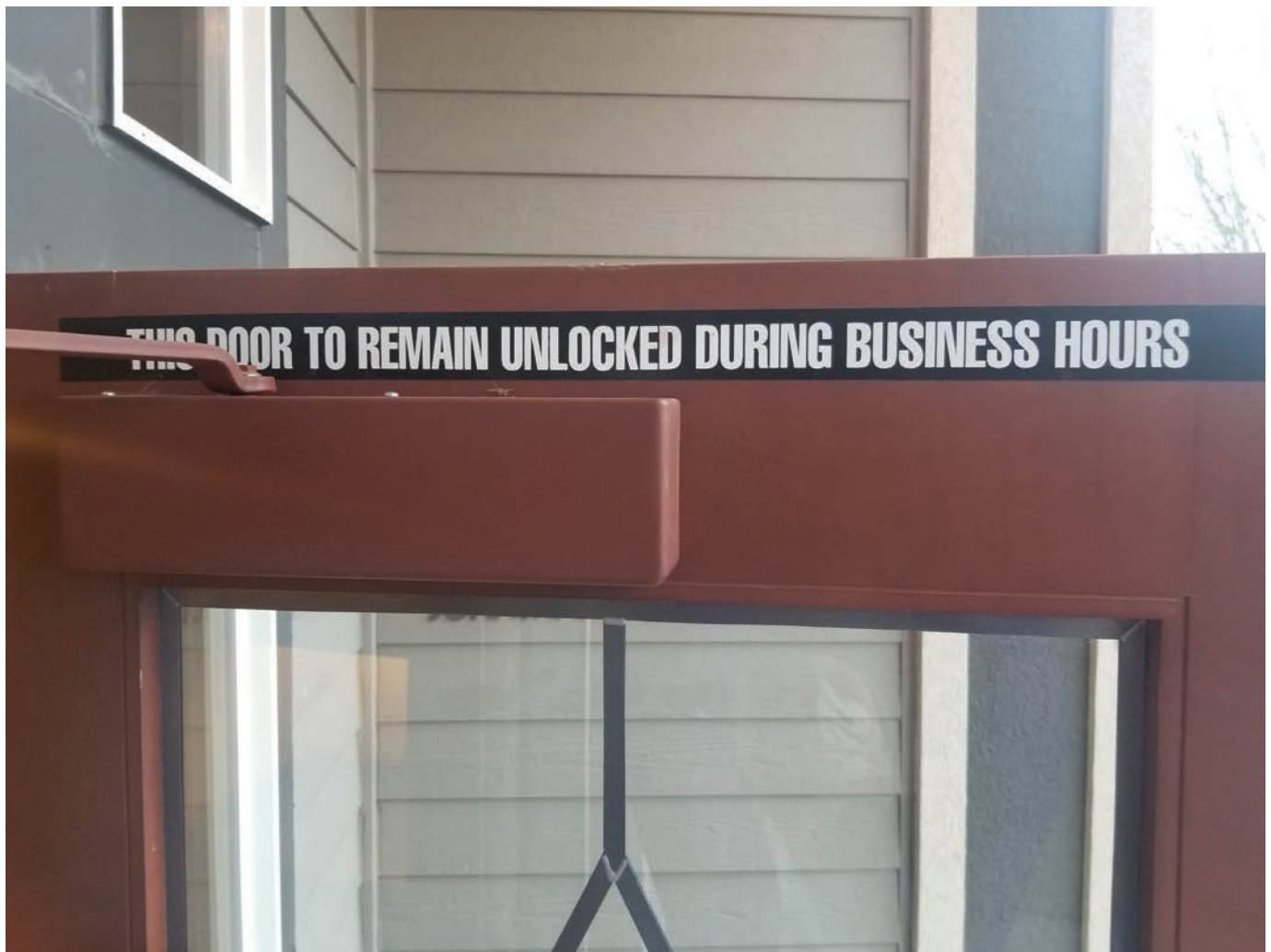
Figure 5. Code allows an emergency exit to have a double-cylinder deadbolt on the main entrance of a business only with the approval of the AHJ — and if there is a sign above the door stating: “This door to remain unlocked during business hours” (or similar wording).
