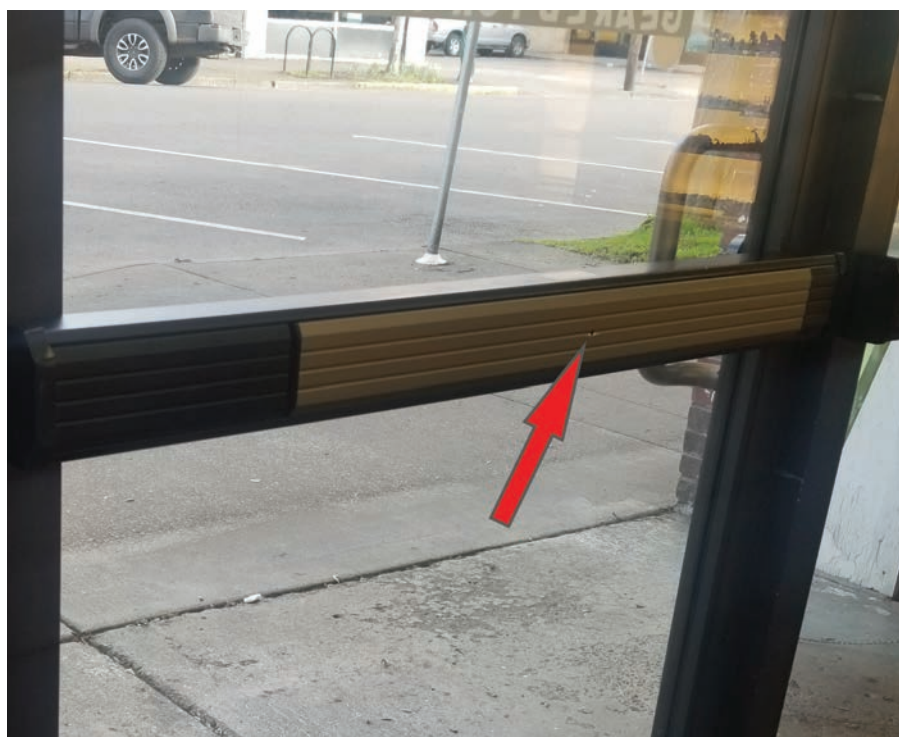
Figure 6. This exit device has a dogging feature. While allowed on some emergency exits, dogging is not allowed on fire-rated doors.
