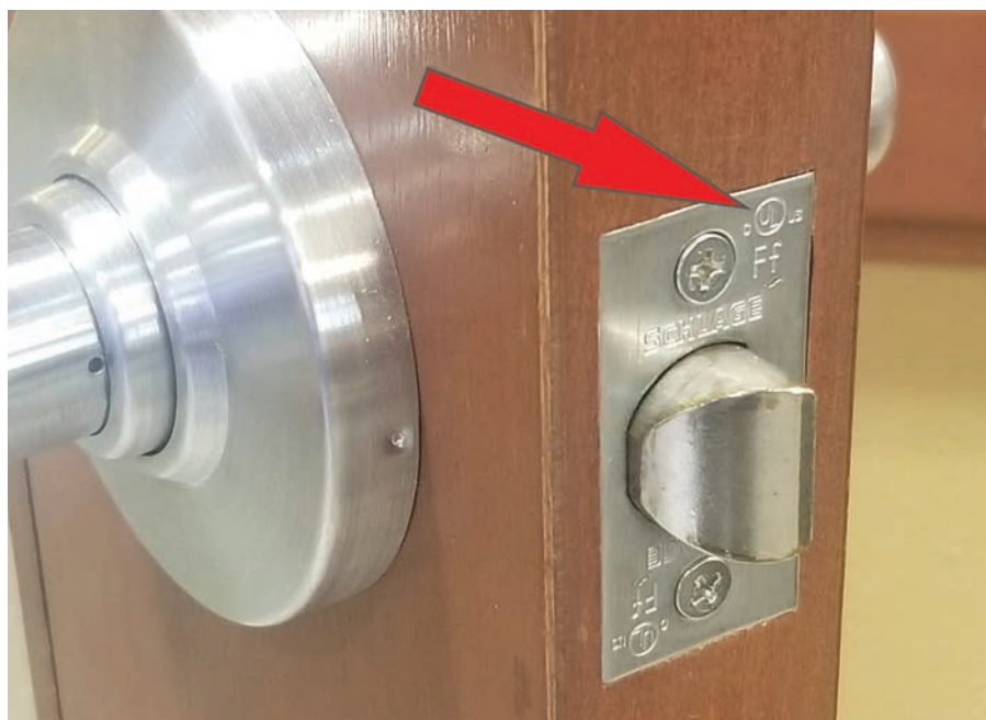
Figure 3. This fire-rated latch is marked with the UL logo.
