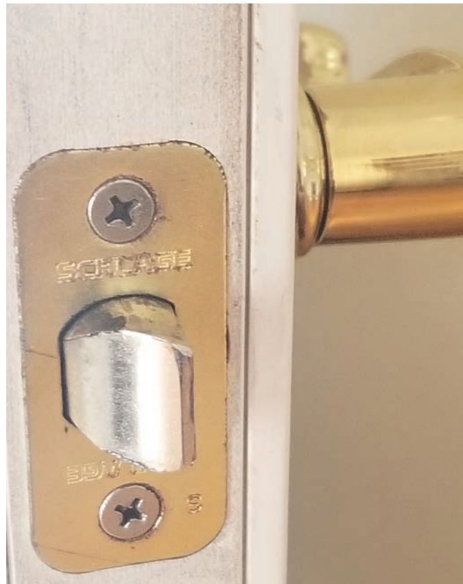
Figure 2. This is a non-fire-rated latch. Be sure all components on a fire door are fire rated.
