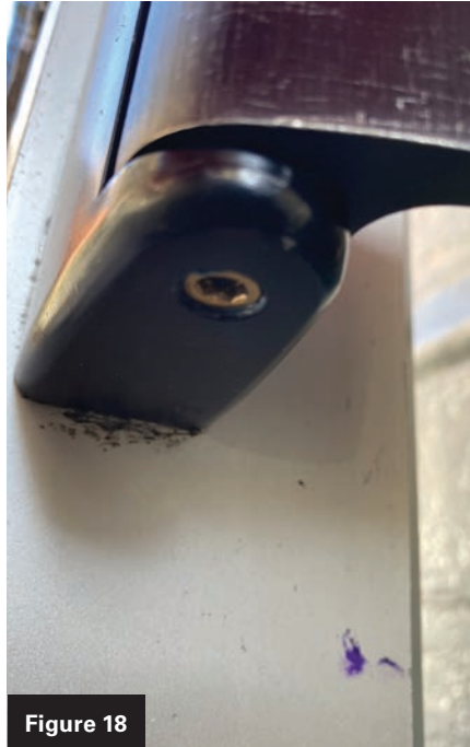
Figures 17 and 18. The set screw is started and then all the way in.
