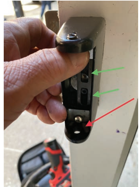
Figure 13. The red arrow is pointing to another set screw hole at the bottom of the escutcheon.
