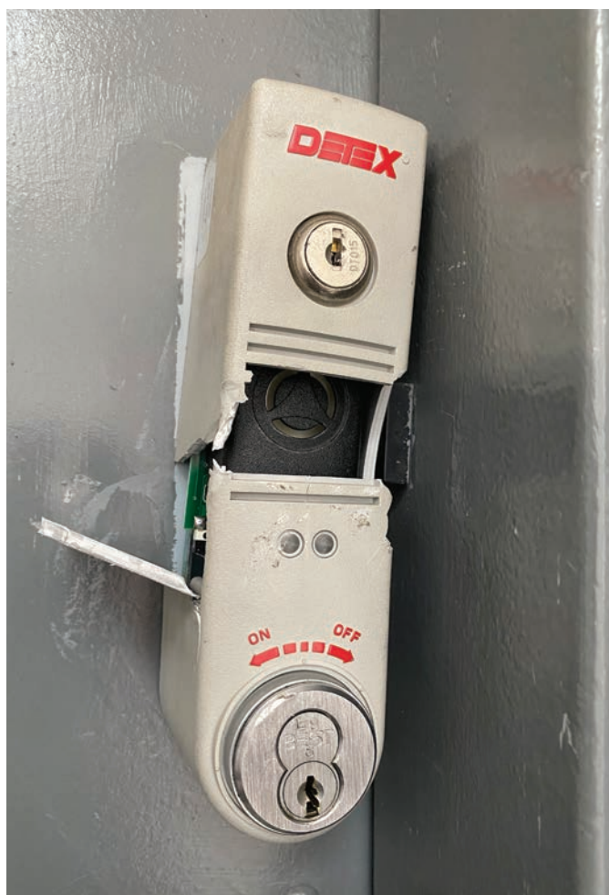
Figure 3. The firefighters smashed this DETEX alarm.
