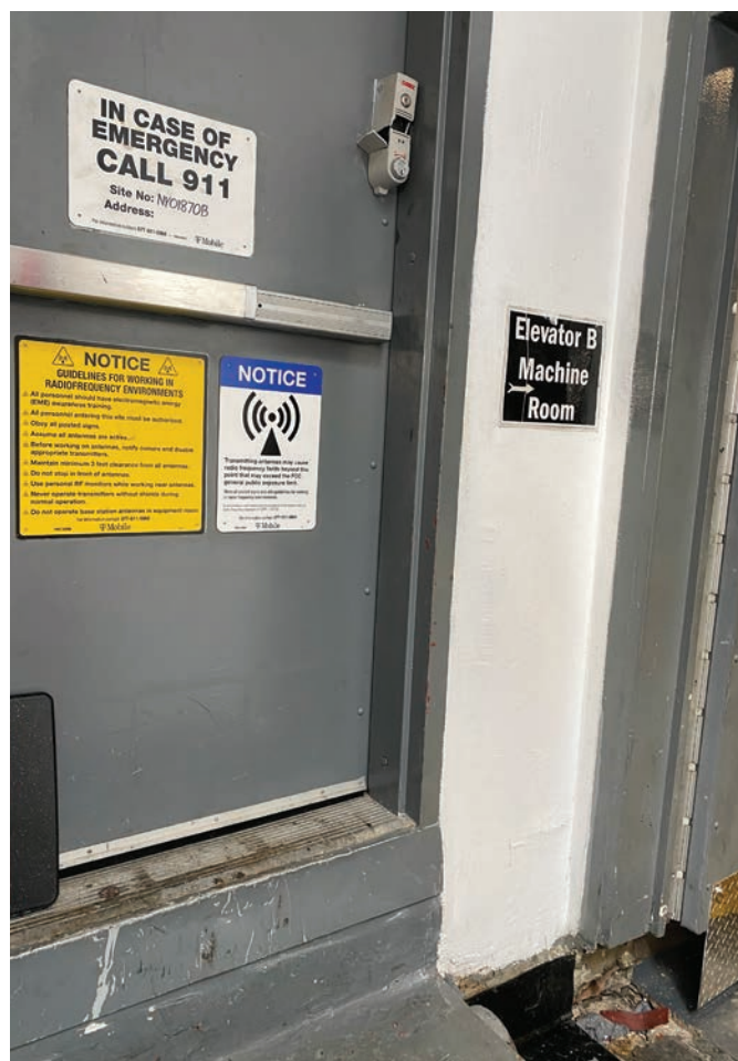
Figure 4. The DETEX is mounted on the hinge side rather than the lock side of the door.
