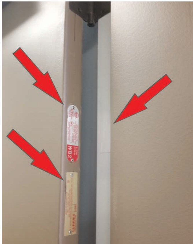
Figure 1. This fire-rated door has two labels on the door plus one on the frame (painted over).
