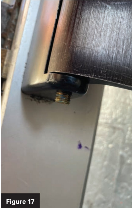
Figures 17 and 18. The set screw is started and then all the way in.
