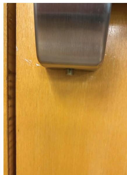
Figure 16. The cover is on, and you can see the threaded part hanging down through the cover.
