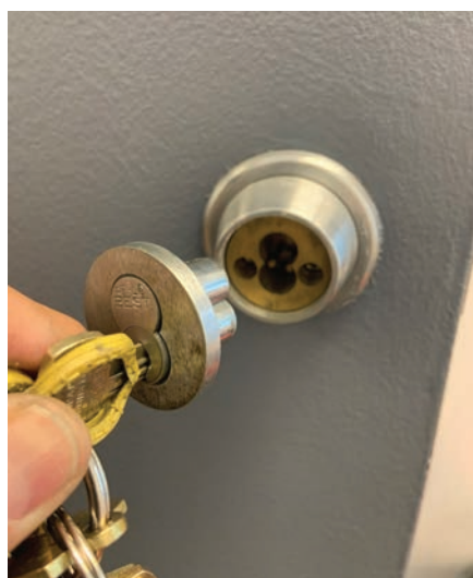
Figure 8. The author is using the control key to remove the outside core, along with the plate around it.
