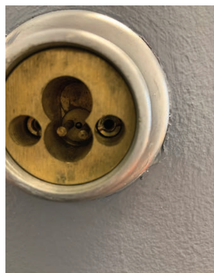
Figure 9. You can see the two screws that attach the outside of the lock to the inside.
