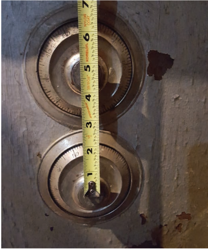
Figure 4. Both dials on the front door are at 4½" on center.
