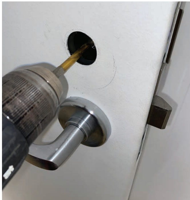
Figure 9. The disc is being used as a guide for drilling the pilot hole.
