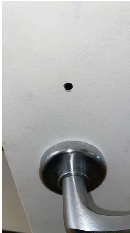
Figure 11. You can see the pilot hole on the back side of the door.
