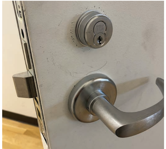
Figure 15. The new cylinder is in place.
