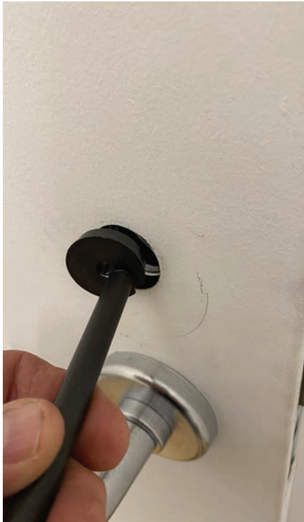
Figure 10. After screwing the threaded rod back in, loosen the clamp and remove the disc.
