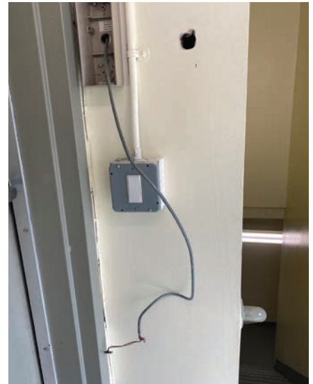
Figure 7. The wire is hanging out of the old DETEX.
