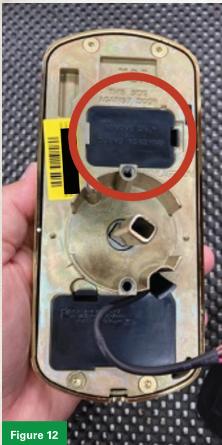
Figures 12 and 13. The solid cover plate hides the cylinder from view and is embossed with "REMOVE ONLY DURING RE-KEYING."
