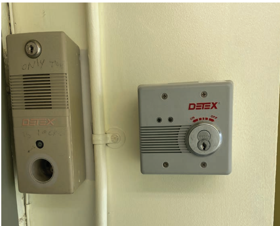
Figure 1. The new conduit wouldn’t fit in the original one’s space.
