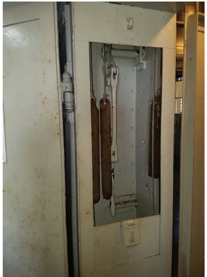
Figure 10. Here's the counter-weighted lever for the sliding door to release inmates.
