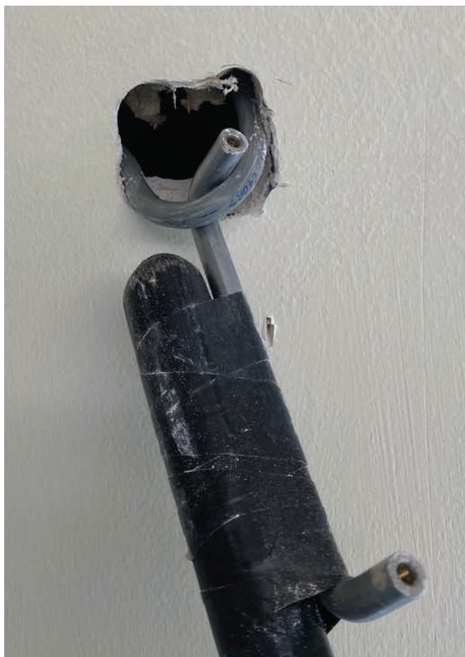
Figure 9. The snagged wire is coming through the hole.
