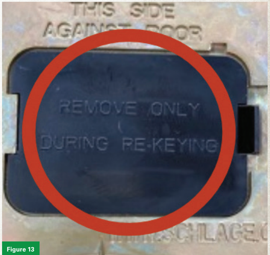
Figures 12 and 13. The solid cover plate hides the cylinder from view and is embossed with "REMOVE ONLY DURING RE-KEYING."
