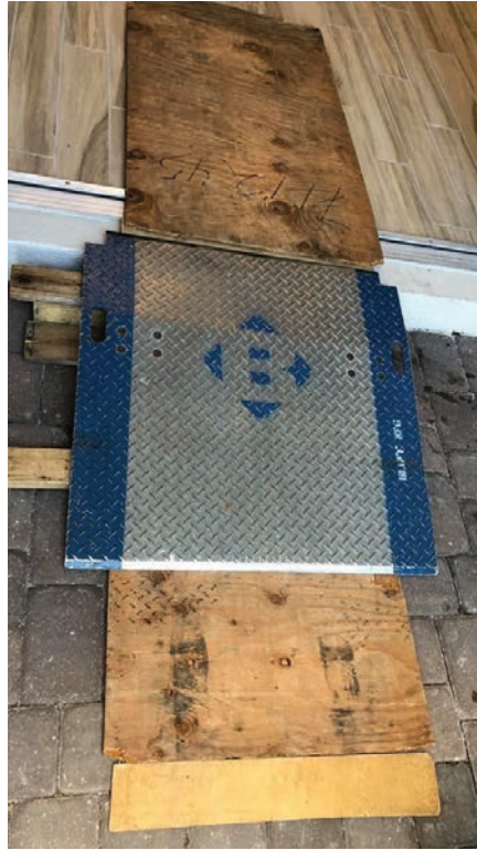
Figure 6. The ramp for the step up into the house was about 6" in elevation.
