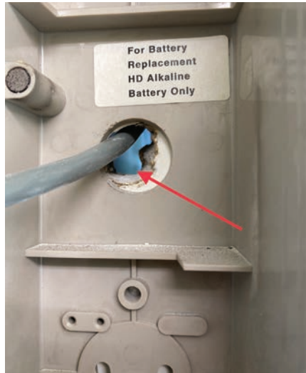
Figure 6. You can see the light from the flashlight within the void behind the old alarm.
