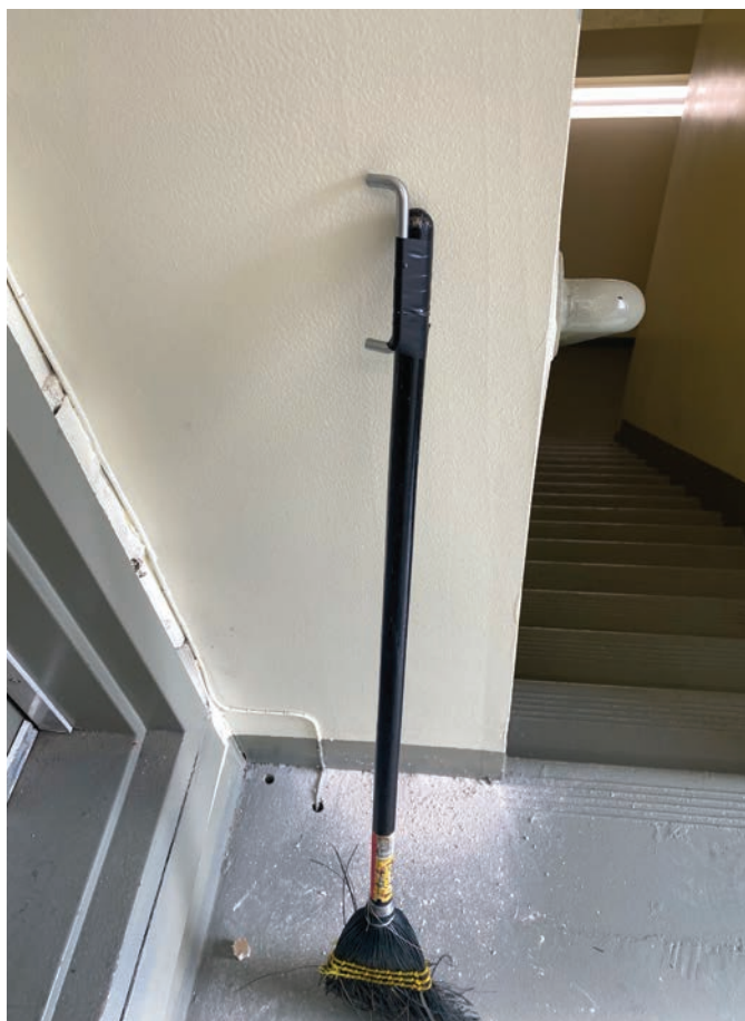
Figure 8. The author improvised by making this tool to pull the wire through the hole.
