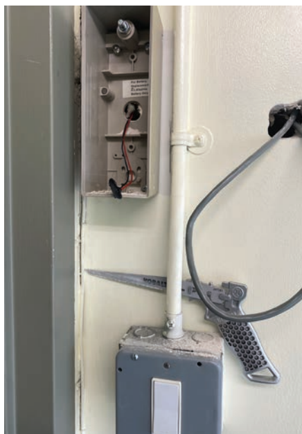
Figure 10. Most of the wire is now pulled through.
