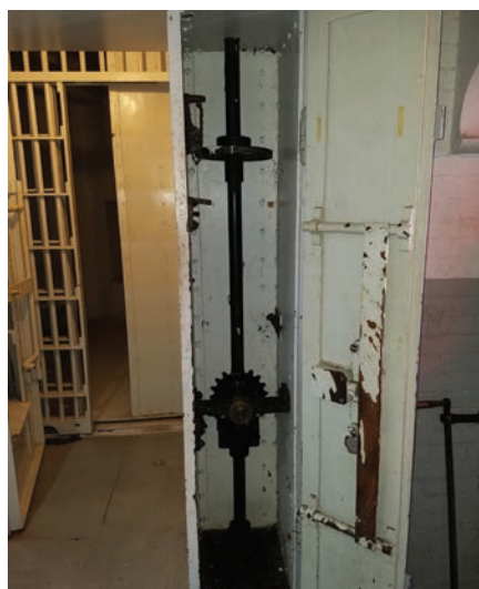
Figure 5. The smaller door holds the larger door shut and houses the turning mechanism.
