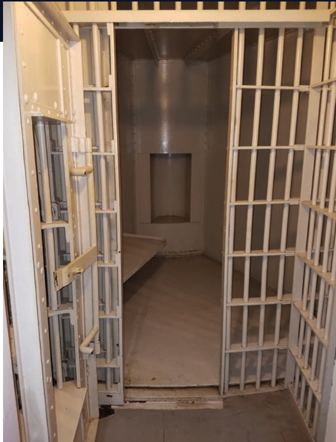
Figure 11. This is the entrance to a cell. Note the track on the floor to guide the sliding door.
