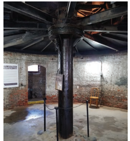
Figure 17. The hollow central pipe supports the cell block, flushes waste and provides ventilation.
