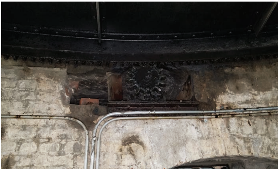
Figure 16. The gear mates with the circular rack to turn the rotary jail.
