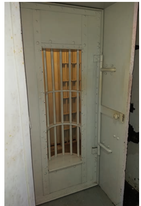
Figure 13. The barred door is locked with a pin in the gear control box.
