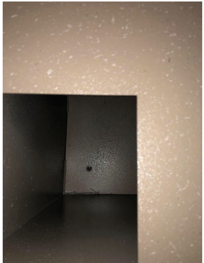
Figure 4. The anchor holes are visible in the bottom of the pedestal.
