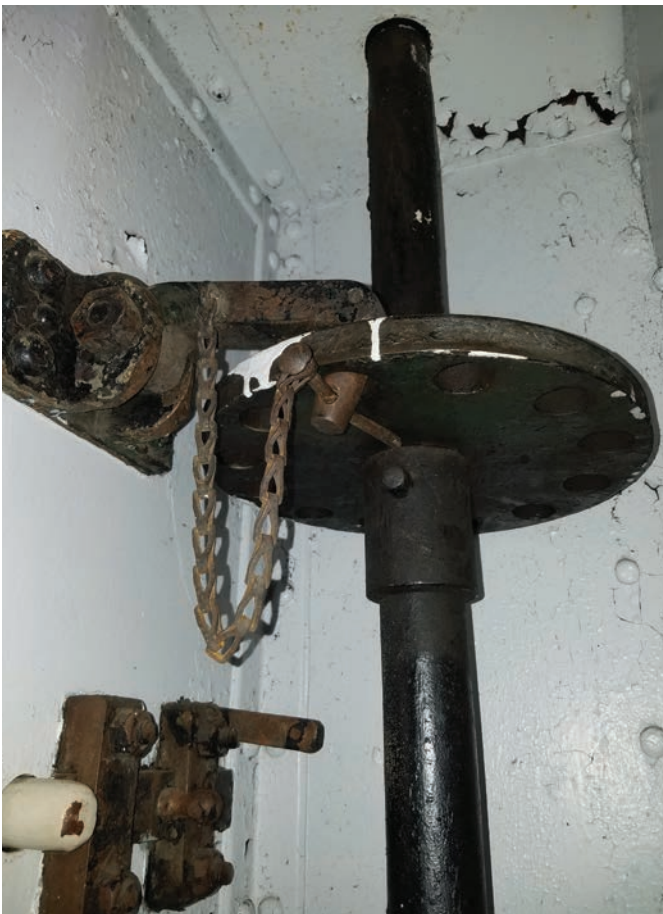
Figure 9. The rotational shaft is pinned to prevent unauthorized rotation.
