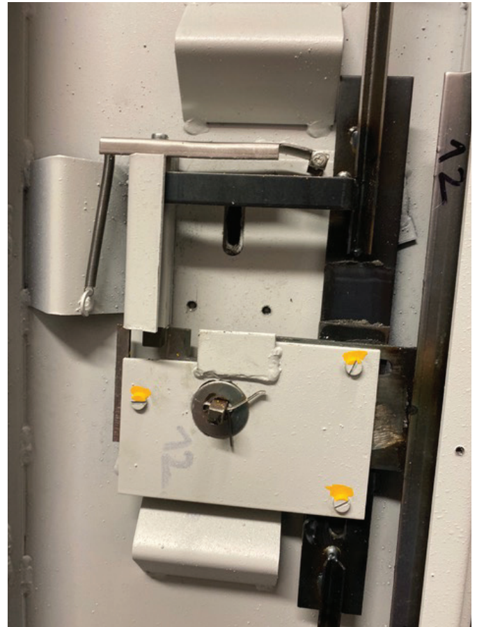
Figure 15. The lock has been removed.
