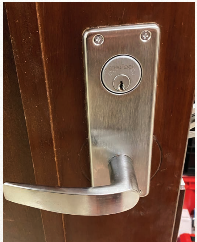
Figure 10. You can see the finished product from inside the courtroom. The existing Medeco cylinders were reused.
