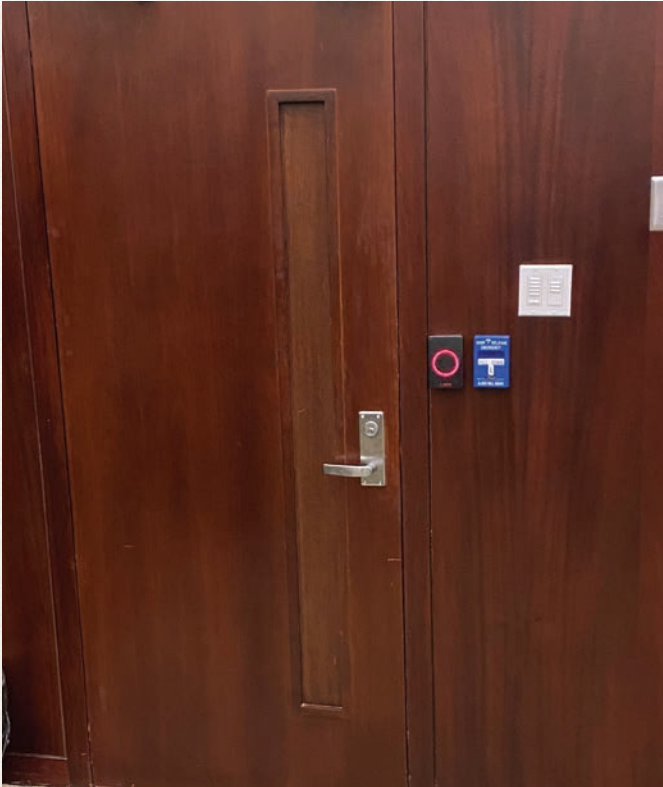
Figure 5. This is the door that had a window. Well, it used to be a window, but for core drilling, it was just like a window. The author had to go up and over at top of door, then back down to hinge transfer.
