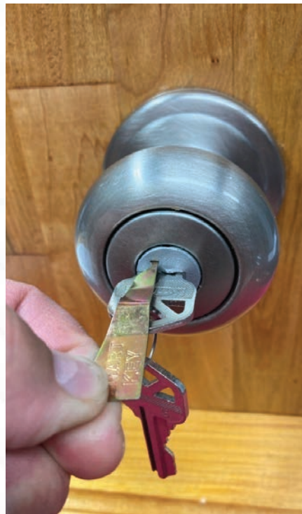
Figure 4. Insert the SmartKey learn tool into the small hole above the cylinder.
