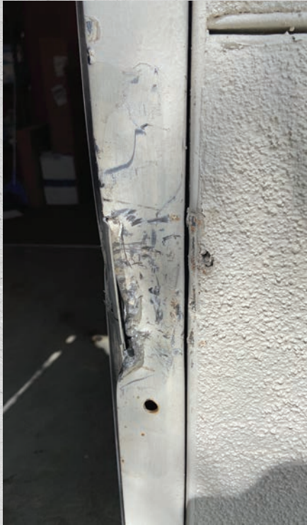
Figure 7. It might not look pretty on the face, but the strike is sitting in the correct location to secure the door.
