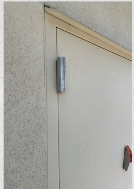
Figure 12. The author used a hinge doctor to move the door over and to make it tighter on the hinge side. Normally, these are used to bend the top hinge a little to bring the door back. In this case, it was used on all three hinges to move the entire door over.
