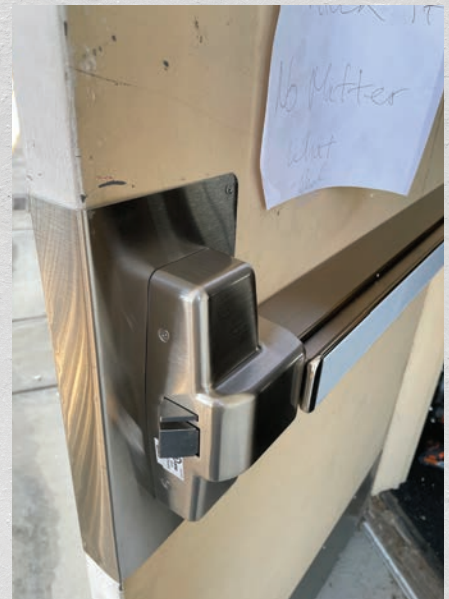
Figure 18. The cover is installed, and one last operation test was conducted to ensure nothing had moved.
