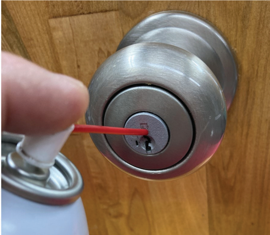
Figure 1. I like to generously lubricate the cylinder. I have had success using Houdini, but I am sure other lubricants would work well, too; we all have our favorites. Use whatever you are comfortable with.
