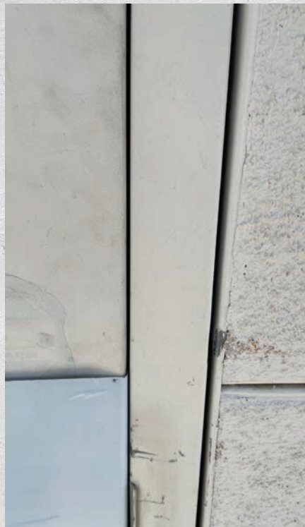
Figure 11. The addition of a wraparound plate left very little room between the door and the jamb.
