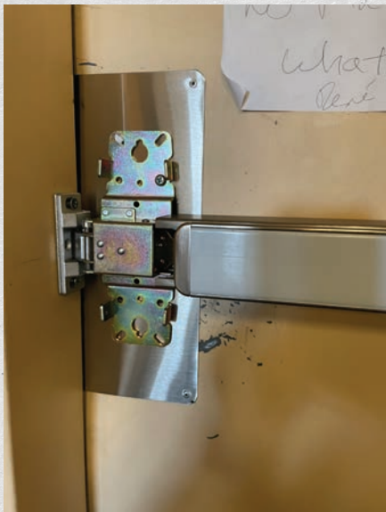
Figure 16. The rim cylinder was installed, and the panic bar mounted with the single screw. Once operation was tested, the second screw in the strike was installed.
