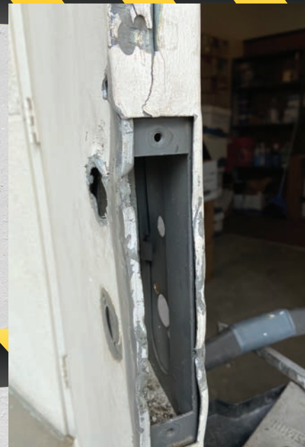
Figure 3. The door looks better and accepted the mortise lock case, but the integrity of the door was severely compromised. Keep in mind that these are temporary repairs until a new door and frame can be procured and installed. Functional is more important than pretty.
