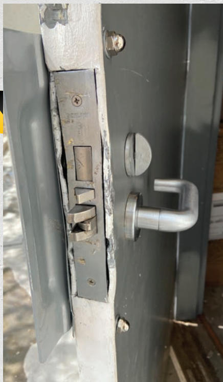
Figure 4. The mortise lock is reinstalled and functions. It is far from perfect, but works.
