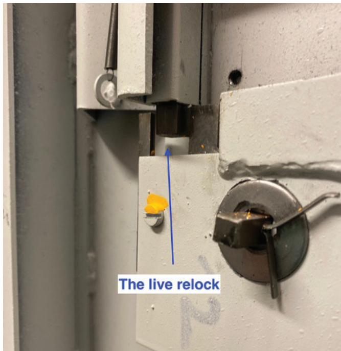
Figure 16. The live relock is shown.
