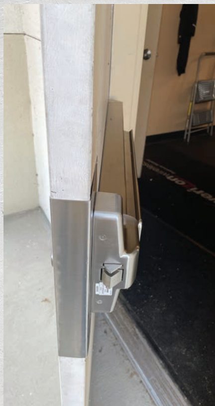
Figure 23. The wraparound plate covers the mortise pocket and provides a nice finished door edge.
