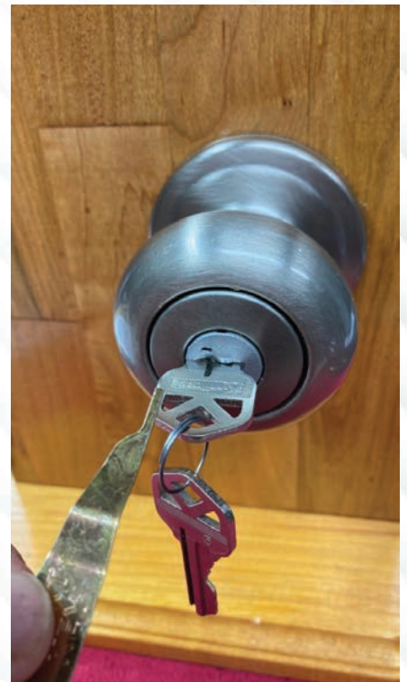
Figure 5. Remove the SmartKey learn tool.
