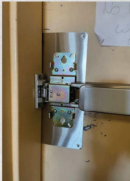
Figure 17. The rest of the center case holes were drilled, and the screws for it were installed.
