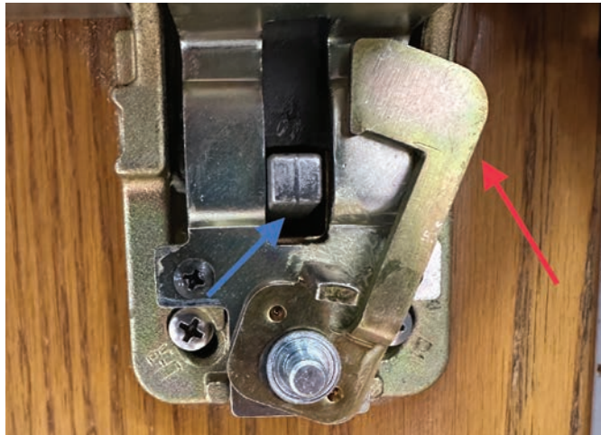
Figure 20. You can see how the internal parts on the head of the panic bar lock the outside trim.
