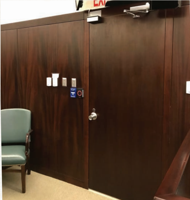
Figure 3. This image provides a full pre-conversion view of the door with the mag lock that needed to go away.
