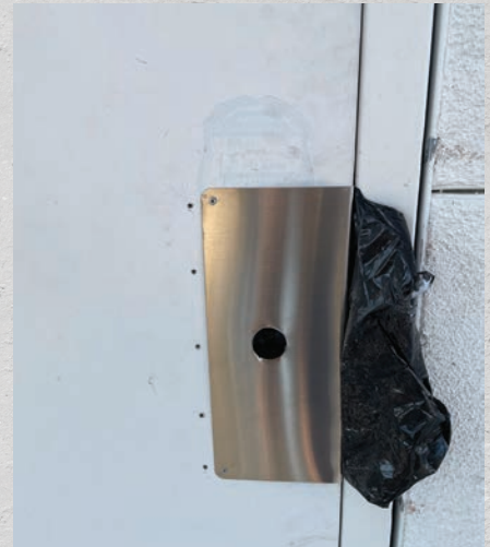
Figure 15. Now that the cylinder hole and one screw hole to mount the device are drilled, the plastic protective film can be removed.
