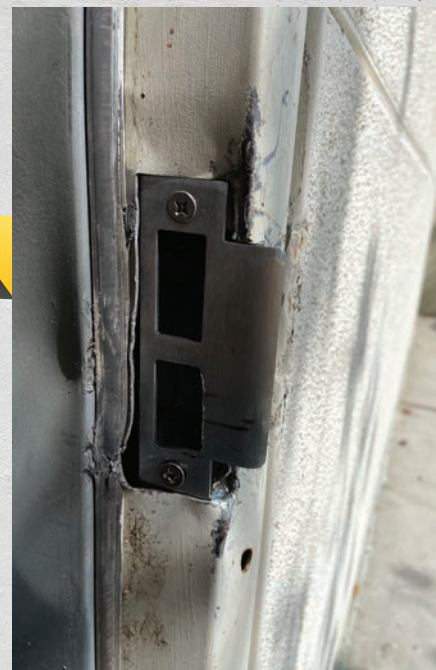
Figure 6. The problem with the strike side is that it is difficult to get behind it or inside the frame without removing the frame. The author bent it back with a prybar and locking pliers. Again, this only needed to work until it could be repaired.
