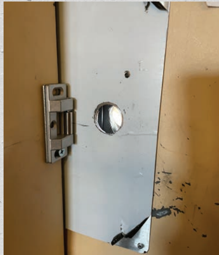
Figure 14. The author's preference is to only drill a single screw hole to ensure proper alignment with the strike and the cylinder hole.
