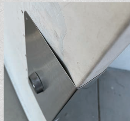
Figure 21. The door was caved in a little from the attempted break-in. I debated trying to cave in the plate or bend it back out from the inside but decided it was not bad enough to worry about. The cylinder is protected with a hard collar typically used with mortise cylinders. This provides better protection than the typical sheet-metal trim ring included with rim cylinders.
