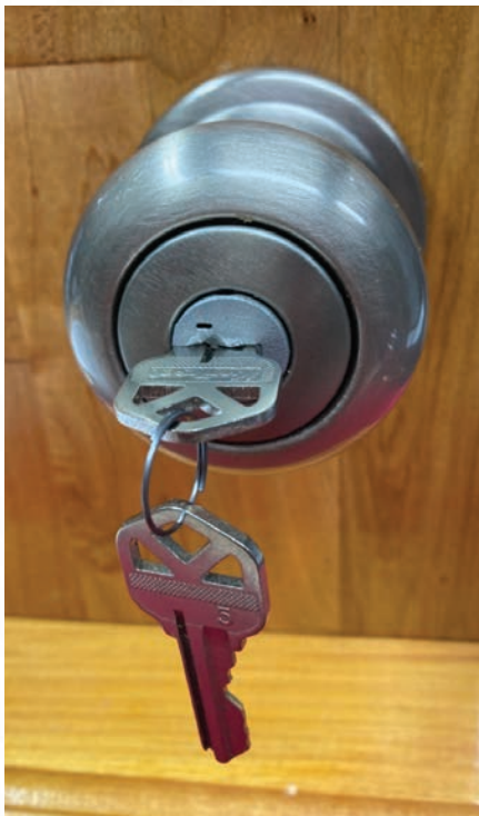
Figure 3. Turn the key \frac{1}{4} turn clockwise to the 3 o'clock position.
