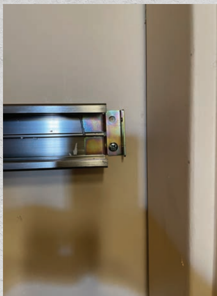
Figure 19. The end cap bracket screws need to be drilled. Use a level, but also look at the door and frame. Close the door and make sure it looks correct. It is rare, but sometimes it looks better to be a little off level if the jamb is off of plumb.
