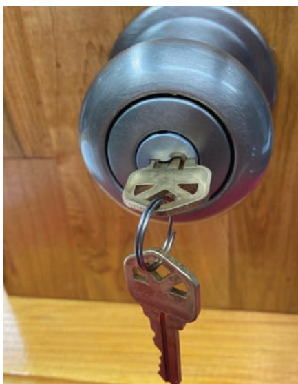
Figure 8. Turn the key counterclockwise 180 degrees to the 9 o'clock position.
