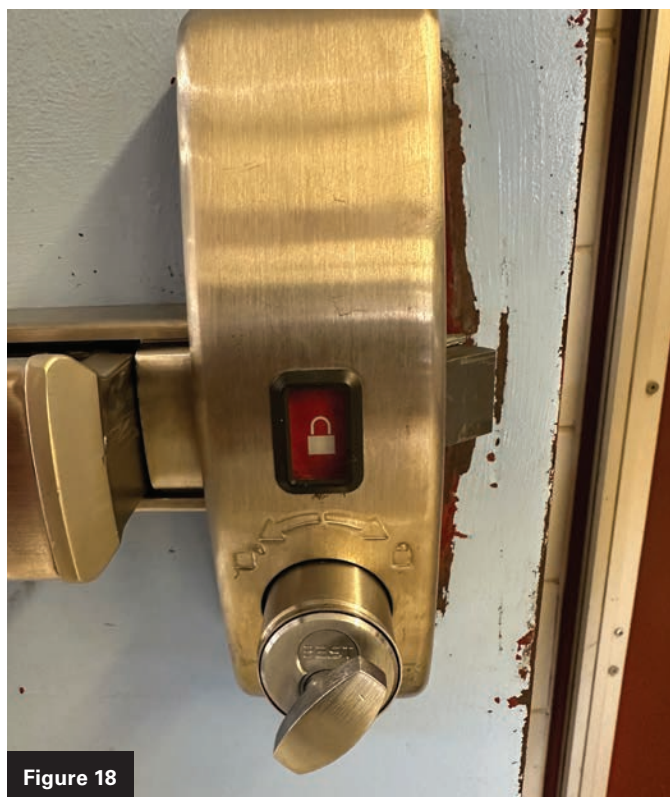
Figures 18 and 19. A PH1 intruder function panic device is shown in the locked and unlocked positions.
