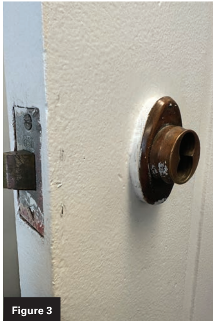
Figures 3-5. A high school had a very old BEST cylindrical deadlatch with a thumbturn.
