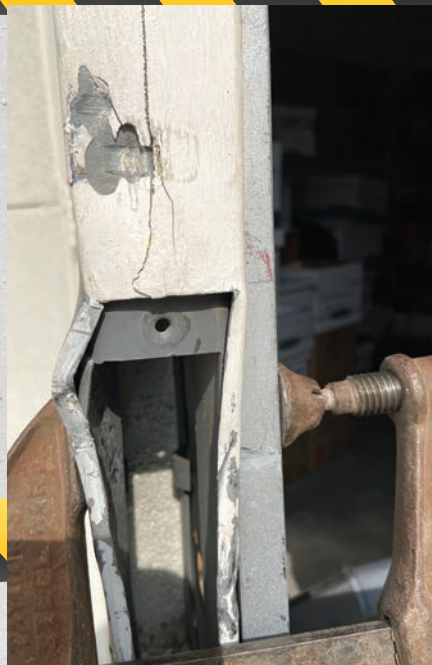
Figure 2. A piece of steel tub was used along with a couple of C-clamps to straighten the door. A hammer added assistance to the clamp. In some cases, you may need to work inside the mortise pocket to reform the door.
