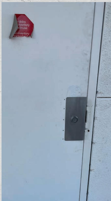
Figure 22. The outside of the door had a line of screws that were not covered by the plate. Sheet metal screws were installed to fill the holes.
