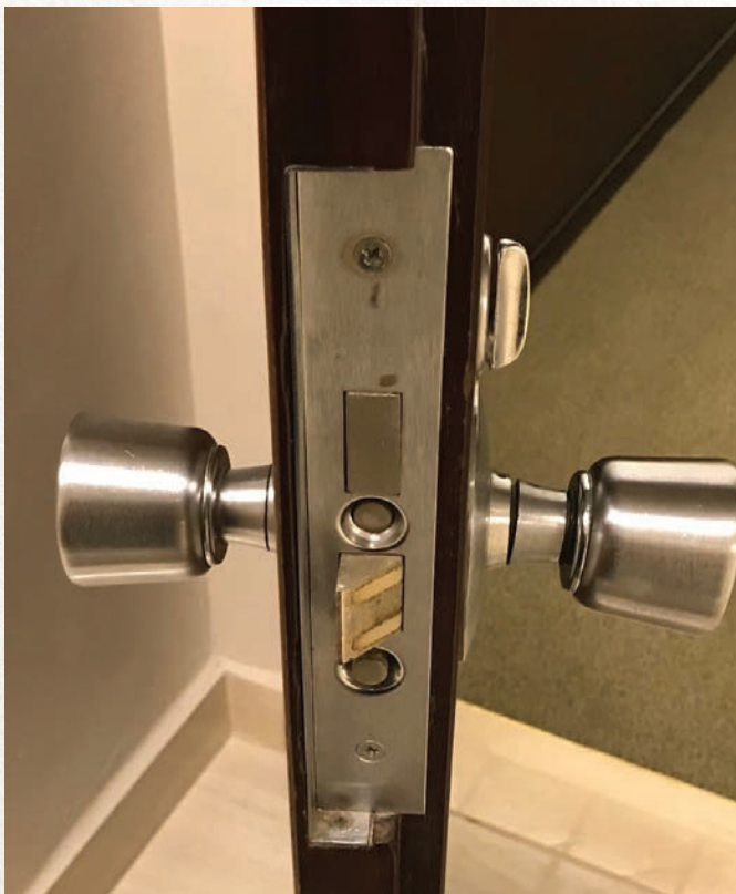
Figure 1. These are the lock and door before the conversion to electric locks. You can see the boot leg or offset on the door.
