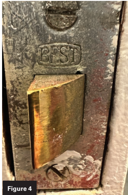
Figures 3-5. A high school had a very old BEST cylindrical deadlatch with a thumbturn.
