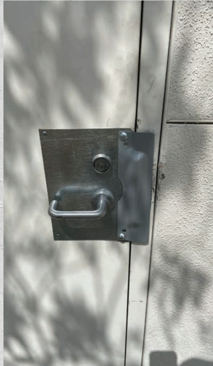
Figure 8. A cover plate made of sheet metal plus a latch guard covered up all the damage.
