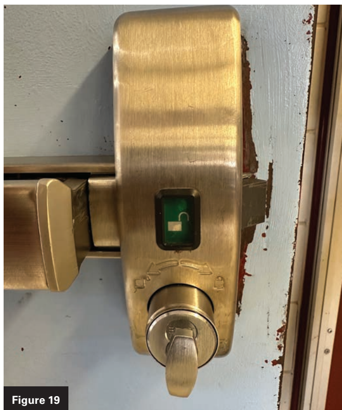
Figures 18 and 19. A PH1 intruder function panic device is shown in the locked and unlocked positions.
