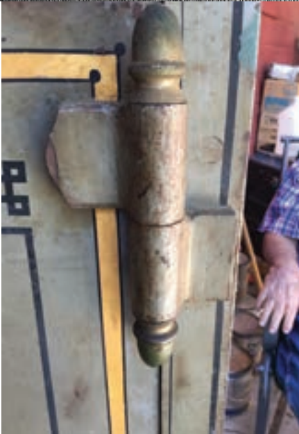
Figure 2. The hinges on this safe are surface mounted.
