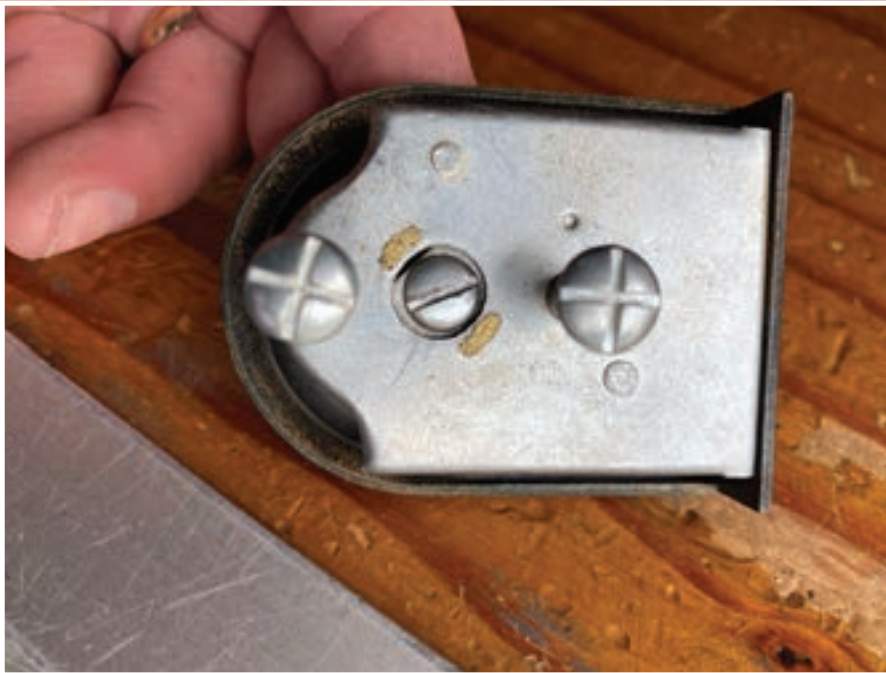
Figure 5. The outer screws mount the lock to the chest, and the center screw holds the key cylinder and dial on.
