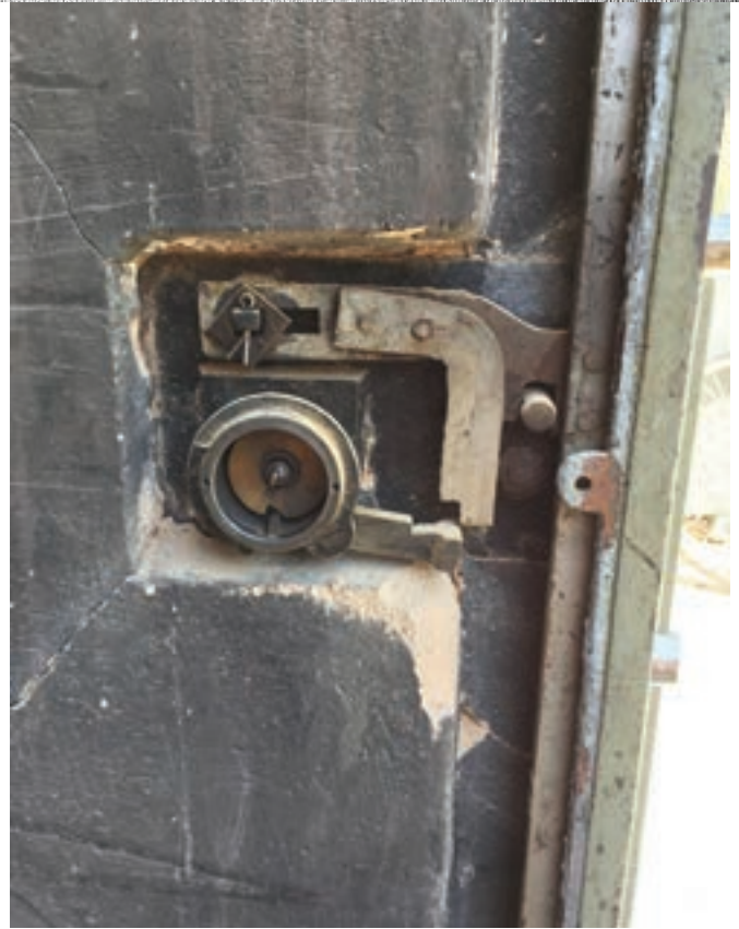
Figure 7. The lock area without the back cover is shown up close. Yale OBs are best drilled where you can look between the gap where the lever enters the lock case.
