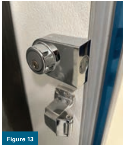
Figures 12 and 13. The red arrow is pointing to the strike for a rim-mounted deadbolt mounted on the frame.
