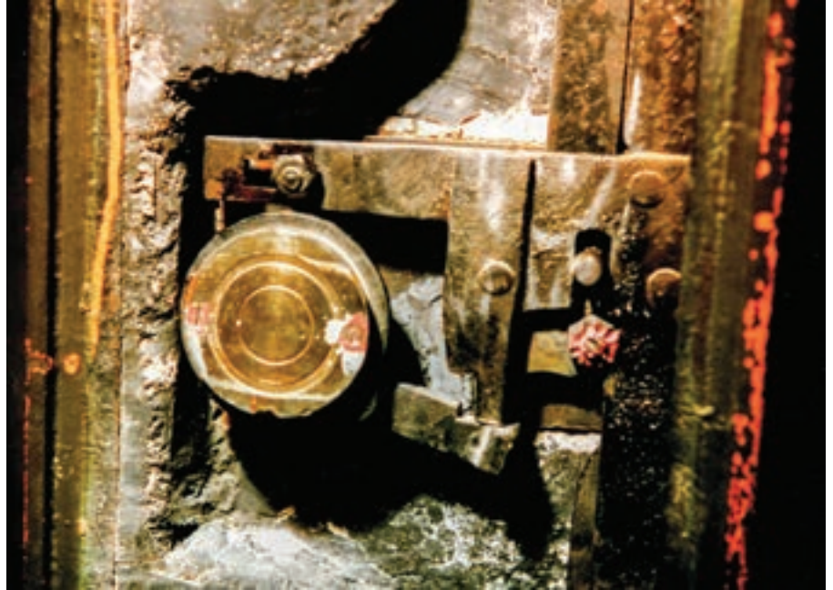
Figure 14. The author patched the holes with some SteelStik putty.
