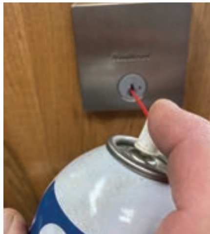
Figure 6. Be sure to lubricate the cylinder before the rekeying process.
