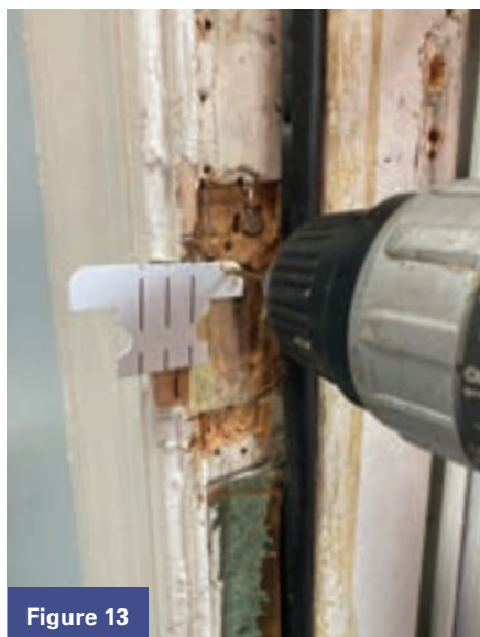
Figures 13 and 14. The author is chiseling out what was needed to make the new strike plate fit properly, and predrilled pilot holes.
