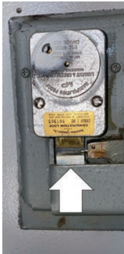
Figure 23. The arrow points to the activated relocker.
