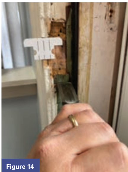
Figures 13 and 14. The author is chiseling out what was needed to make the new strike plate fit properly, and predrilled pilot holes.
