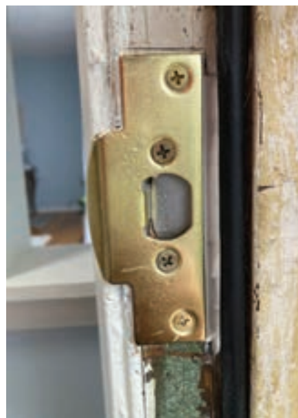
Figure 15. The new strike plate is installed.
