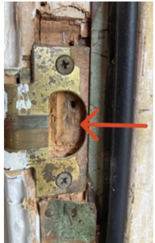
Figure 5. There is barely any of the wood cut out for the latch to drop into.
