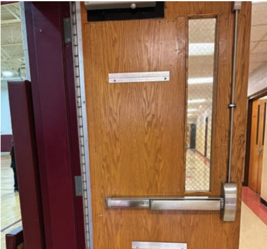
Figure 5. This image shows a vertical rod panic device on a single door.
