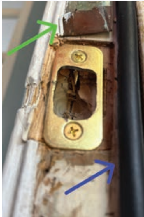
Figure 3. The spring bronze weatherstripping (green arrow) and the self-adhesive weatherstripping seal (blue arrow) on the doorframe were causing a bind on the door.
