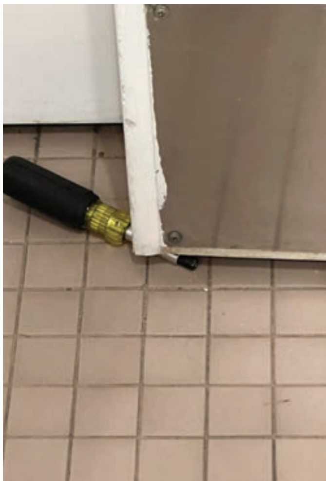
Figure 12. The author wedged a screwdriver under the door to help get the hinge back in position.
