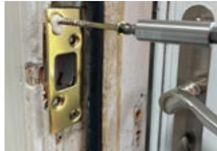
Figure 24. The new strike plate is being attached.
