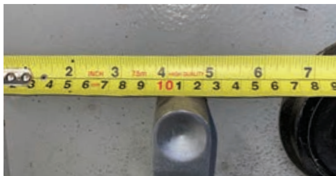
Figure 6. Our research showed that when the distance from the edge of door to handle center is less than 6", the lock is usually RH. Not this time.
