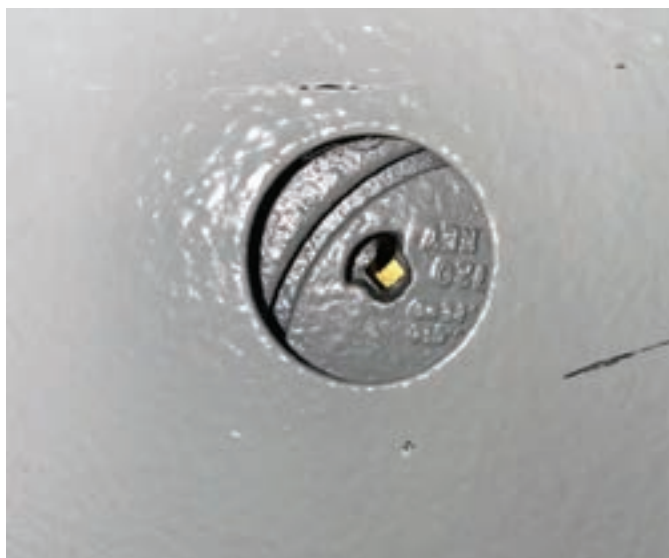
Figure 18. There is an extra-large hole in the door pan for the change key.
