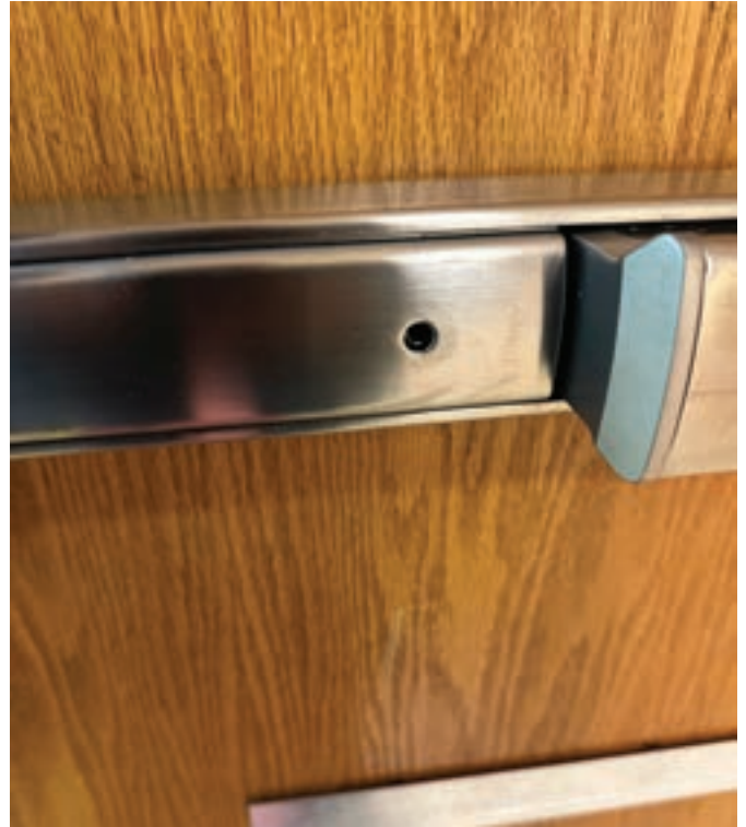
Figure 4. See the hole for the dogging key, also a no-no.
