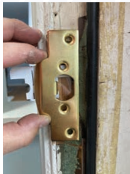
Figure 12. The new strike plate is positioned on the doorframe.
