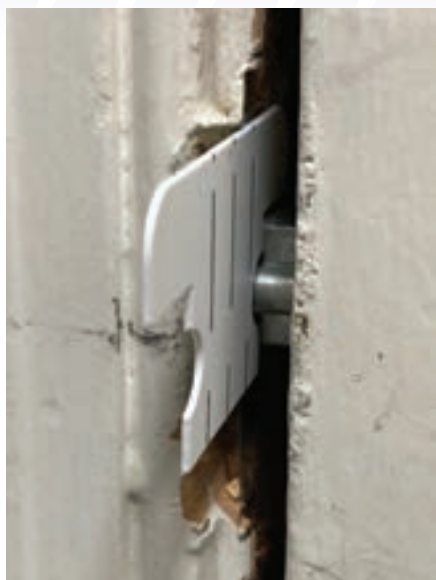
Figure 10. The adhesive side of the location card is facing the doorframe.
