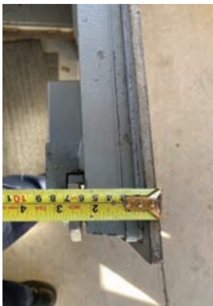
Figure 16. The locking bar depth is shown.
