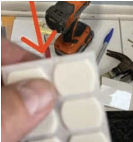
Figure 20. The location tape is double-sided, so once it's installed on the end of the deadbolt, peel off the outer portion to reveal the sticky side.
