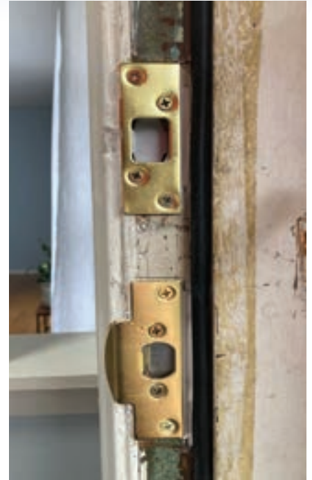
Figure 25. Here's the completed work for both strike plates.
