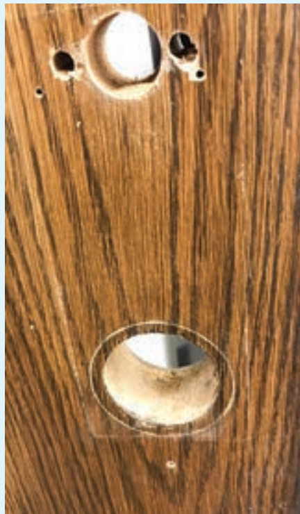
Figure 16. You can see how close the pilot holes were to the existing holes from the previous installation.
