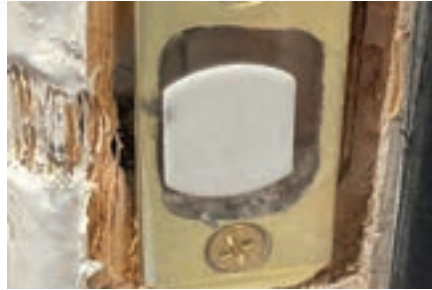
Figure 23. The author used this as a guide for the new strike plate.
