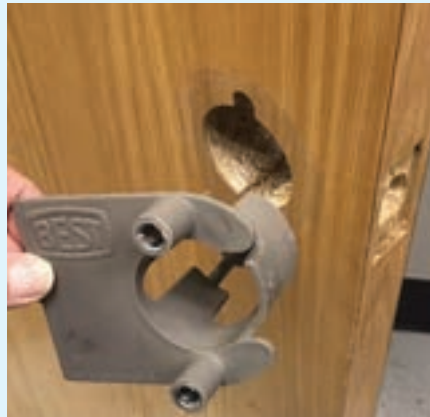
Figure 10. A few lock companies made plastic jigs for making the holes without needing the paper template.
