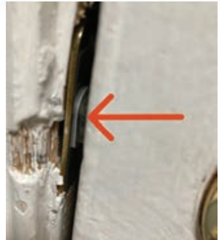
Figure 22. The location tape on the end of the bolt is sticking to the cover tape that's covering the deadbolt strike plate.
