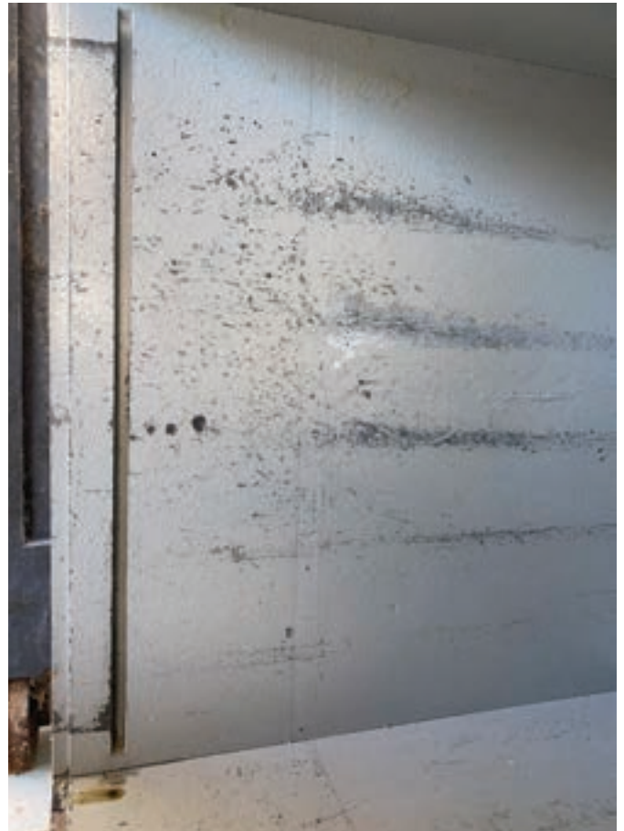
Figure 14. There is a groove on the wall for the locking bar and same on the other side for the hinge fixed bar.
