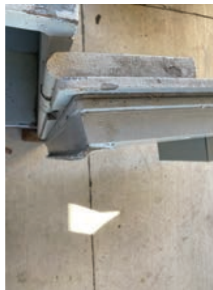
Figure 17. The hinge-side doorframe interlock is visible.
