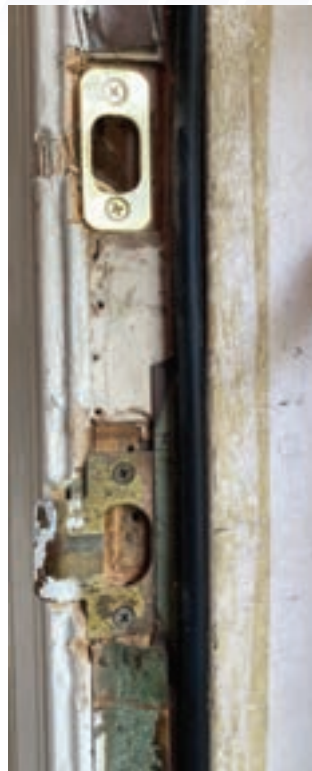
Figure 4. There appeared to be previous work done on the doorframe and strike plates.
