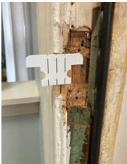
Figure 11. The author could see exactly where the new strike plate should be positioned.
