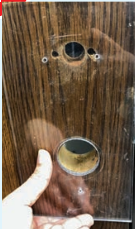
Figure 15. The two top guide holes are very close to holes that existed from the previous Simplex 1000 installation.
