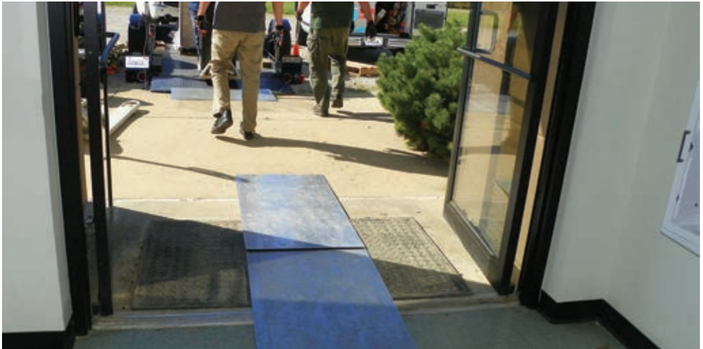
Figure 9. Protect the Threshold – This job was pretty straightforward. Here, the closest sheet protected the threshold from damage as the heavy cabinets were brought through the doors, while the outer sheet smoothed out a small ridge from the concrete sidewalk pad to the entryway.
