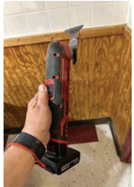
Figure 14. The author used a vibrating tool to make room for the latch pocket in the plate.
