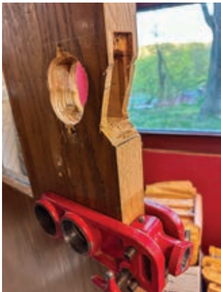
Figure 7. Whoever did the installations used the old deadbolt holes and strike — but the old preps were for mortise deadbolts.
