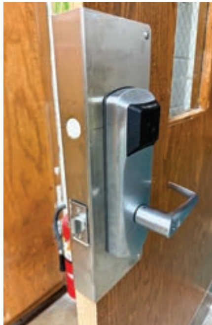
Figure 19. This is another view of the contact and the completed E-Plex installation.
