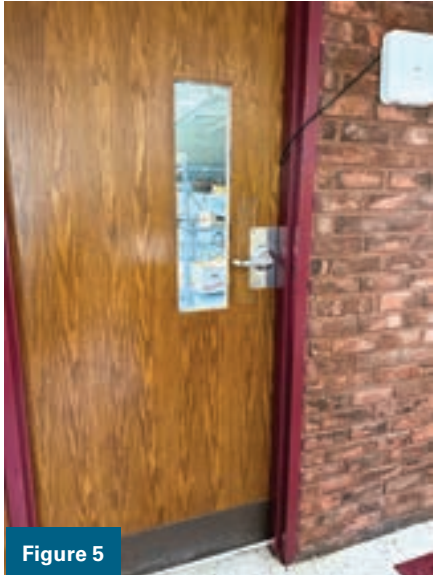
Figures 5 and 6. Notice how high the locks are on these two funky installations.
