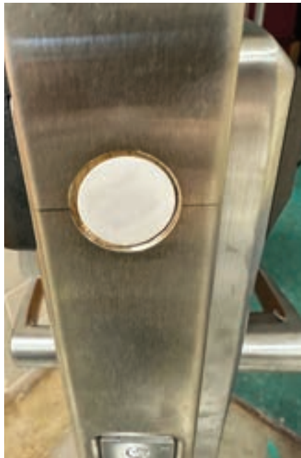
Figure 18. Here's a finished contact installed through the 1" hole in the wrap.
