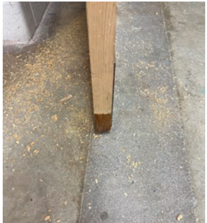
Figure 2. You can see how the very bottom of the door still has a few inches of the original finish.
