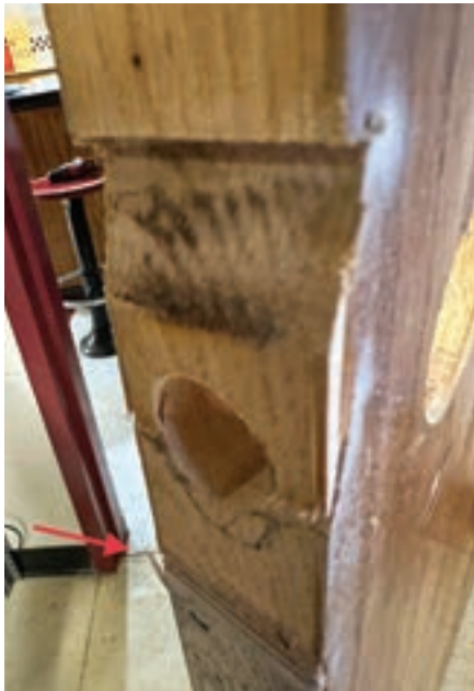
Figure 12. The red arrow points to the bottom of the chiseling the author did for the wraparound to fit.
