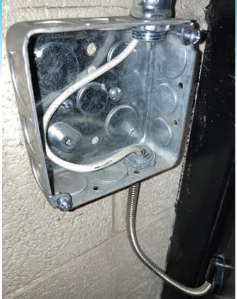
Figure 1. The electrical workbox was just used as a pass-through for the power wire.
