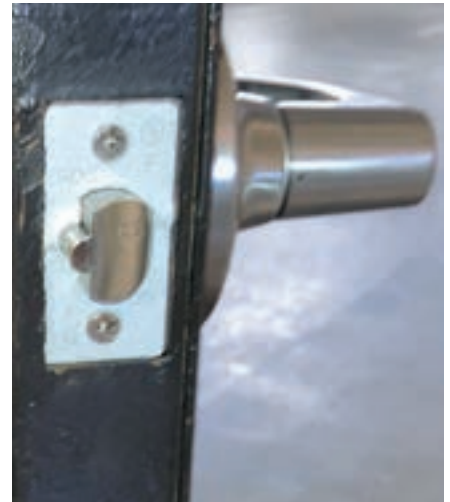
Figure 20. The latch is installed.
