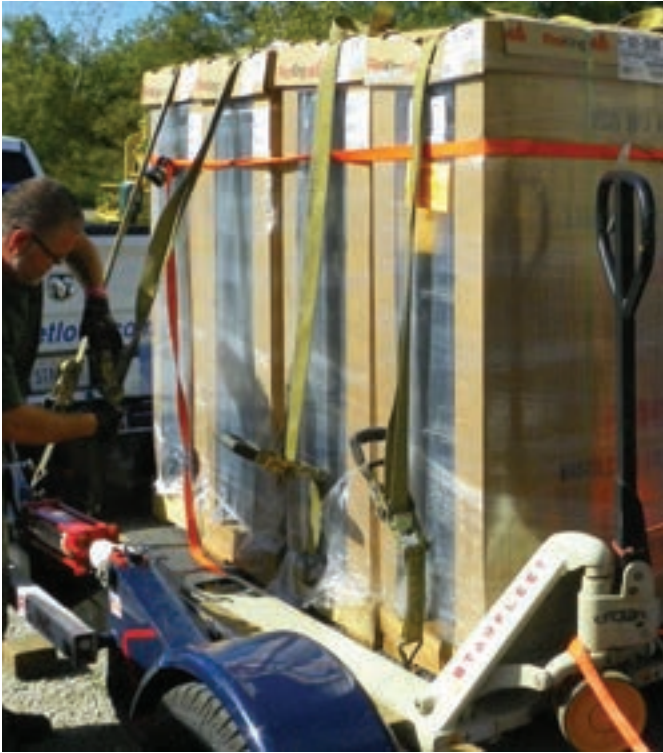
Figure 5. Loosen the Ratchets – Next, the larger tie-down straps were released from one side of the trailer frame rails. Each cabinet has its own primary vertical strap, and a second narrower strap was used to cinch the four units together horizontally.
