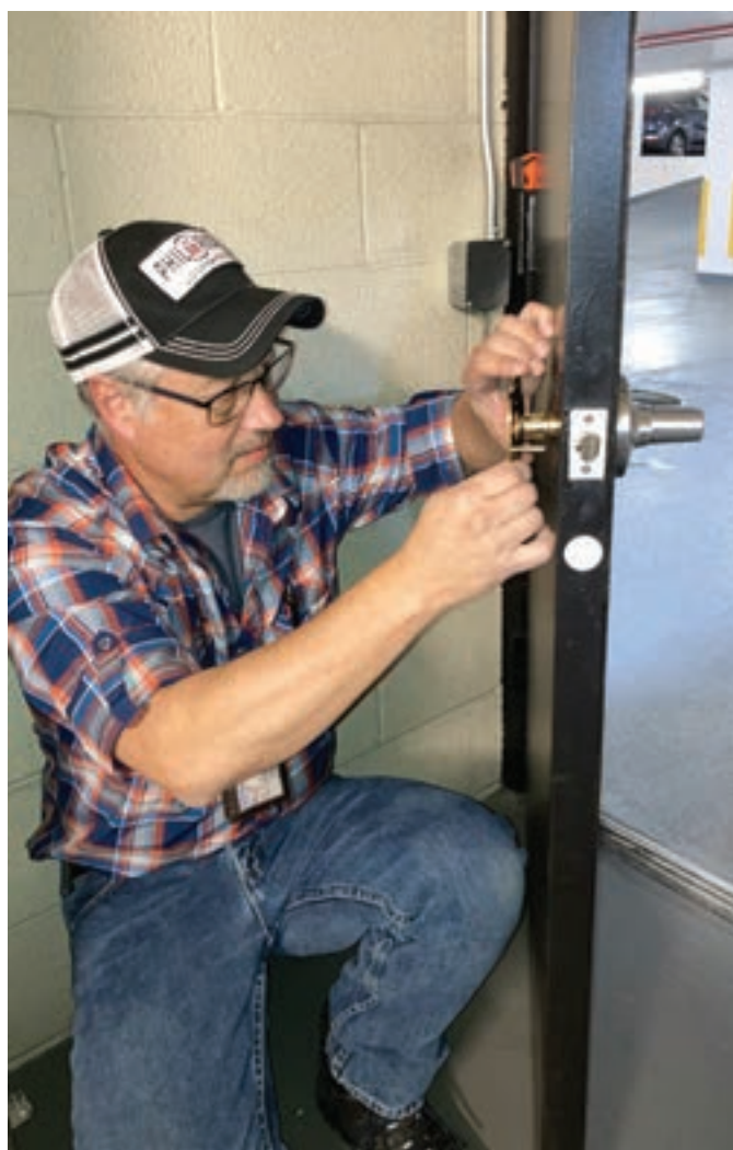
Figure 23. The author is installing the lock.
