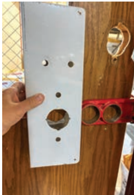
Figure 8. The author is checking to see if the wraparound would cover the top hole.
