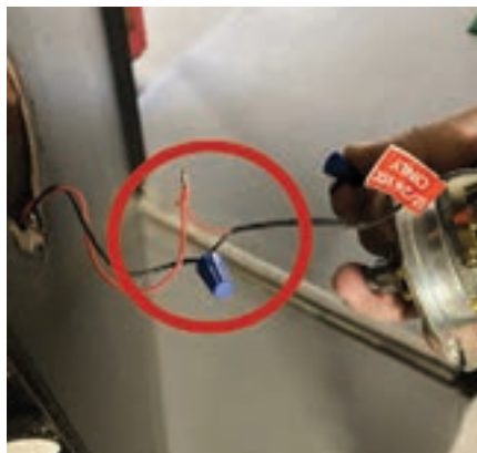
Figure 2. The power wires were attached to the lock with twist-on wire nuts.
