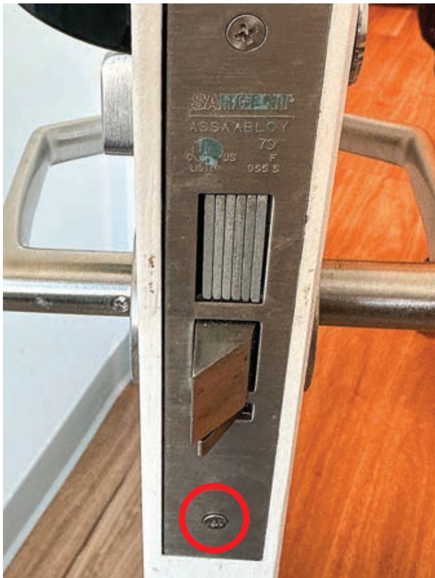
Figure 1. The red circle shows the bottom screw on which someone used impact drivers.
