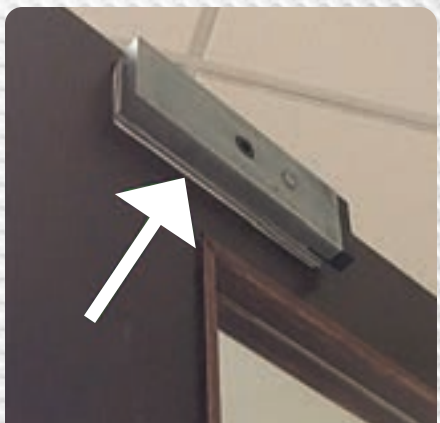
Figure 13. The armature plate was not floating on the door as it should be.
