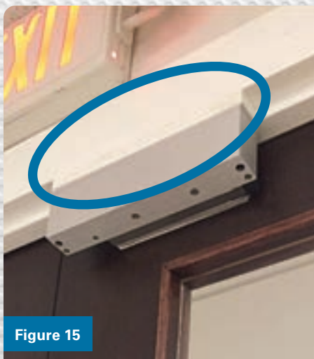
Figure 13. The armature plate was not floating on the door as it should be.
