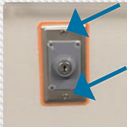
Figure 23. Phillips-head screws were used on the switch plate to fasten it to the low-voltage workbox.
