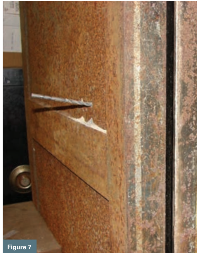
Figure 6. The second hole was a little over 4½" back at the same height.
