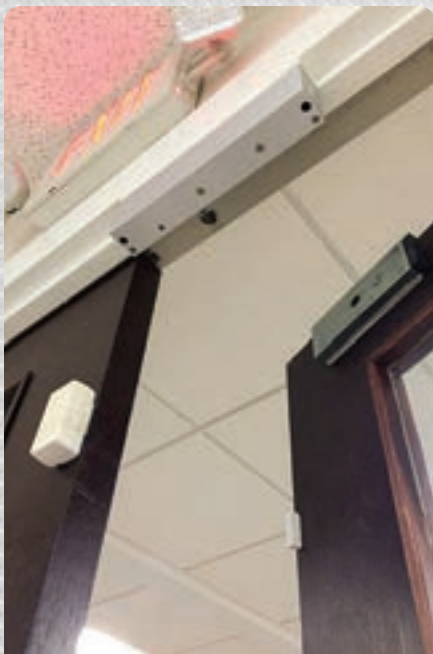
Figure 1. The main entry door had a magnetic lock, and above the lock was an emergency exit sign with emergency lighting.
