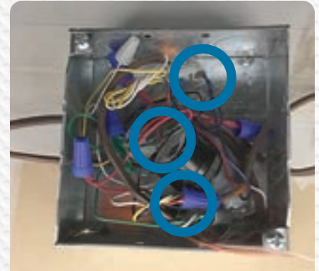
Figure 7. Some of the wires were broken or poorly connected.
