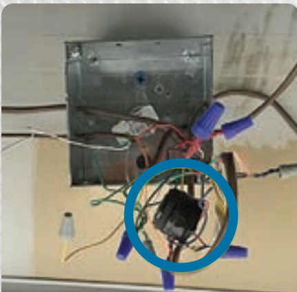
Figure 8. There was a piezo siren inside the workbox.
