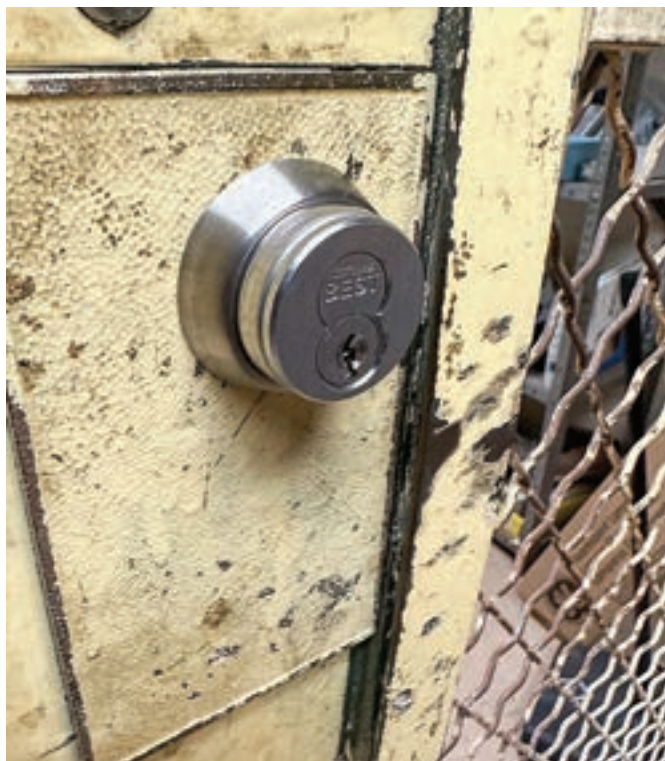
Figure 10. The gate lock is reinstalled.
