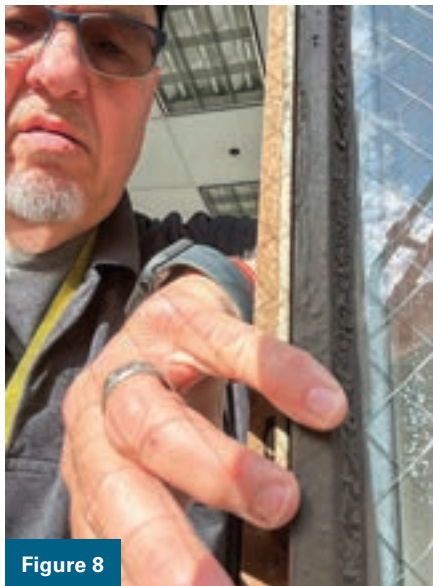
Figures 8 and 9. These two images are a reminder to the author of how he's going to accomplish the job. In Figure 8 , his hand is on the putty holding the glass in.
