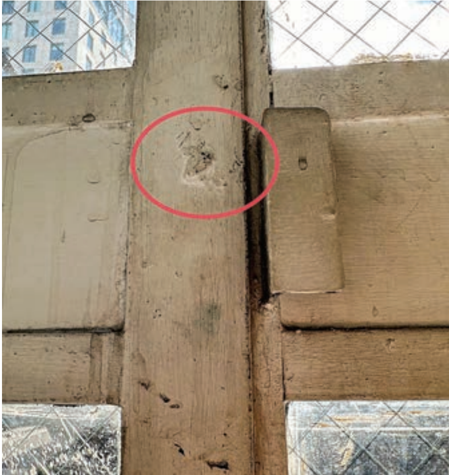
Figure 7. The client wants the author to put a DETEX EAX 500 on this metal casement window that opens onto a fire escape.
