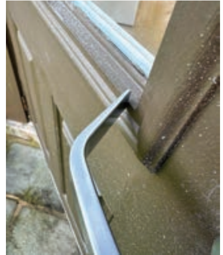
Figure 3. The return on the lever is too long and is not clearing the moulding.
