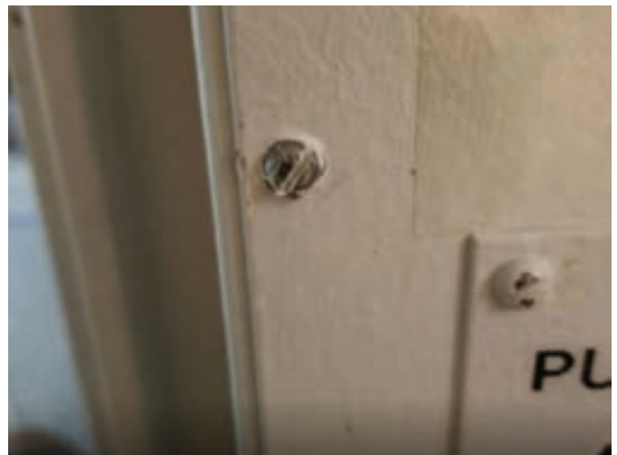
Figure 6. The Screws. Possibly the most annoying part of the job was removing the 30 (count ‘em: 30!) slotted screws from the back plate. These screws were so full of paint that they looked like rivets at first glance. Thankfully, while the door exterior was recently painted, the inside was not. Undisturbed for who knows how many decades, it was a real chore. Oddly enough, they all “got lost” during the repair and had to be replaced with Phillips self-drillers that went in quite nicely with the cordless drill.
