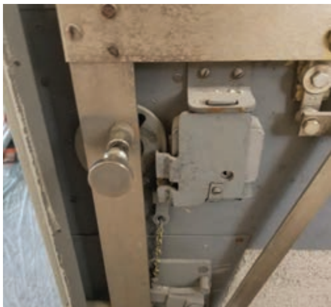
Figure 10. Inside Release. The emergency inside release handle is seen here. Pulling the knob toward you disconnects the bolt carrier bar from the handle cam. Then applying some effort and sliding the knob to the right moves the boltwork back, allowing egress.
