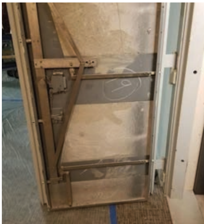
Figure 12. The End. With all the hard work finished, it was time to wrap this job up. Since I did a complete service to this door, I'd repaired, adjusted and lubricated virtually every moving part in this door as well as the lock itself. I then reassembled the door cover (with those shiny new screws) and invoiced the customer.
