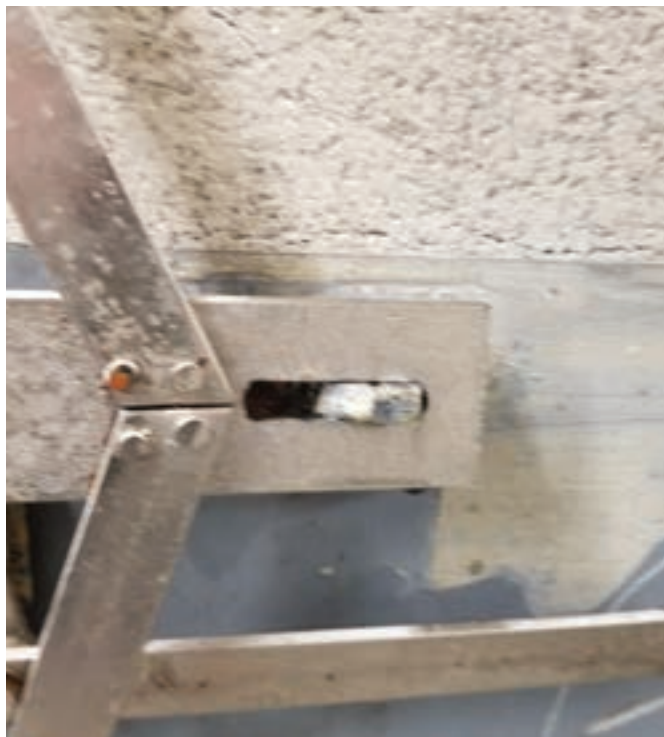
Figure 11. The Guide. Here is the center tab that guides the boltwork back.
