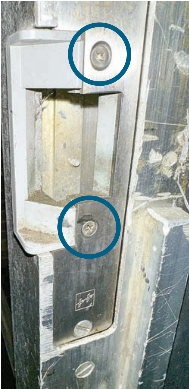
Figure 9. The keeper is missing on this strike.
