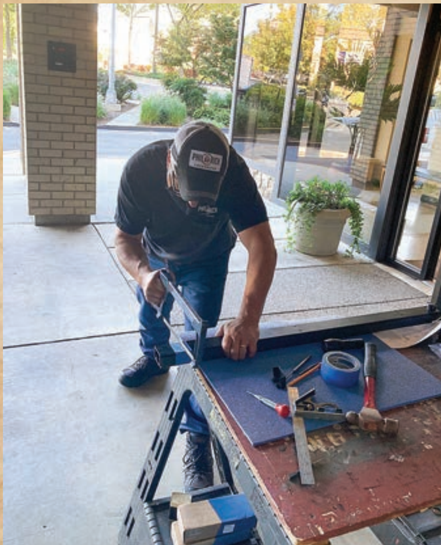
FIGURE 3. Hacksaws are the author's go-to when there is only one exit device to cut.
