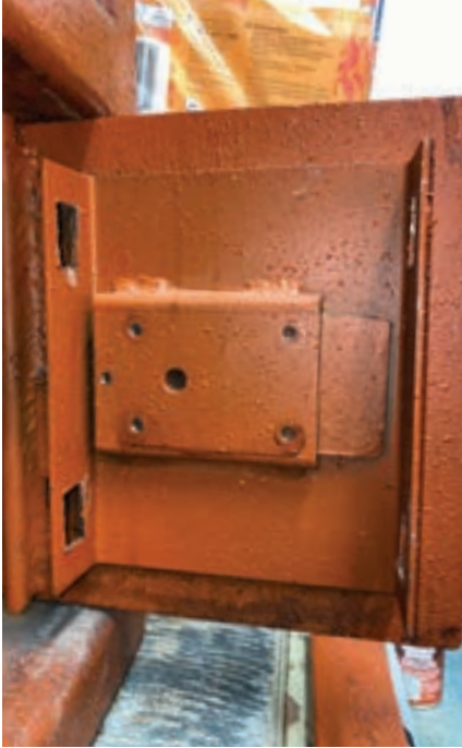
FIGURE 12. The lock is removed from the door.
