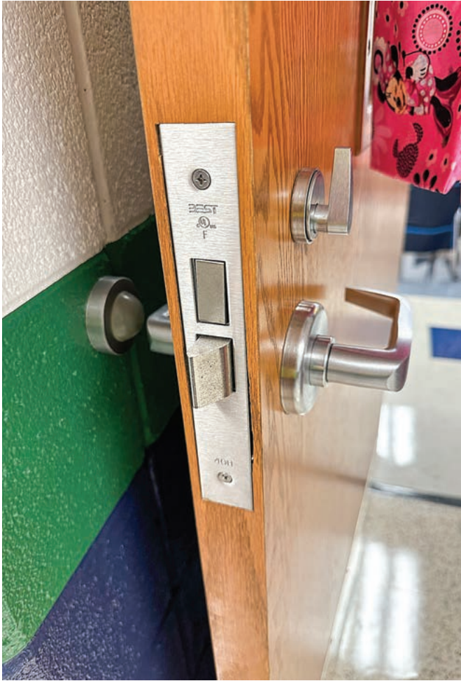
FIGURE 10. This classroom door has a mortise lock with a deadbolt.
