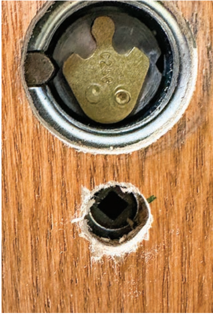
FIGURE 15. The lock is reassembled minus the mortise thumb turn.
