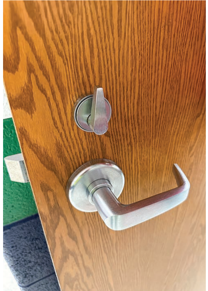
FIGURE 11. The mortise thumb turn on the inside of the door throws and retracts the bolt.
