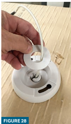
FIGURES 27-29. You can see the sequence of securing the antenna with the plastic washer and nut.
