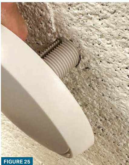
FIGURES 25 AND 26. The author is fitting the antenna through the hole.
