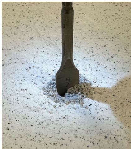
FIGURE 23. The author is drilling a \frac{7}{8} " hole through the tile with a spade bit.
