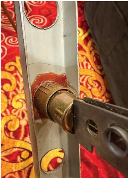
FIGURE 7. The drive-in deadbolt is held in place by epoxy.
