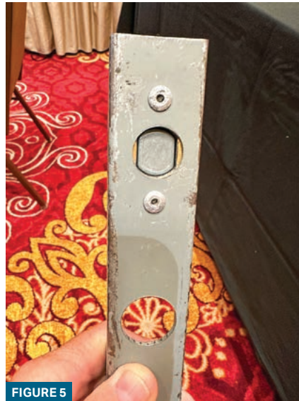
FIGURES 5 AND 6. The deadbolt is inside the door and held on with rivets.
