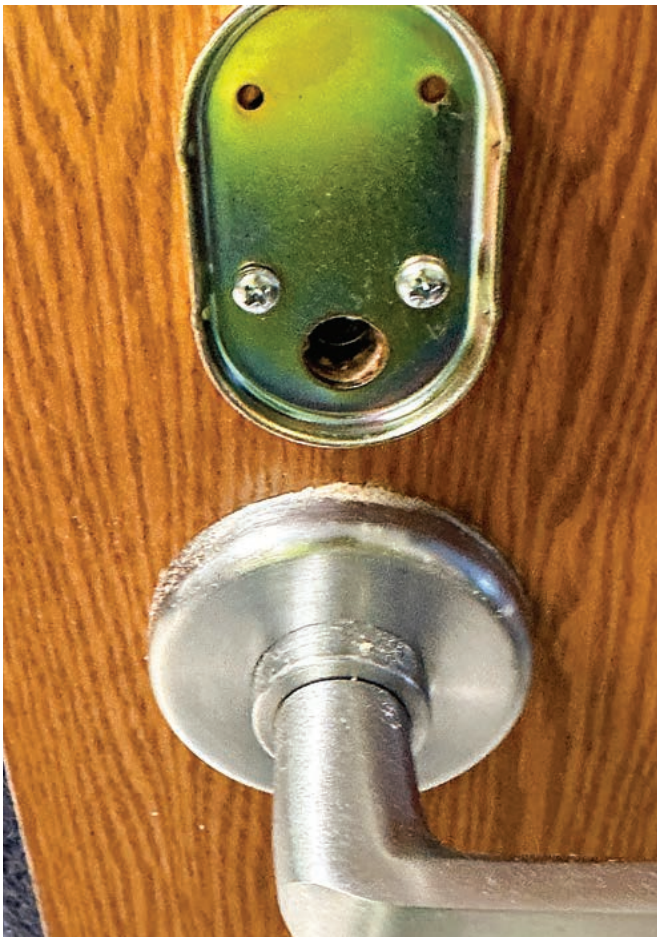
FIGURE 18. The back plate has the two bottom screws installed.
