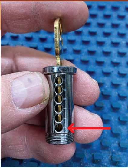
FIGURE 22. The key blank does not extend far enough into the plug to reach the sixth chamber.
