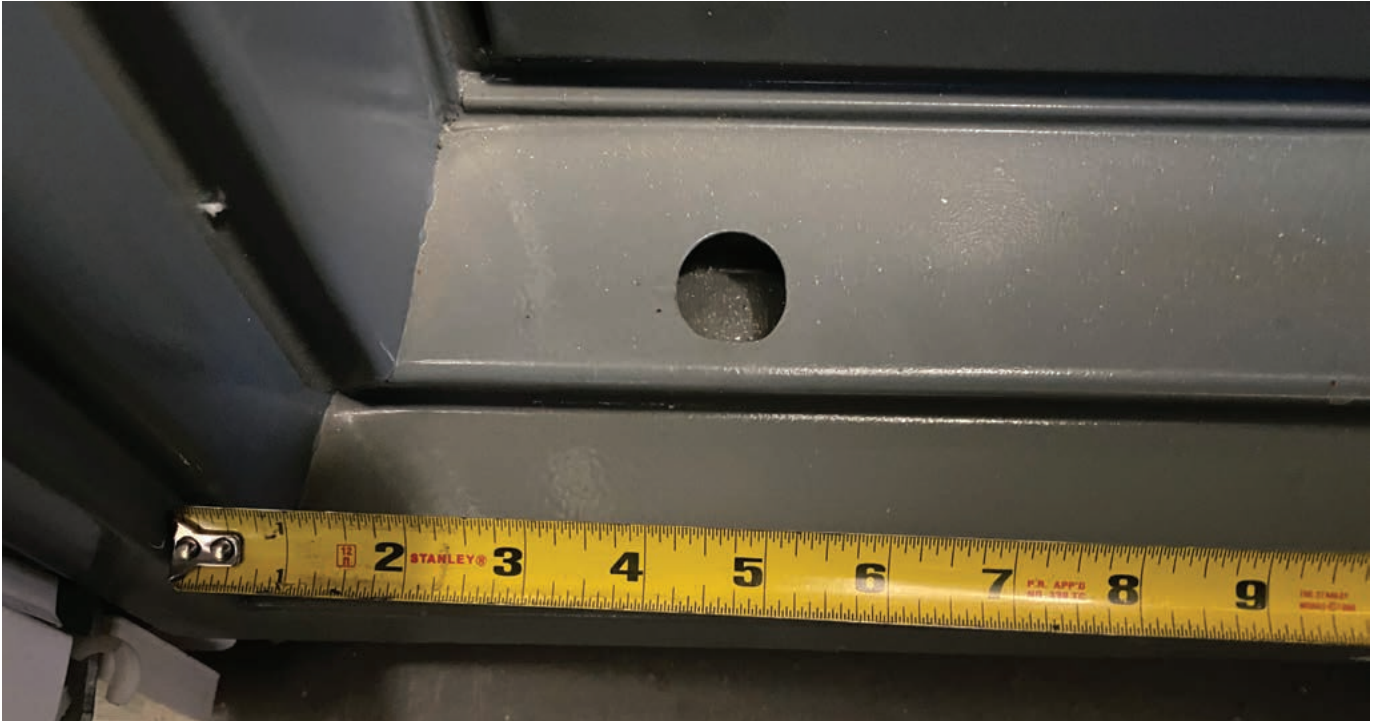
FIGURE 5. The bottom door bolt is 4\frac{1}{2} " from the opening edge lock.
