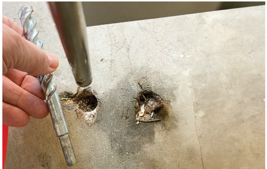
FIGURE 25. Here is the debris in the hole and the masonry drill bit the author used.
