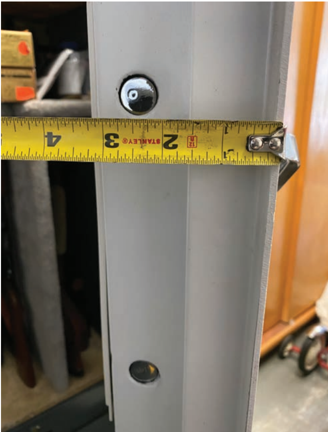
FIGURE 6. All door bolts are 2\frac{3}{8} " deep.
