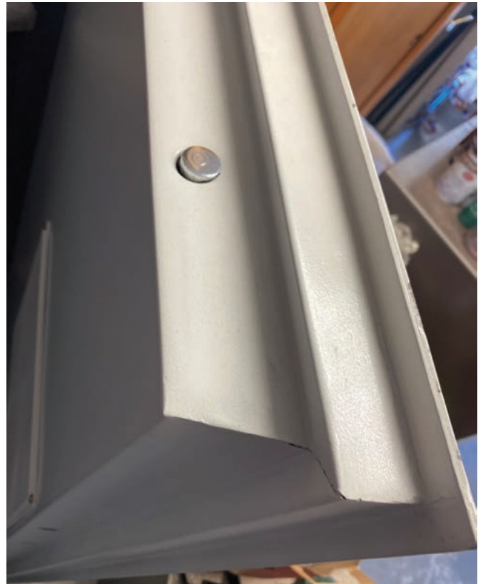
FIGURE 4. The top door bolt is 7" from the opening edge.
