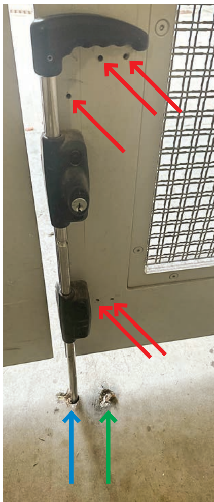
FIGURE 7. You can see the previous mounting holes (red arrows).
