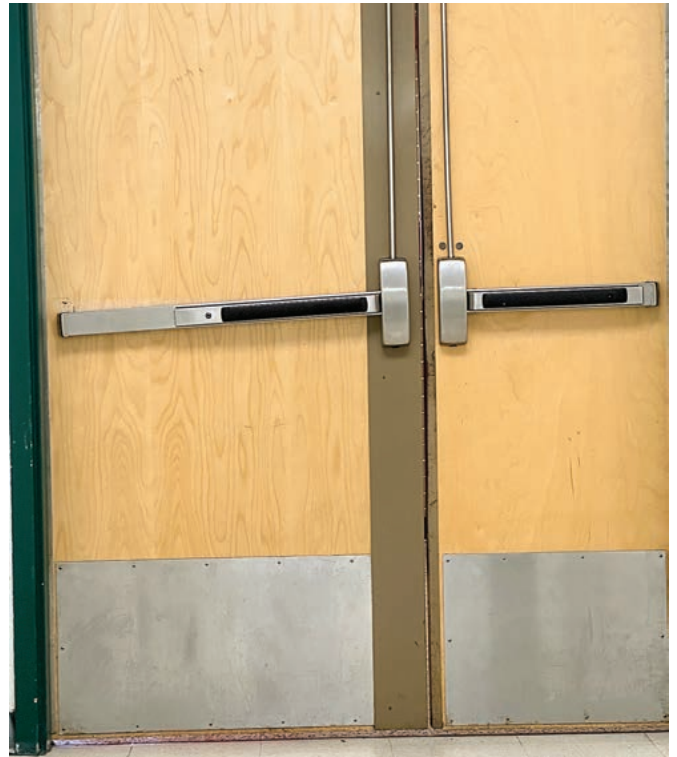
FIGURE 13. The top screw hole, which you can see above the foot of the bar, was stripped.
