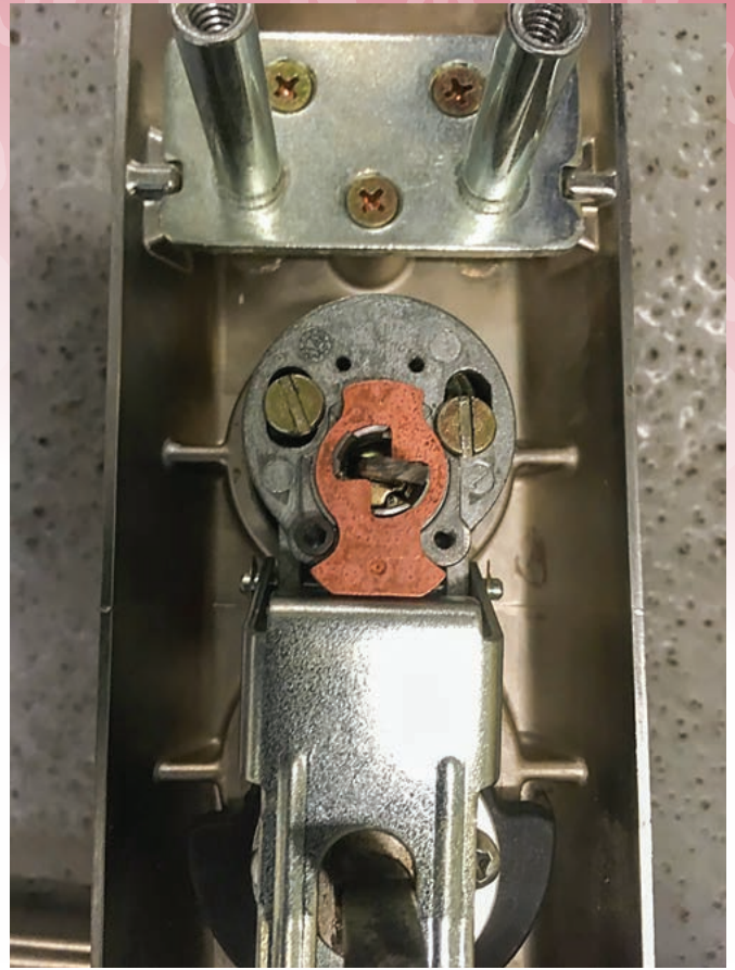
FIGURE 34. The replacement cylinder housing assembly is installed.
