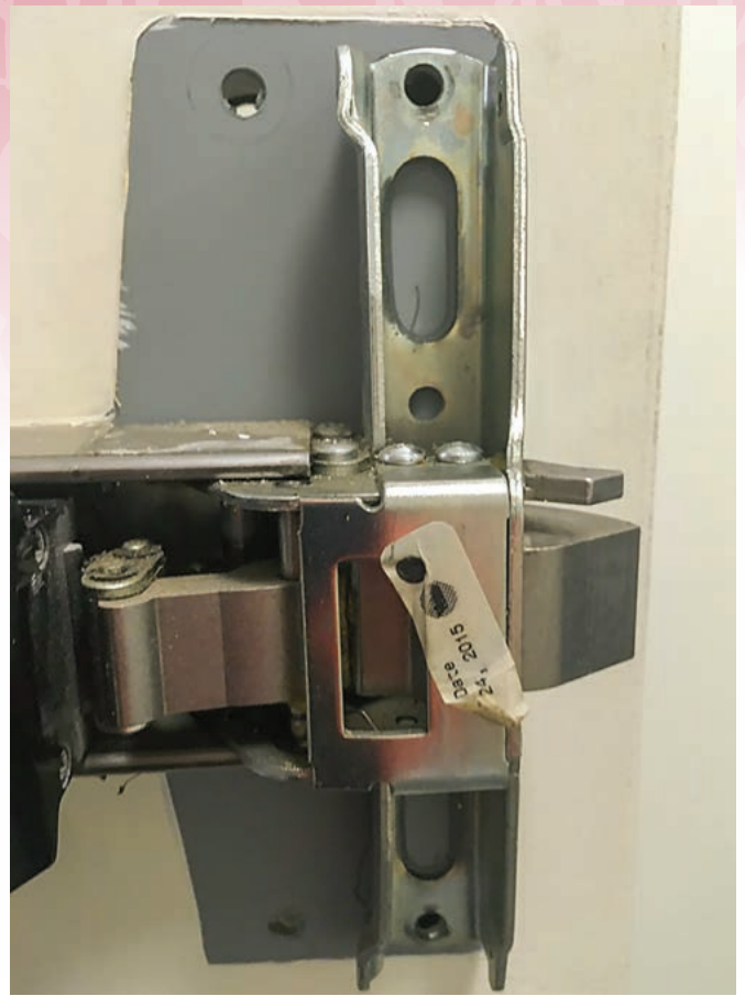
FIGURE 25. The four screws holding the trim to the door have been removed.
