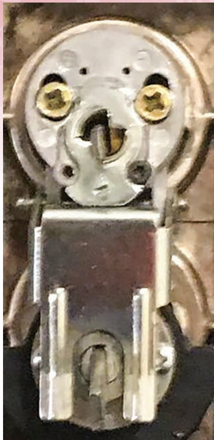
FIGURE 9. The cam assembly is installed.
