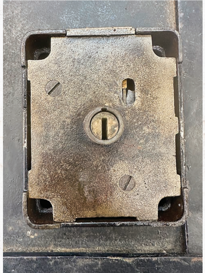
FIGURE 21. The bolt is fully retracted.
