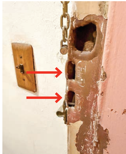
FIGURE 15. The two red arrows point to two rectangular holes on the door frame.
