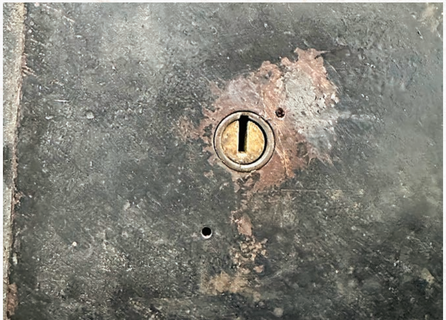
FIGURE 29. The drilled hole is plugged.
