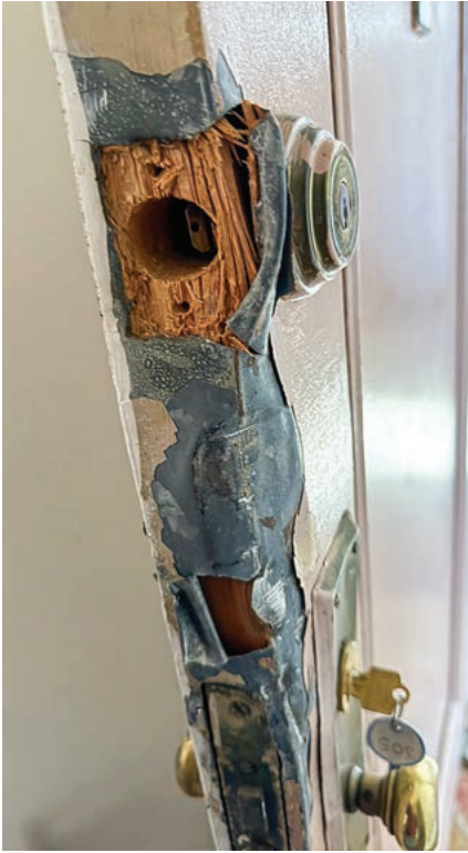
FIGURE 8. This is the most-damaged door (305). You can see how the wood is exposed.
