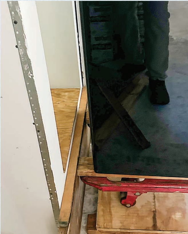
FIGURE 1. The platform is made. The pallet jack and safe will do the lifting to level with the opening.
