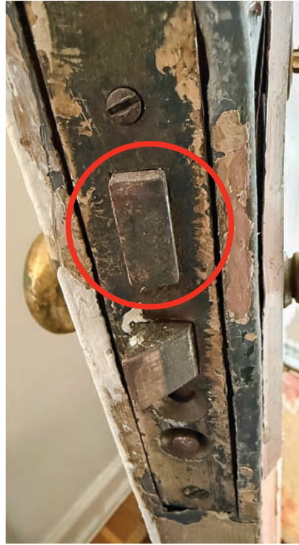
FIGURE 9. The deadbolt of the Chesler mortise lock is circled in red.
