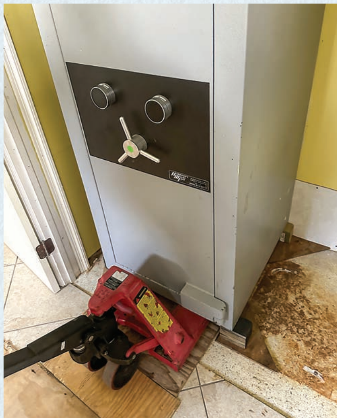
FIGURE 12. The beast is up on 4x4s, and the team was able to pull it out with the pallet jack.
