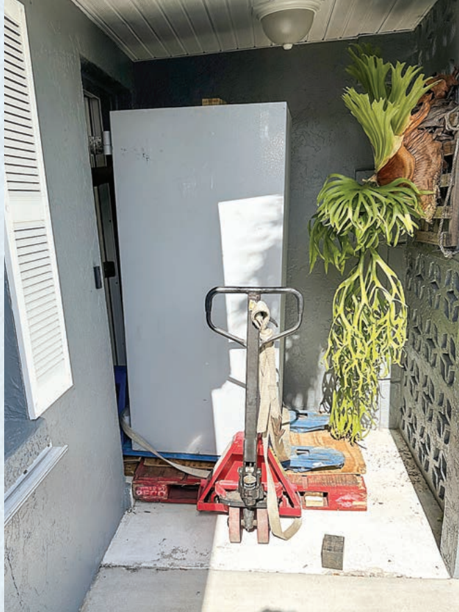
FIGURE 15. This is the front door. You can see the pallet that was used to fill in the front entryway. Two pallet jacks were used to make this tight right turn.
