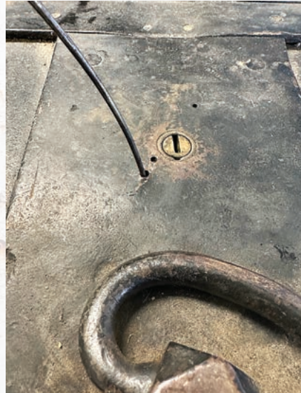
FIGURE 11. The wire is being fished through the lever gates.
