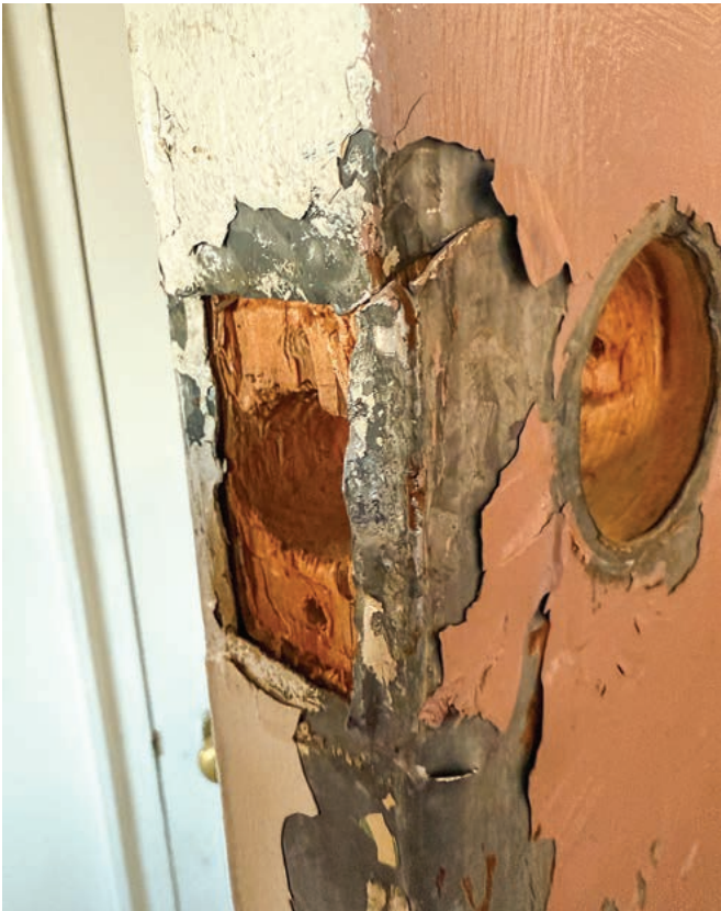
FIGURE 12. The author bent the metal around close to where it used to be by the bolt hole.
