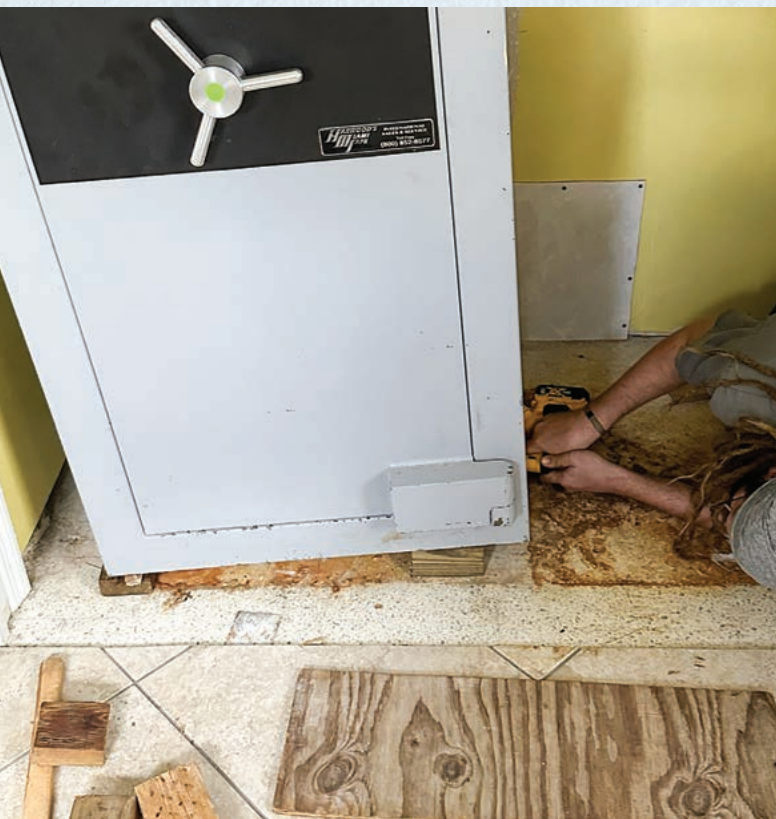
FIGURE 11. The safe is high enough to get Sawzall underneath, with a long blade to cut the bolt.
