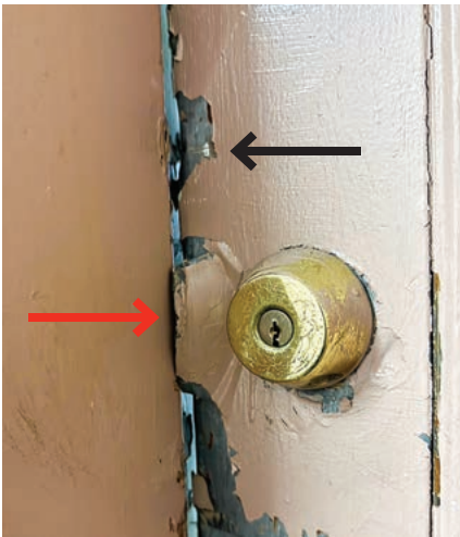
FIGURE 14. The black arrow points to the gain of purchase above the lock, and the red arrow points to the pry marks on the lock.
