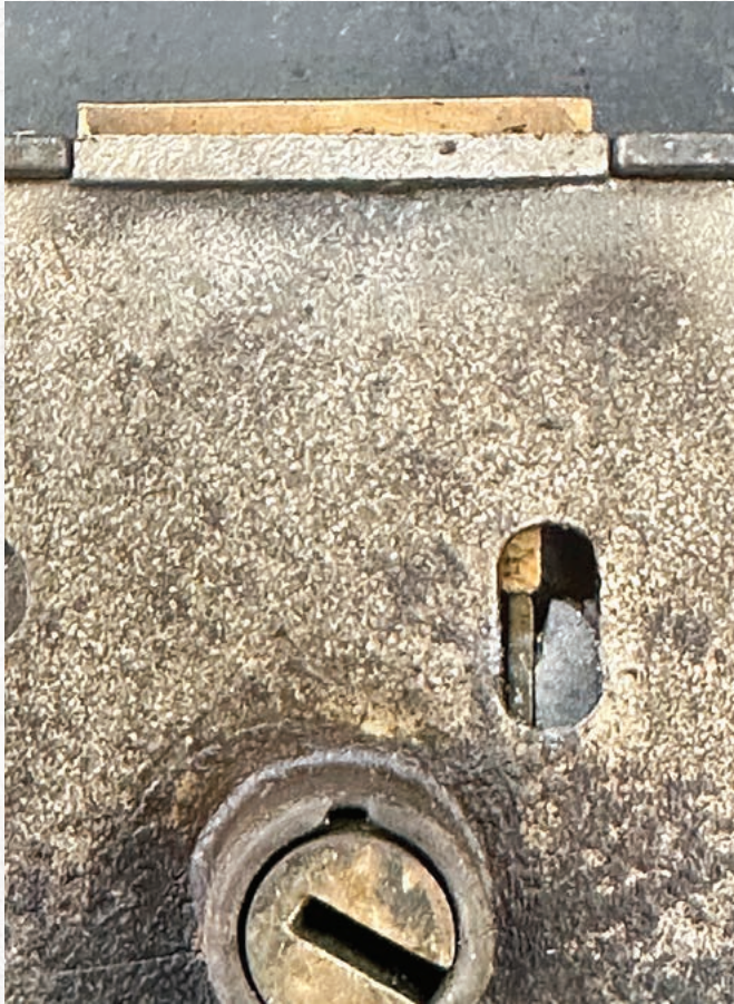
FIGURE 20. The lock bolt is partially retracted.
