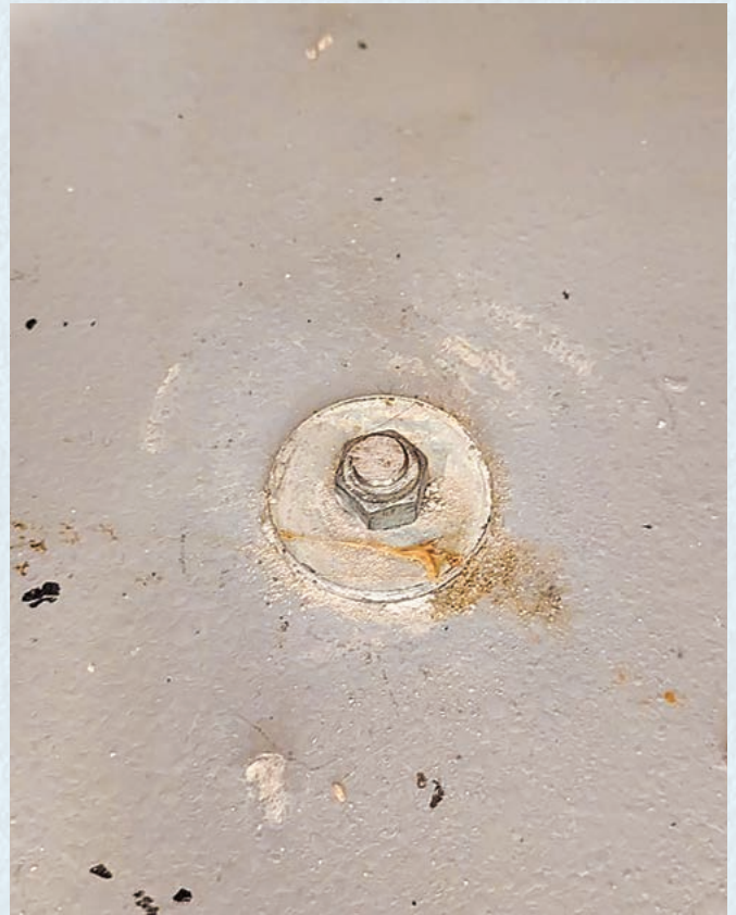
FIGURE 8. This is the bolt down — the expandable bolt anchor.
