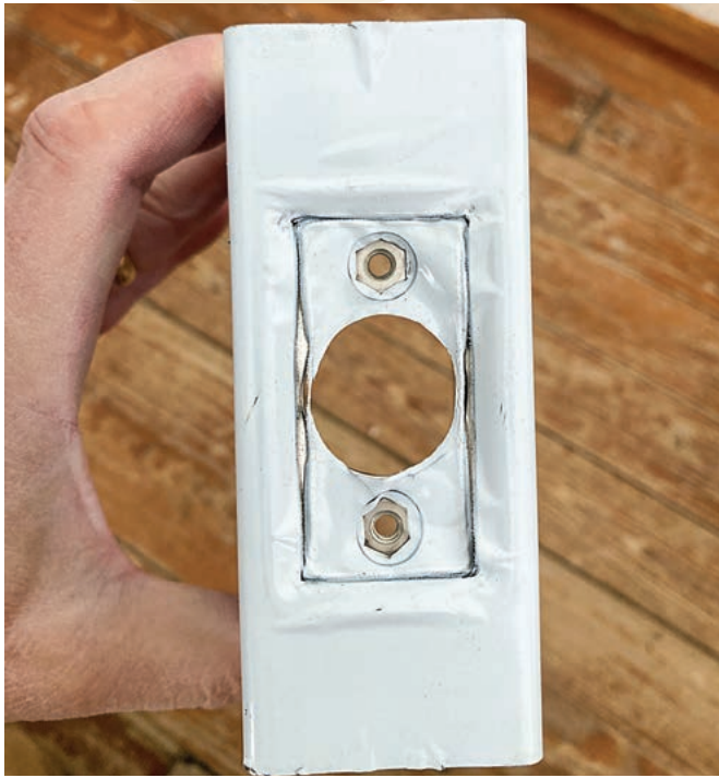
FIGURE 13. The wrap has an indent in the latch prep.
