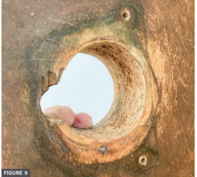
FIGURES 7-9. These images show what was under the wrap reinforcement.
