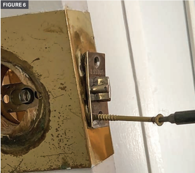
FIGURES 5 AND 6. There were two different types of screws used to install the wrap reinforcement.
