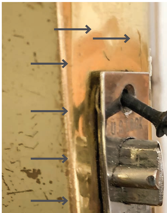
FIGURE 4. You can see the hammer marks from the unsuccessful attempt to make a recess.
