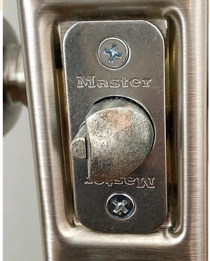
FIGURE 18. The screws securely fastened the latch to the wrap.
