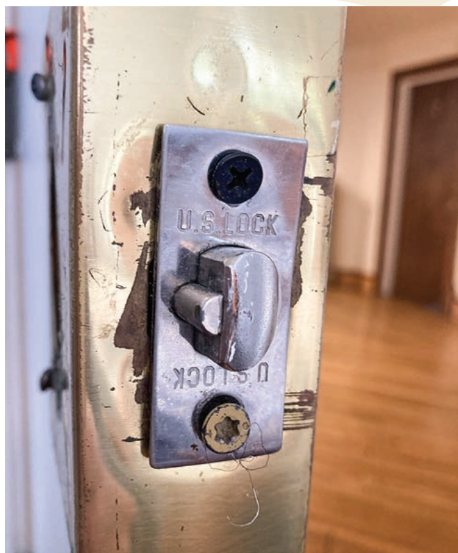
FIGURE 3. The existing wrap had a flat front that did not provide a recess for the latch to sit in.
