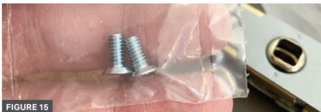
FIGURES 14 AND 15. The indent in the latch prep accepted machine screws that came with the wrap.
